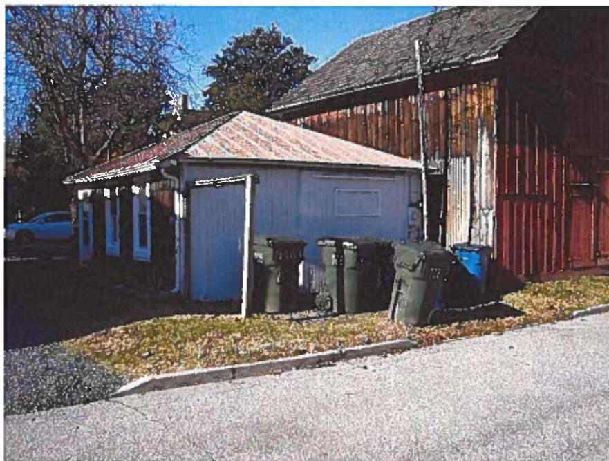
Alley view of the North outbuilding
