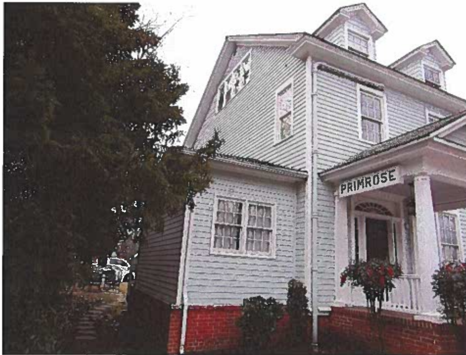
PHOTOGRAPH 3 North elevation of the main building.
