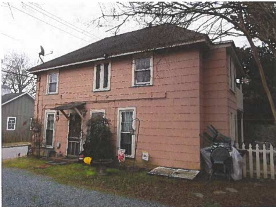
PHOTOGRAPH 14 North elevation of the two-story out-building.
