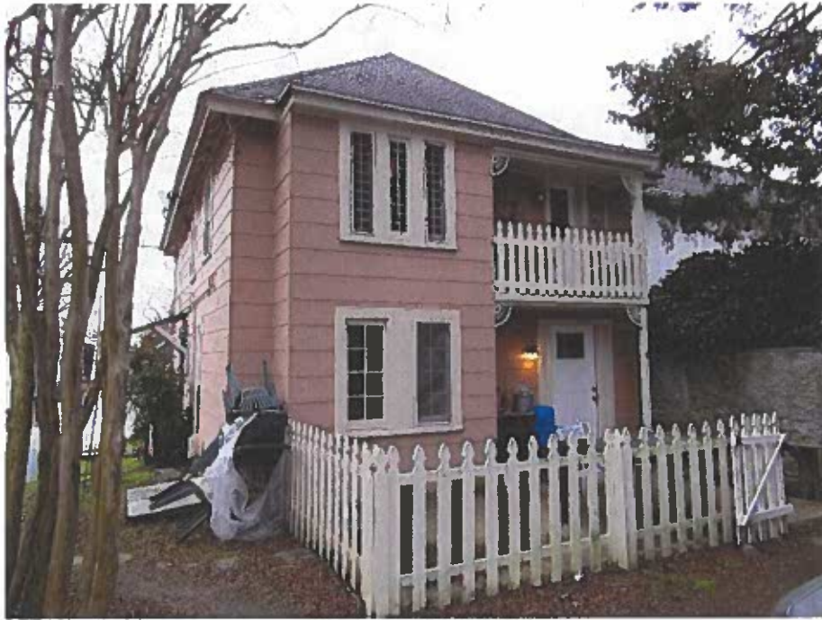
PHOTOGRAPH 13 West elevation (front) of the two-story out-building.
