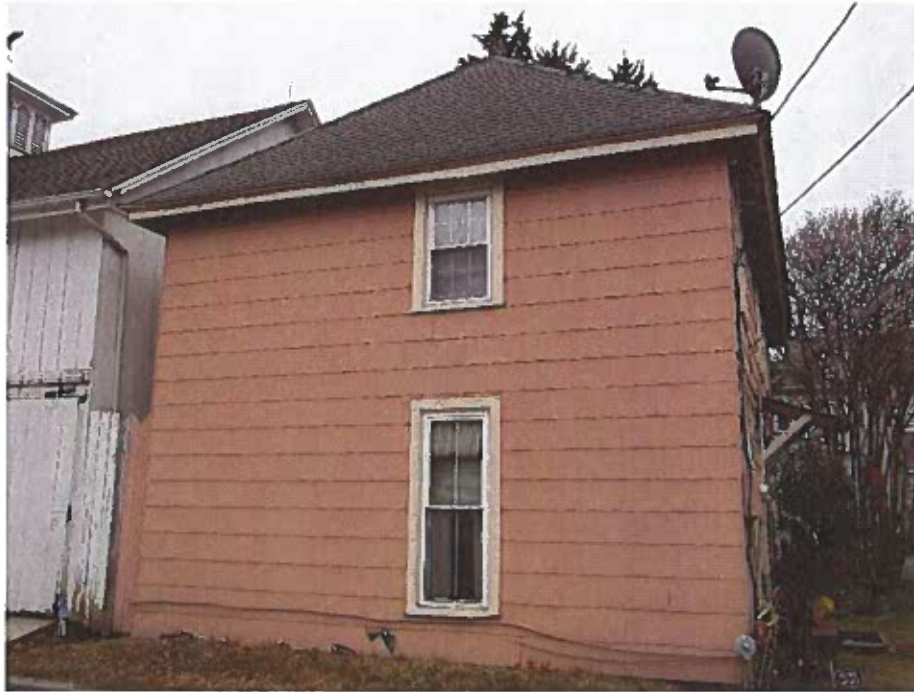
PHOTOGRAPH 15 East elevation of the two-story out-building.
