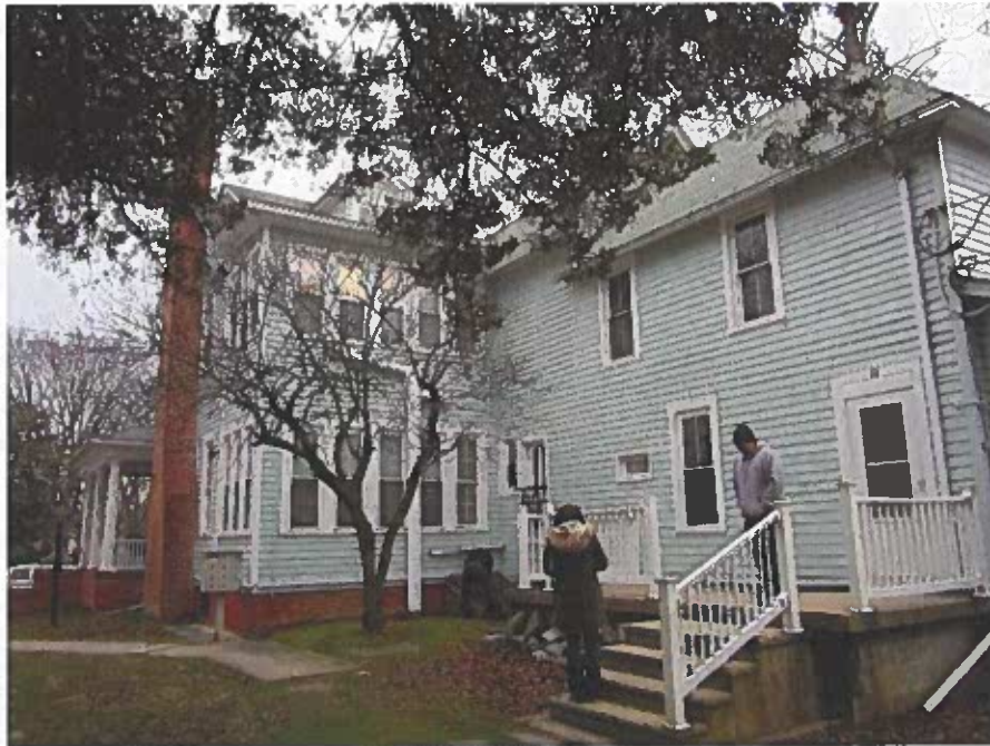
PHOTOGRAPH 5 South elevation of the main building.
