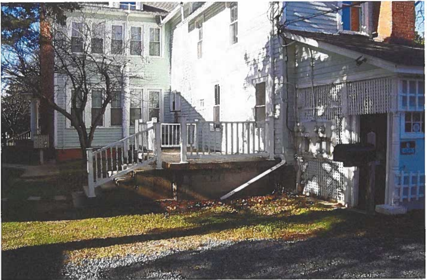
Southeast view of the main structure
