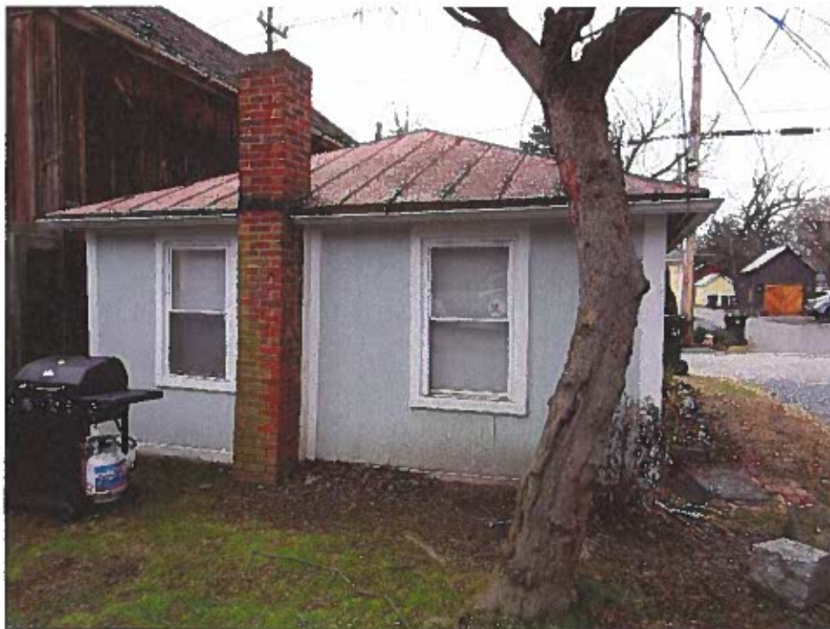
PHOTOGRAPH 20 West elevation of the one-story out-building.
