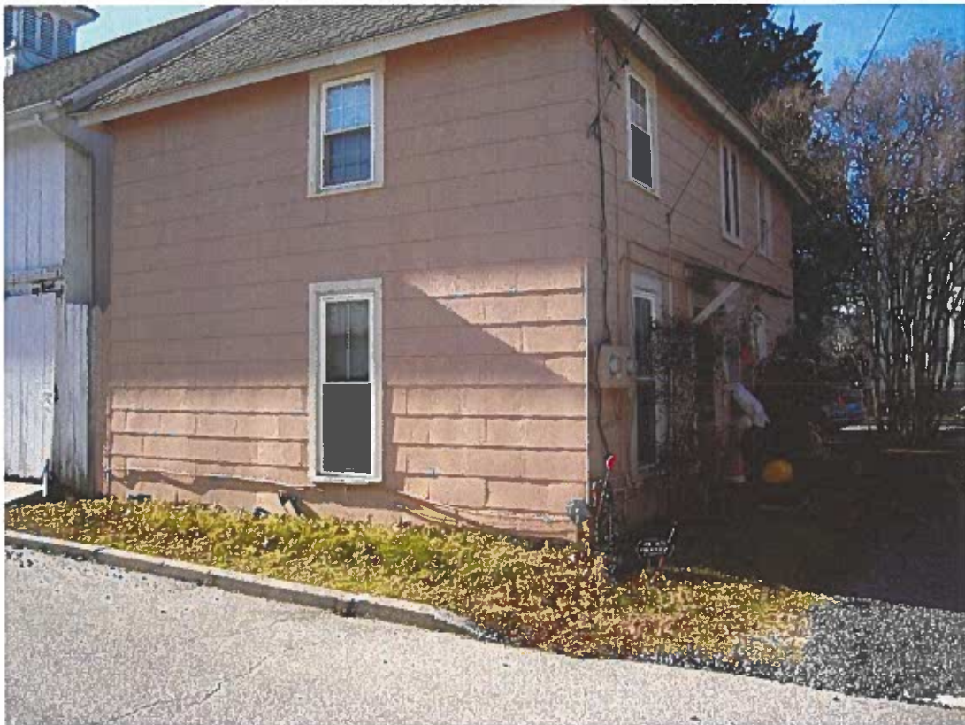
Alley view of the South outbuilding
