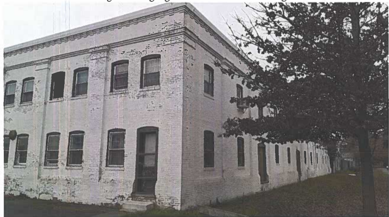
Easton Wholesale Building. To be highlighted as the main Contributing structure at Dover Station.
