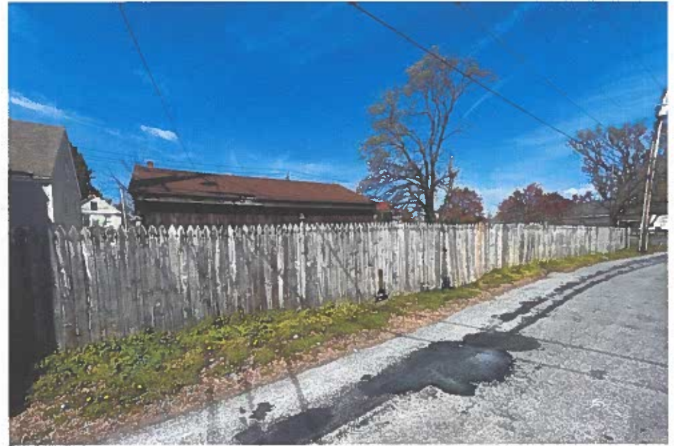
Existing Fence – Scott's Alley (Rear)
