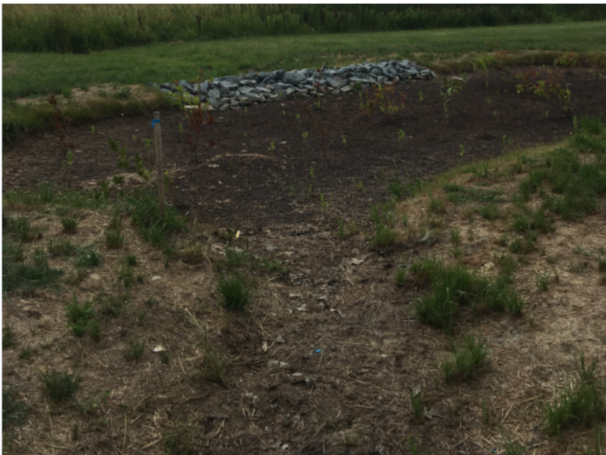
Photo Taken 7/11/17 – Rain Garden #2
