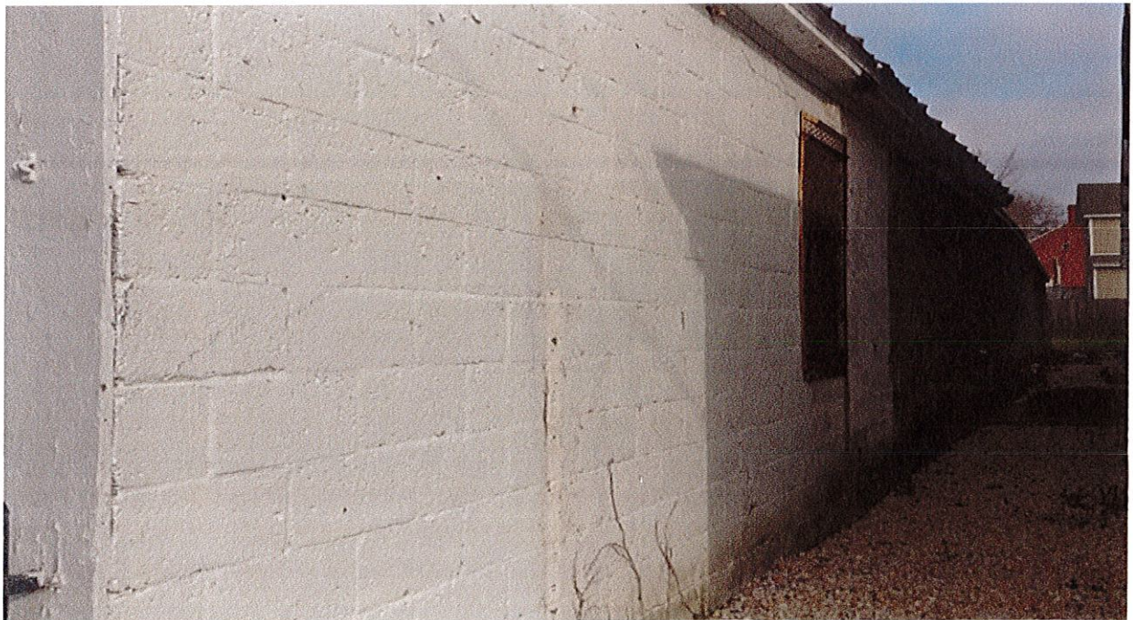
Southern Façade Looking East
