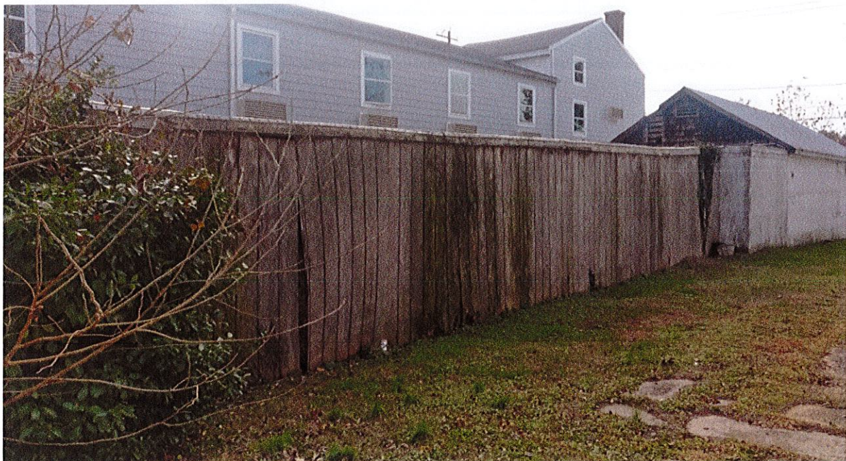
Northern Façade Looking West
