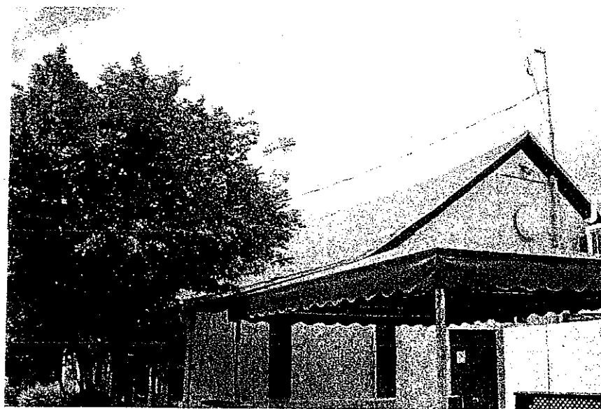
3 - Side Elevation Showing Roof Sag
