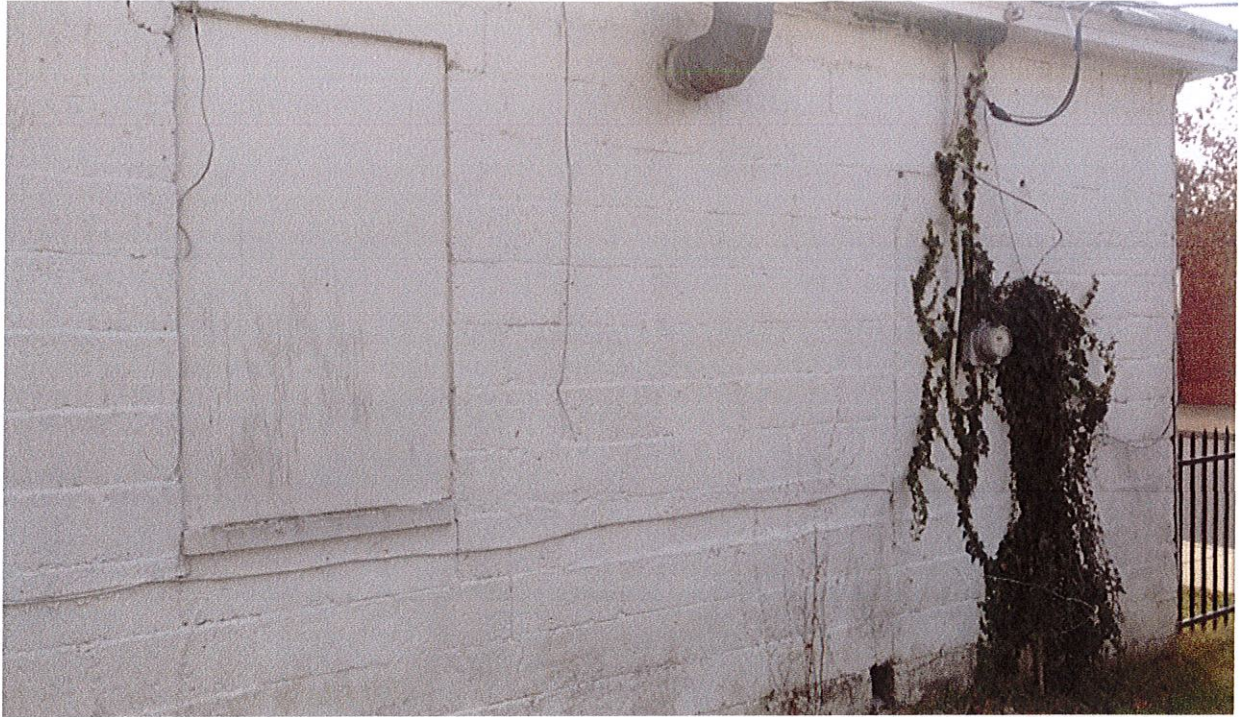
Northern Window Opening
