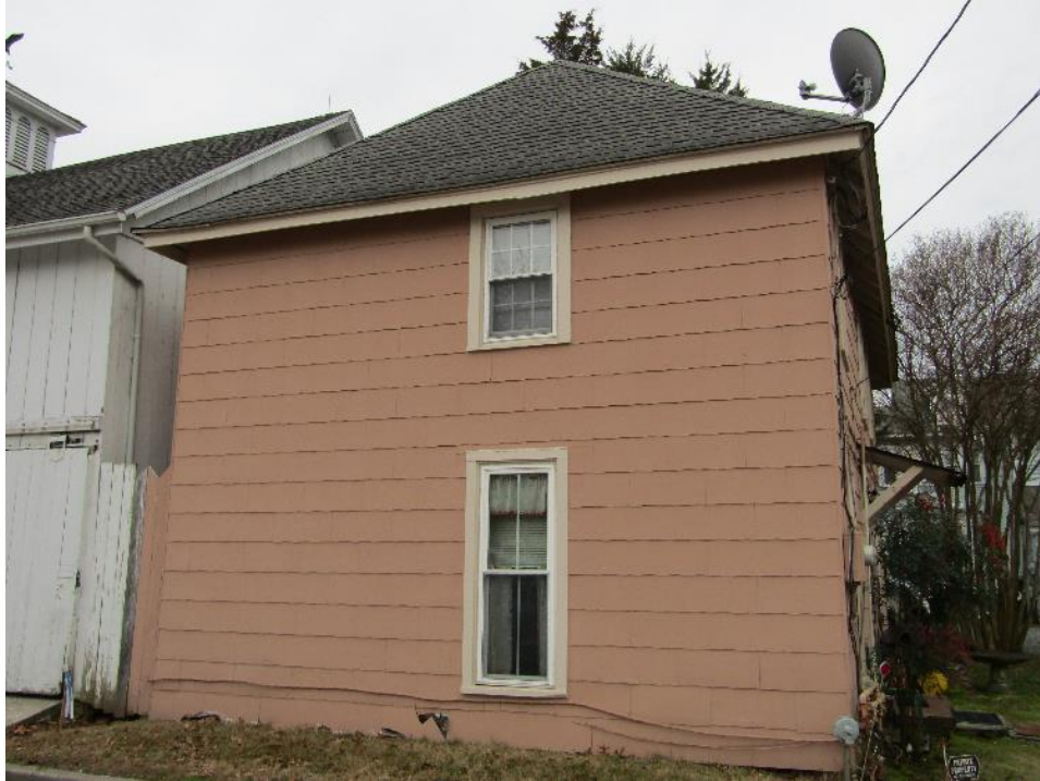
PHOTOGRAPH 15 East elevation of the two-story out-building.
