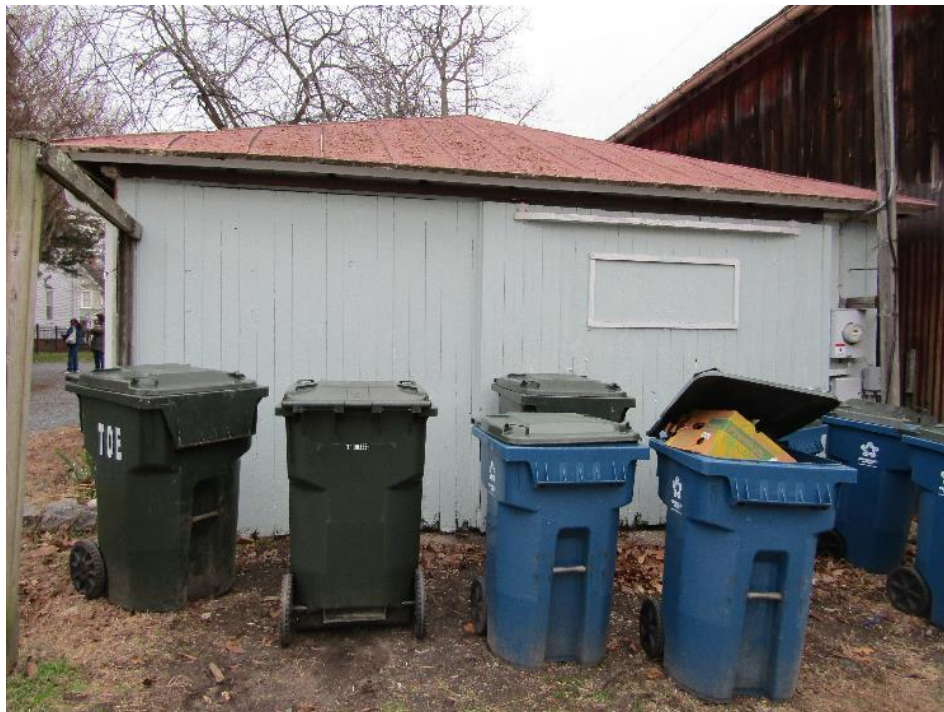
PHOTOGRAPH 22 East elevation of the one-story out-building.
