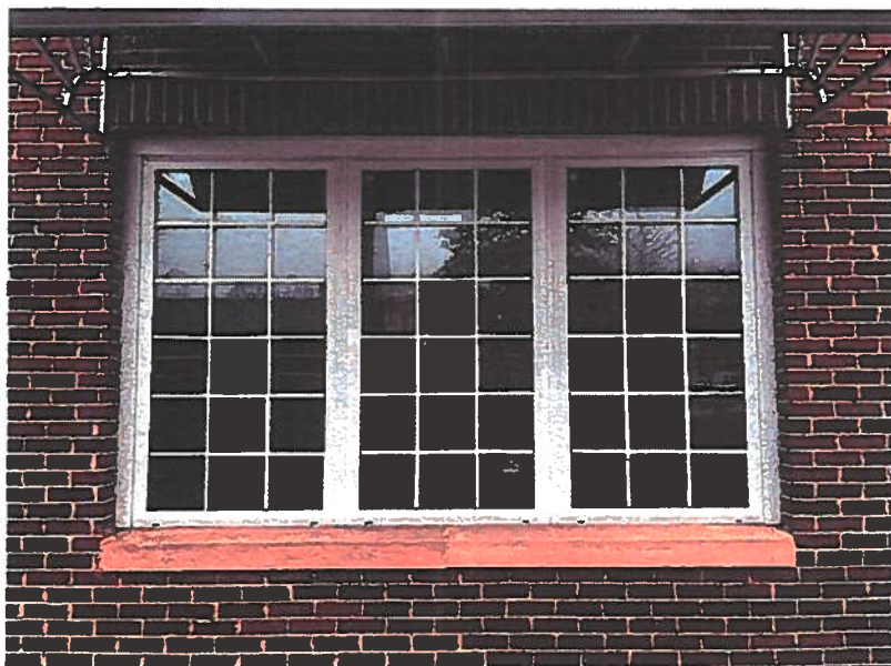
Existing Window No. 3
