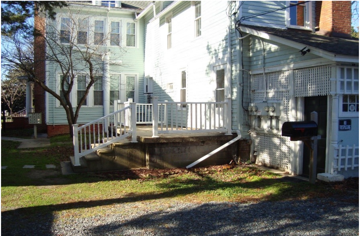
Southeast view of the main structure
