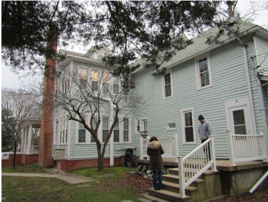
PHOTOGRAPH 5 South elevation of the main building.
