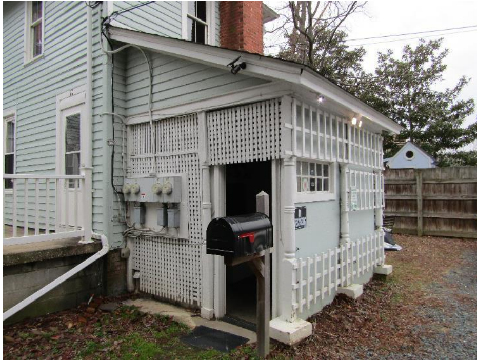
PHOTOGRAPH 9 East end of the main building.
