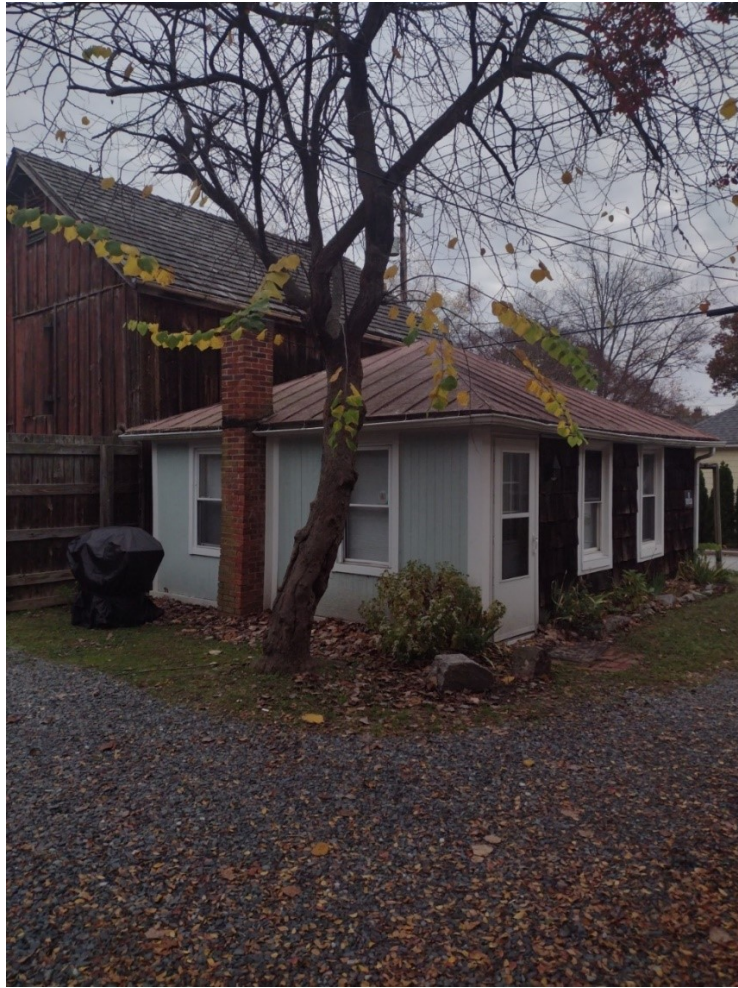
Northeast side view of the North outbuilding
