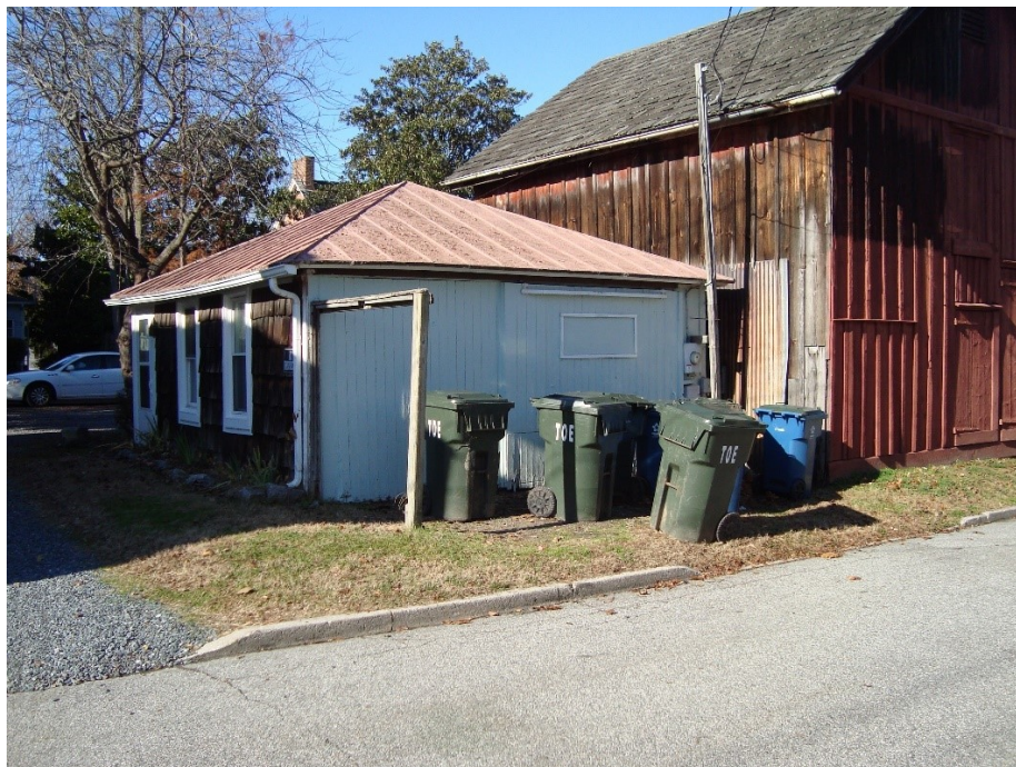
Alley view of the North outbuilding
