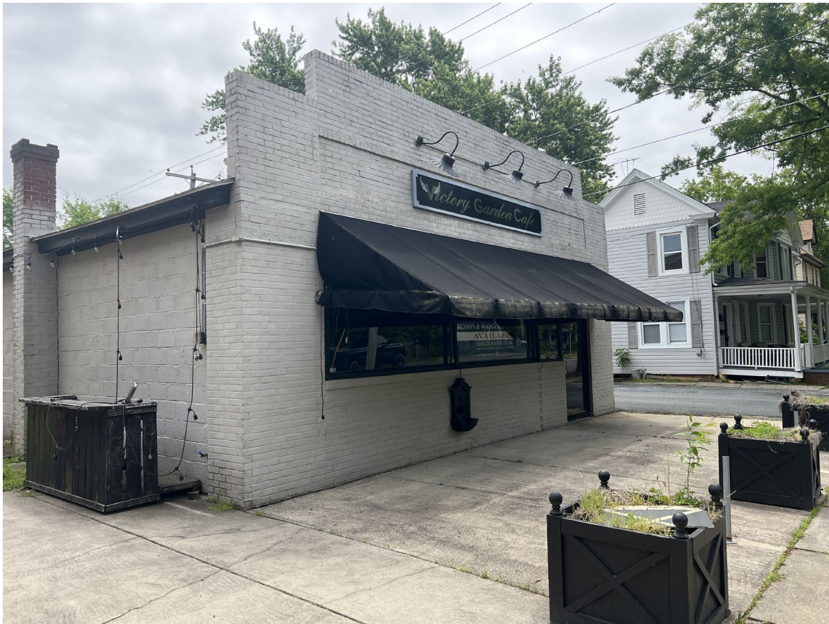
Beaux Monde Fitness Facility 124 S. Aurora Street, Easton MD
