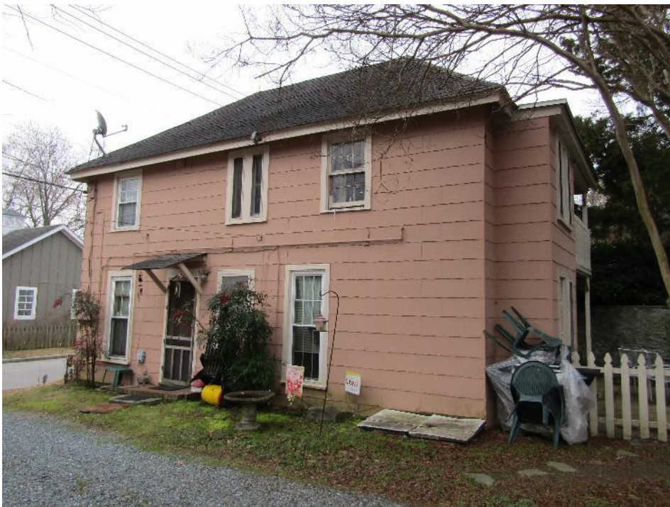
PHOTOGRAPH 14 North elevation of the two-story out-building.
