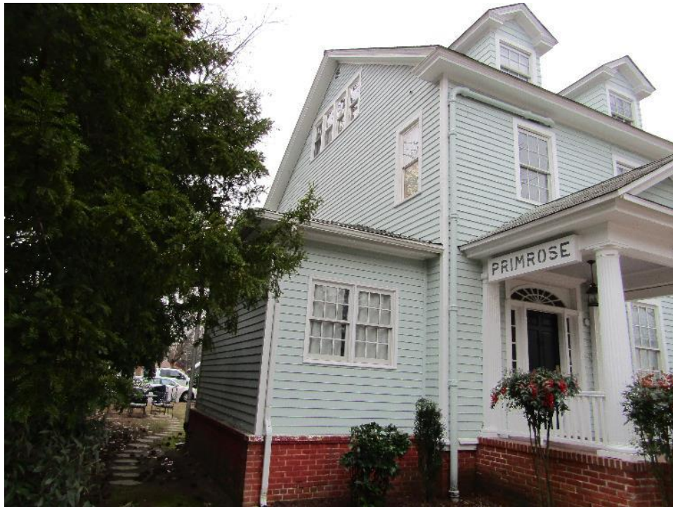
PHOTOGRAPH 3 North elevation of the main building.
