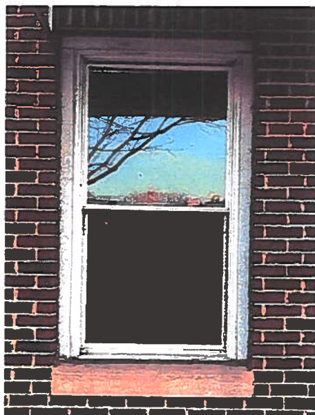
Existing Window No. 1
