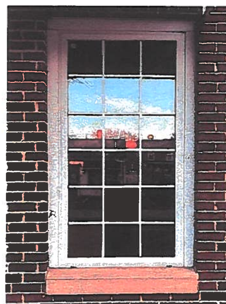
Existing Window No. 2
