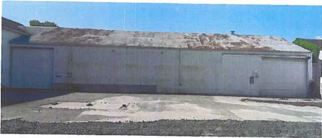
EXISTING CONDITIONS EXTERIOR BUILDING 4
