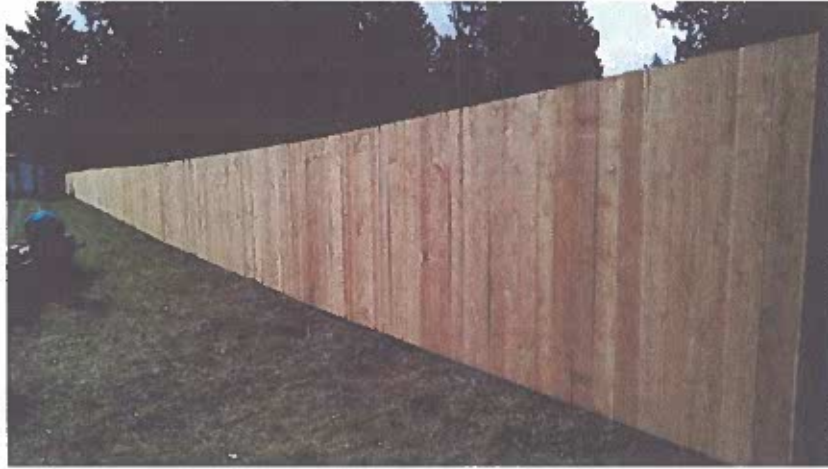
Straight board Fence
