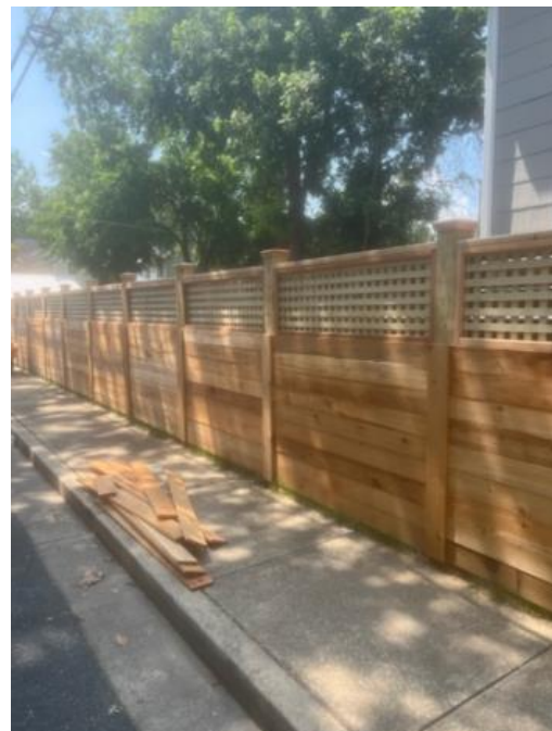
Higgins Street Fence as Installed
