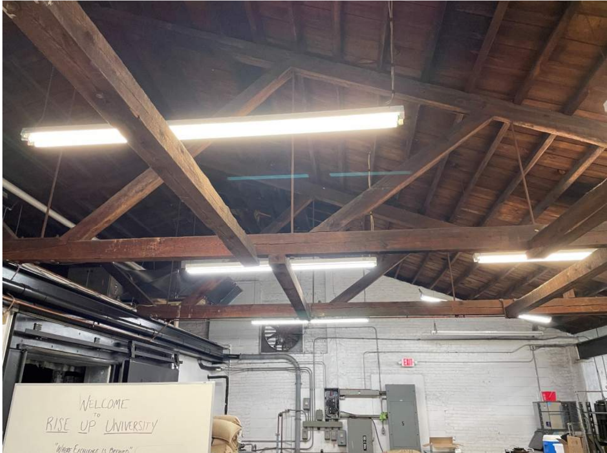
Photograph No. 1: Overall View of Existing Timber Trusses
