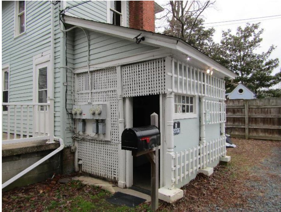
PHOTOGRAPH 9 East end of the main building.
