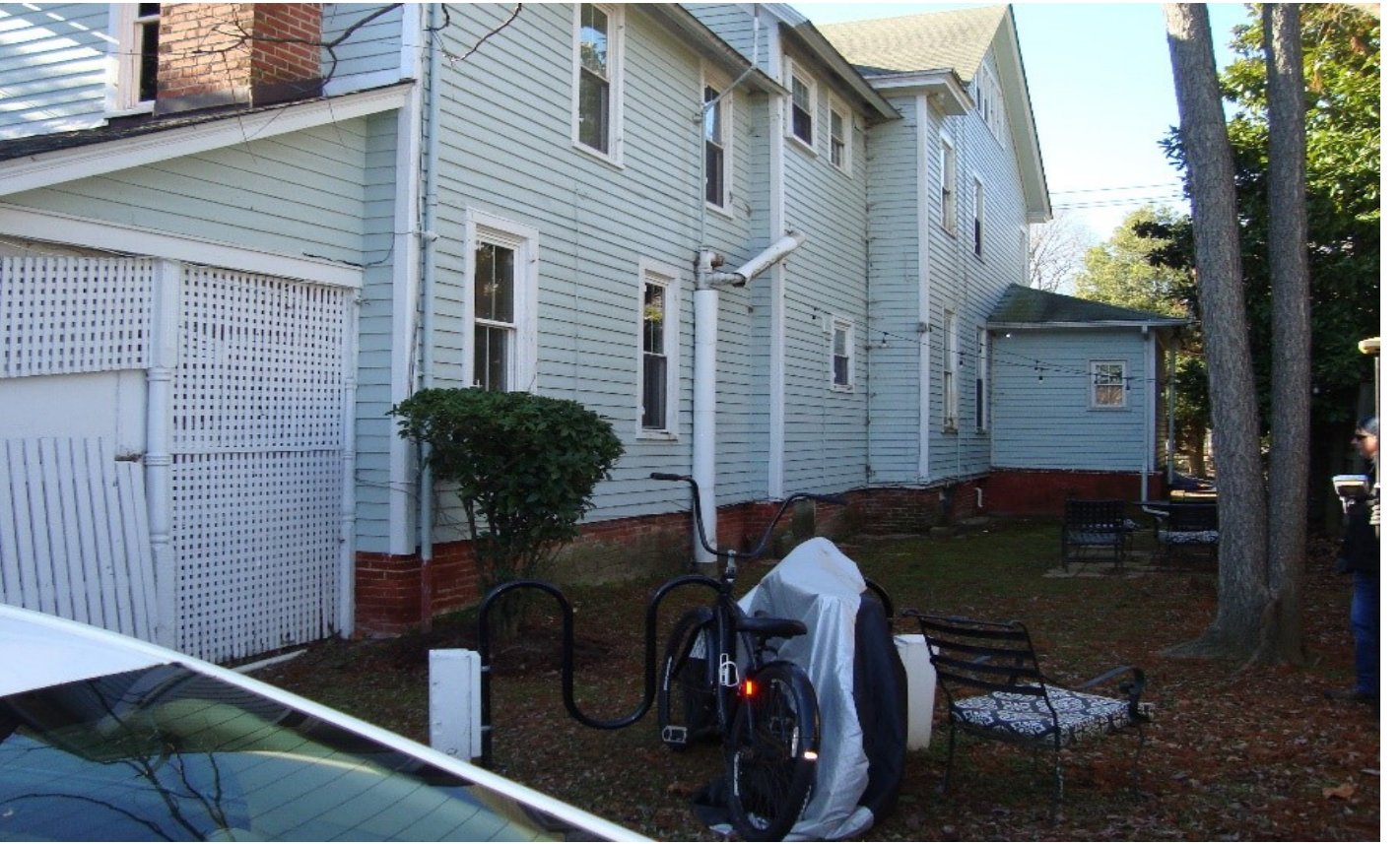
Northeast view of the main structure
