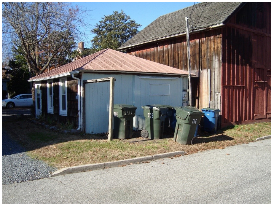
Alley view of the North outbuilding
