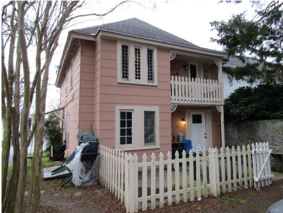
PHOTOGRAPH 13 West elevation (front) of the two-story out-building.
