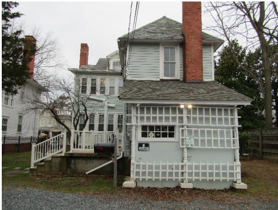
PHOTOGRAPH 4 East elevation of the main building.
