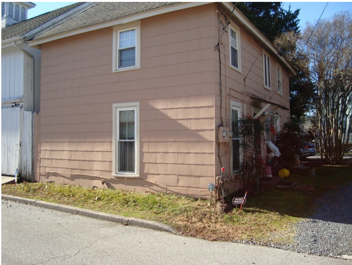
Alley view of the South outbuilding
