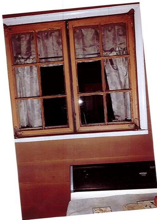
Figure 1 Existing Casement Window
