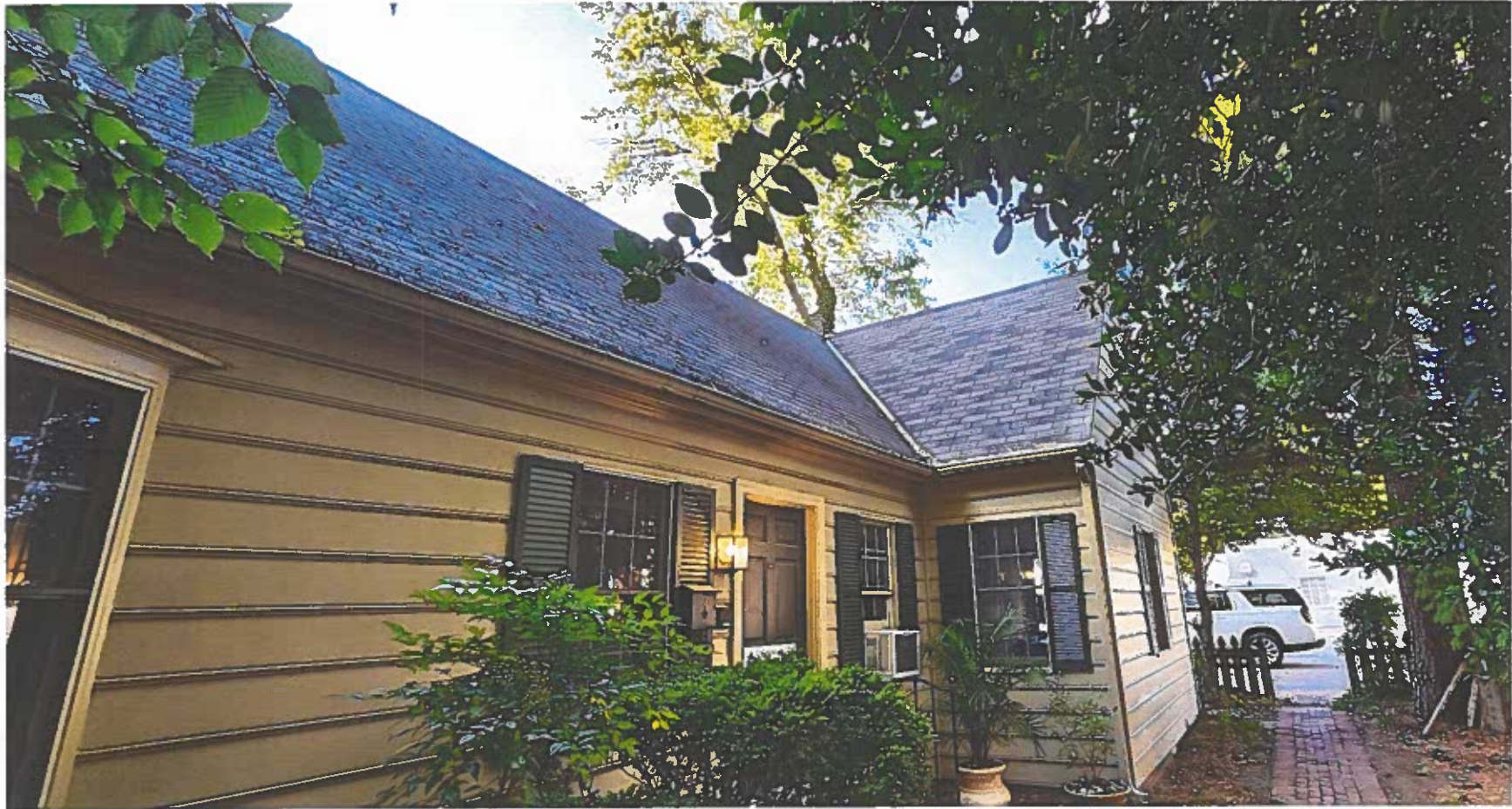
REAR BUILDING, EAST SIDE:
