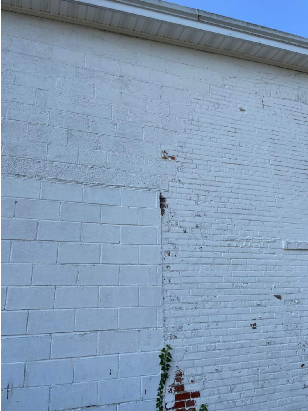
Photograph No. 20: Exterior Wall Transition from Original Brick Wall to Addition CMU Wall
