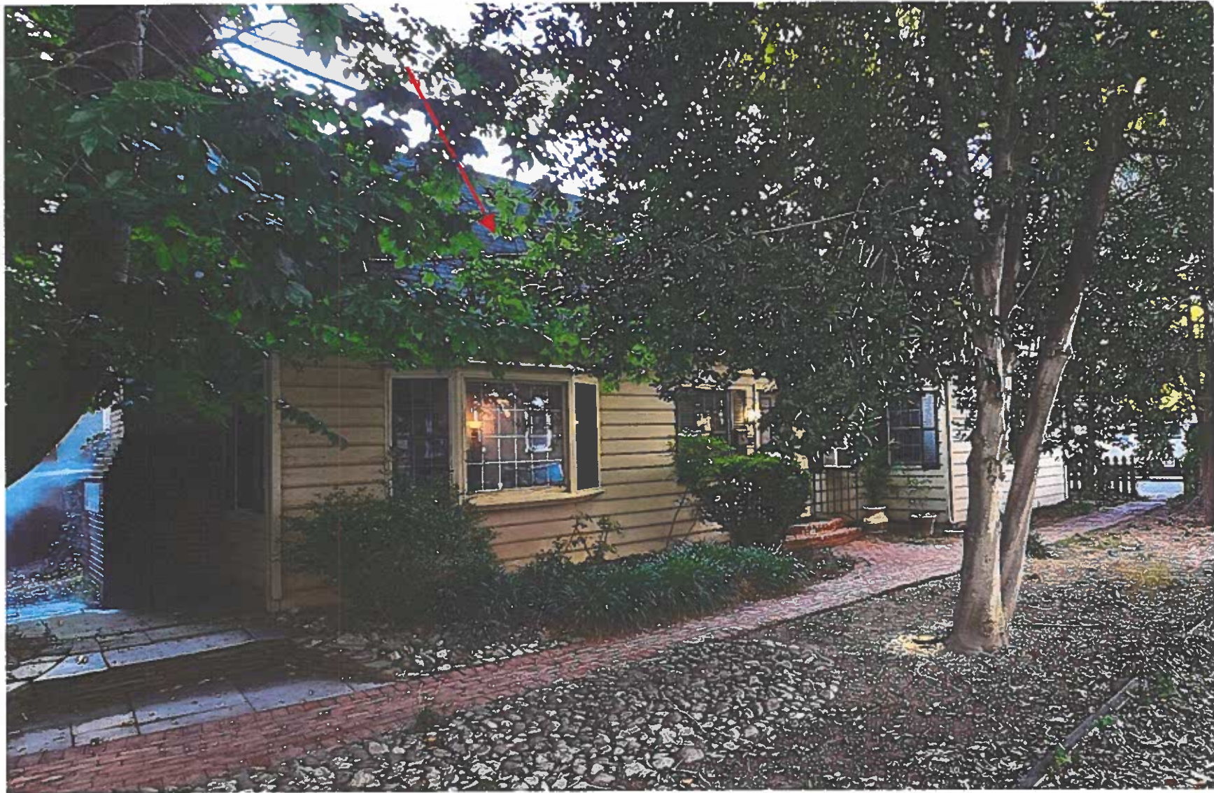
REAR BUILDING, EAST SIDE:
