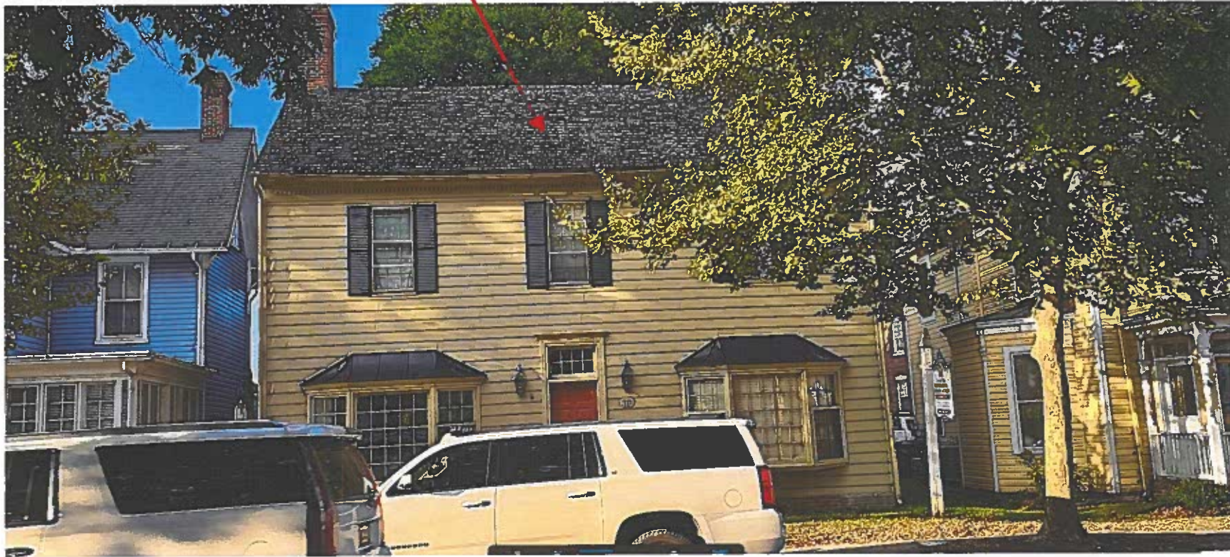
FRONT BUILDING, FRONT ELEVATION:
