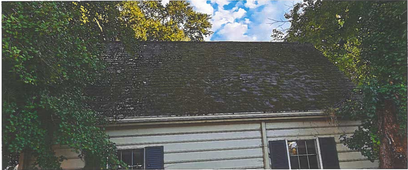
REAR BUILDING, REAR (NORTH) SIDE:
