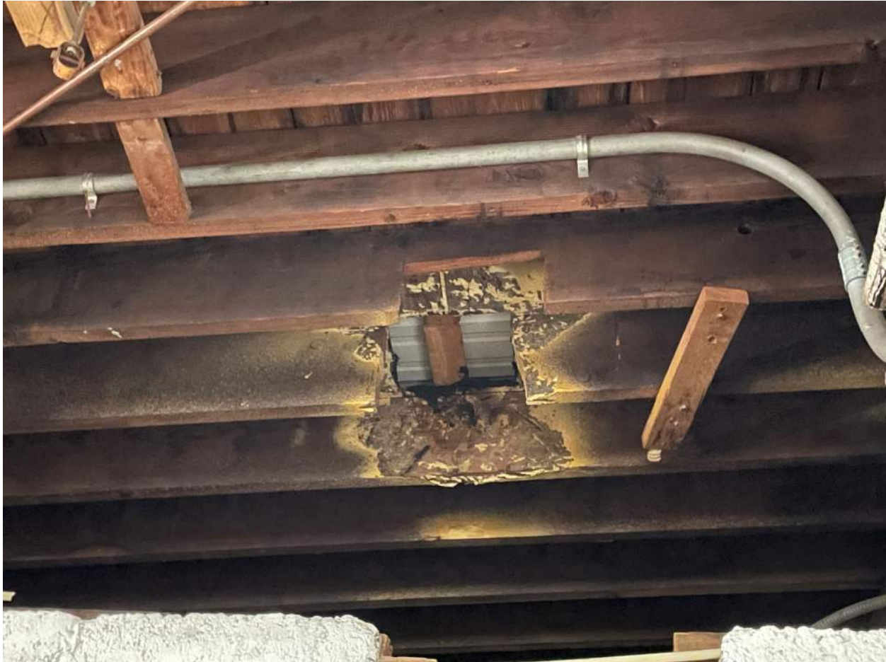
Photograph No 18: Existing Rafters Cut At Roof Level
