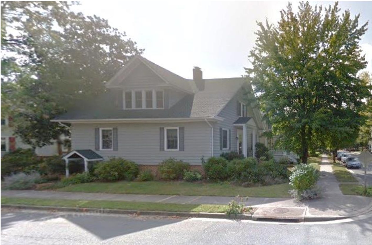
300 S Hanson Street (Side View)
