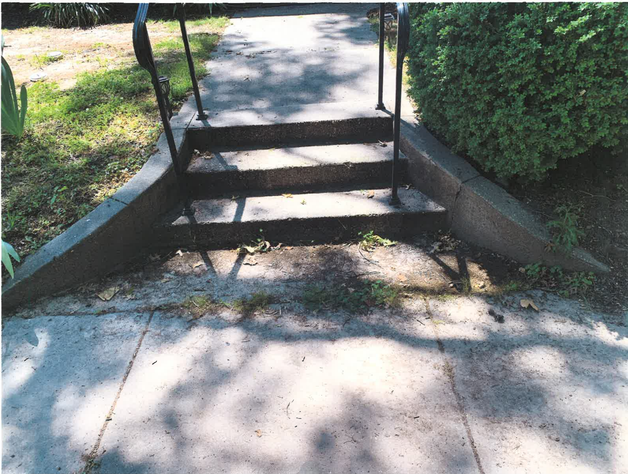
EXISTING FRONT STAIRWAY
