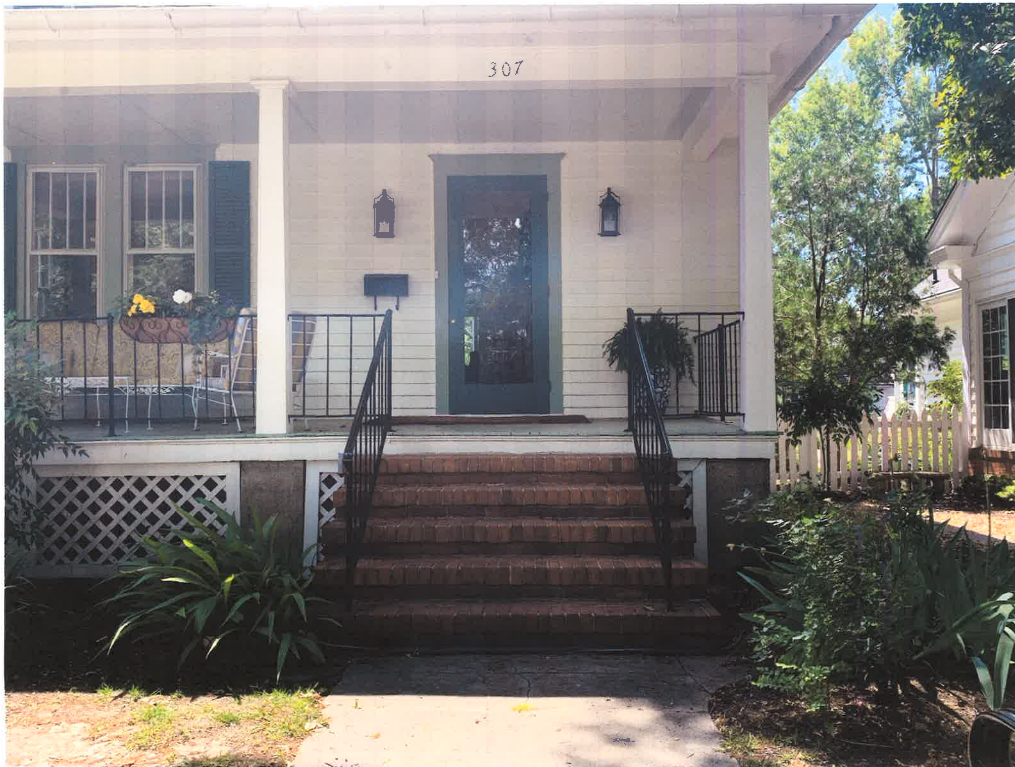
EXISTING FRONT PORCH STAIRWAY
