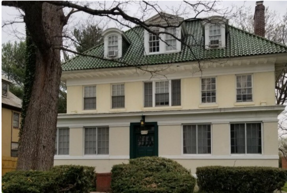
Exterior with Spanish Tile Roof
