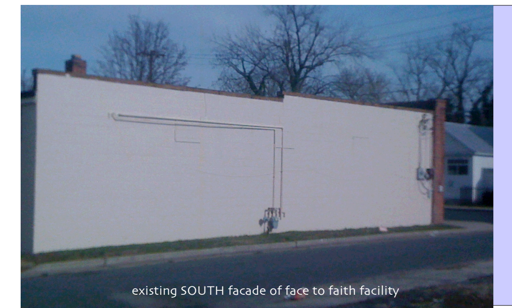
existing SOUTH facade of face to faith facility
