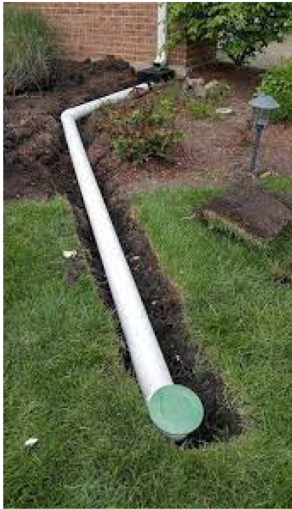
PVC PIPING TO POP-UP EMITTER DETAIL (NOT TO SCALE)
