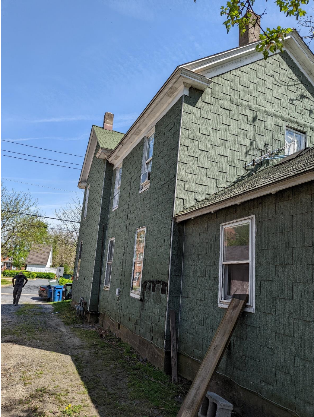
Picture 2: Existing condition right from rear
