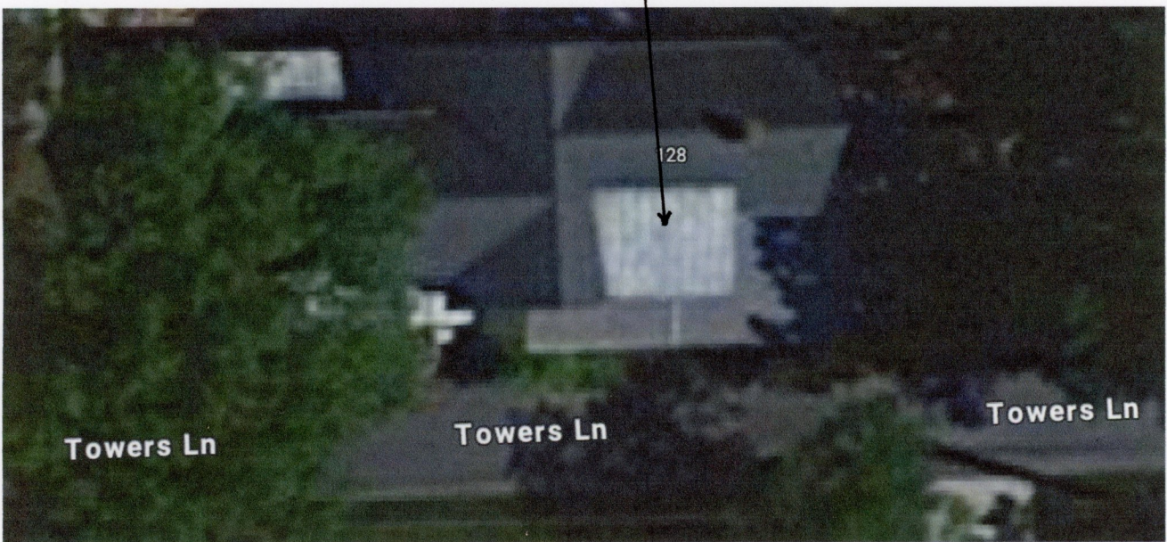
128 S Harrison - Satellite Photo Showing Metal Roof
