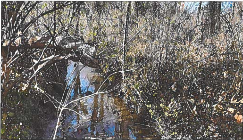
PHOTO 3. STREAM IS STRAIGHTENED AT CULVERT (PHOTO 2) AND FLOODPLAIN IS NONEXISTENT DUE TO ROAD CONSTRAINTS.
