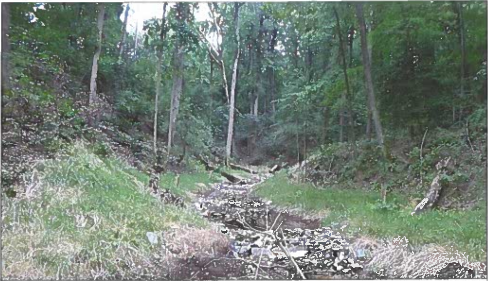
PHOTO 3. COBBLE WEIRS WITH WOODY DEBRIS ENSURE THAT STREAM MAINTAINS LATERAL STABILITY AND DOES NOT MIGRATE Laterally.
