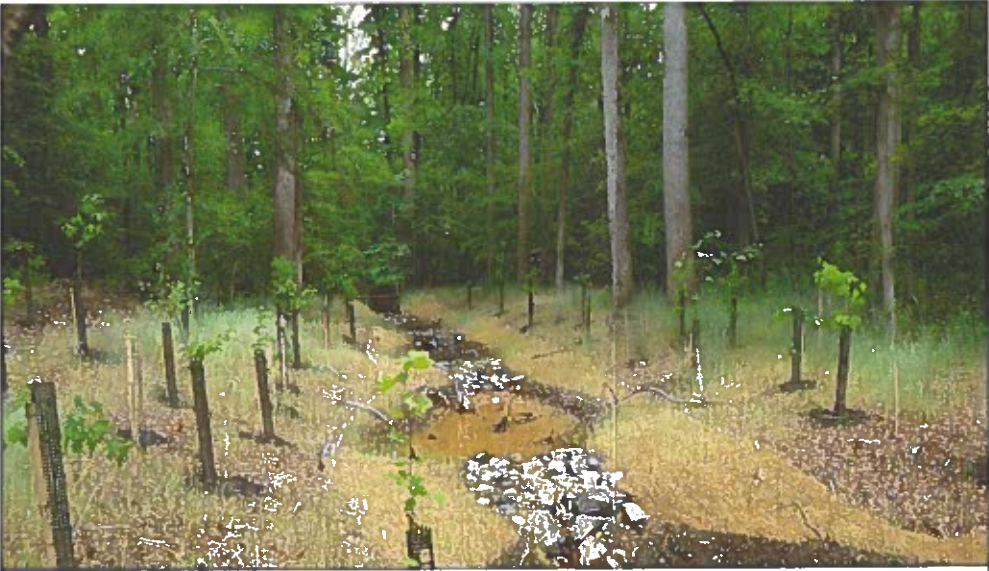
PHOTO 4. VEGETATION IS PLANTED WITHIN THE BANKFULL WITH OF EXAMPLE PROJECT SO TREES WILL BE FED BY CHANNEL.
