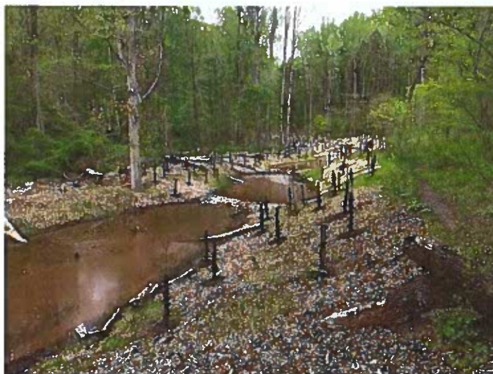
RSC restoration implemented for Arundel Rivers Federation.
