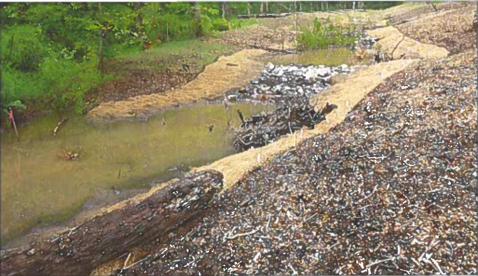
PHOTO 2. EXAMPLE PROJECT SHOWING CONSTRUCTED POOLS AND COBBLE WEIRS WITH LARGE WOOD TO PROVIDE ADDITIONAL ROUGHNESS.
