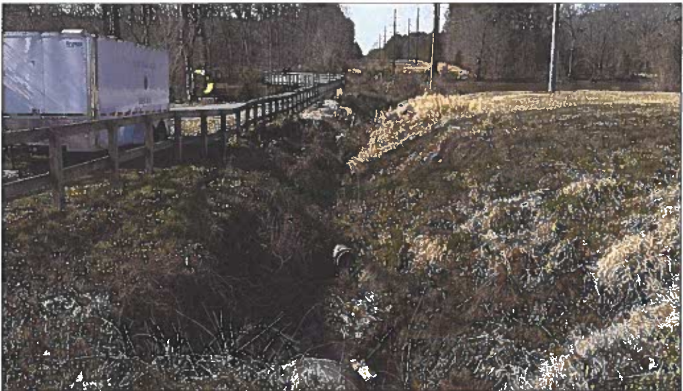
PHOTO 2. EXISTING STREAM RUNS PARALLEL TO EXISTING TRAIL, DISPLAYING SIGNS OF HISTORIC STRAIGHTENING.
