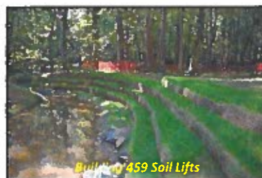
Mount Vernon Slope Stabilization
