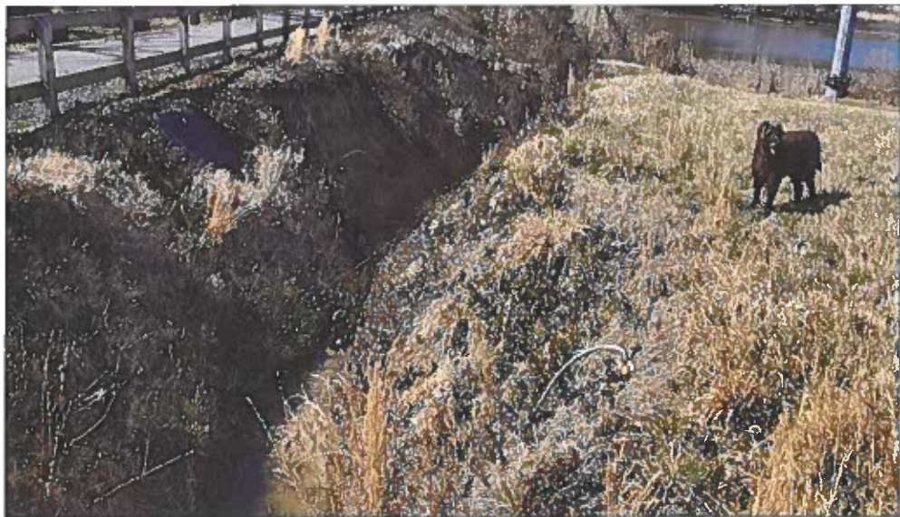
PHOTO 3. STREAM IS DEEPLY INCISED AND DOWNCUTTING IS ENCROACHING ON THE NEARBY TRAIL WALK.
