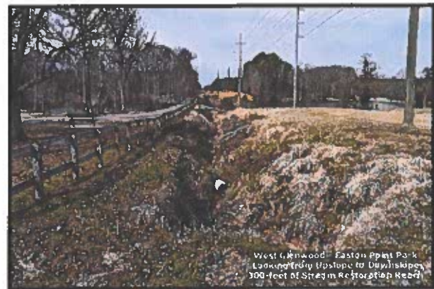
Overview Photo of the West Glenwood Project.
