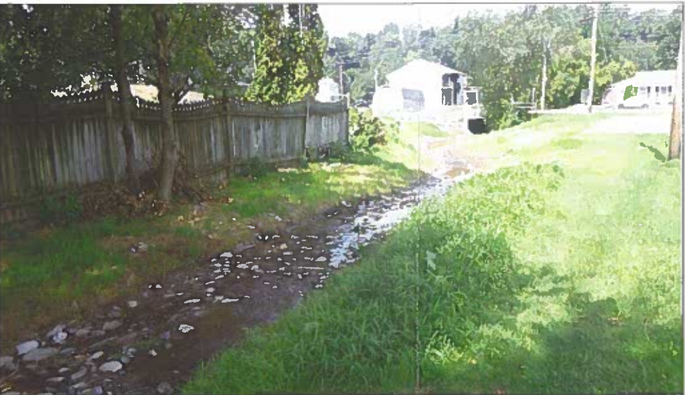
PHOTO 2. EXAMPLE PROJECT SHOWS STREAM COEXISTING WITH NEARBY RESIDENCE. VIEW UPSTREAM OF CONSTRUCTED RIFFLE.
