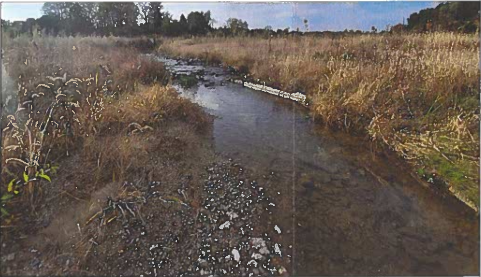
PHOTO 1. EXAMPLE PROJECT WITH STABLE RIFFLE POOL PLANFORM SHOWCASING A STABLE ENTRENCHMENT RATIO WITH NO VISIBLE INCISION.
