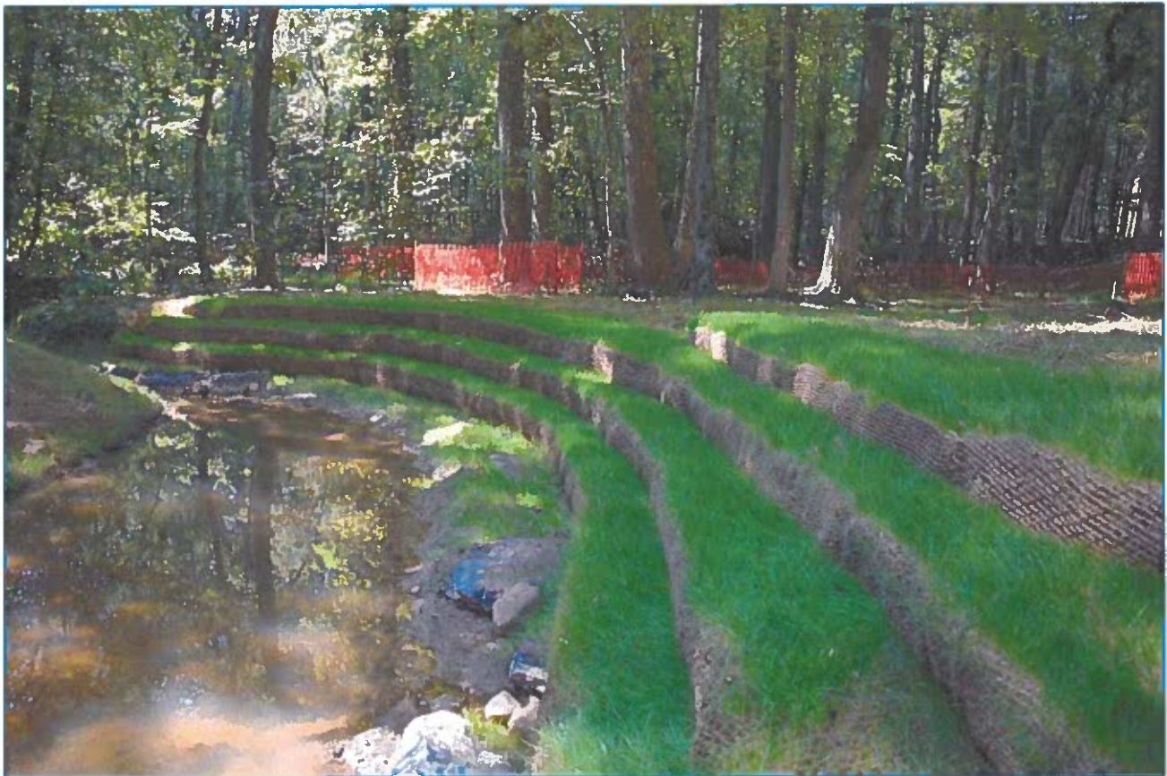
The project included the construction of in-channel riffle grade control, soil lifts and the creation of an off-line vernal herb pool, which was the remains of a hairpin meander bend, sealed-off in the realignment of the stream.
