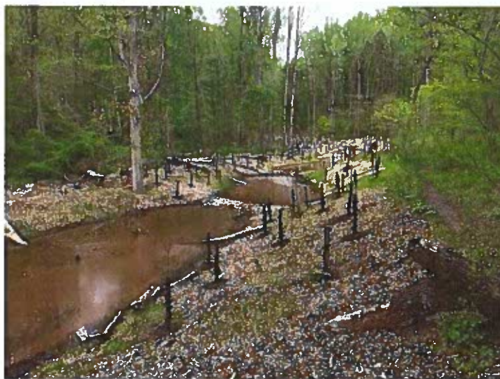
RSC restoration implemented for Arundel Rivers Federation.
