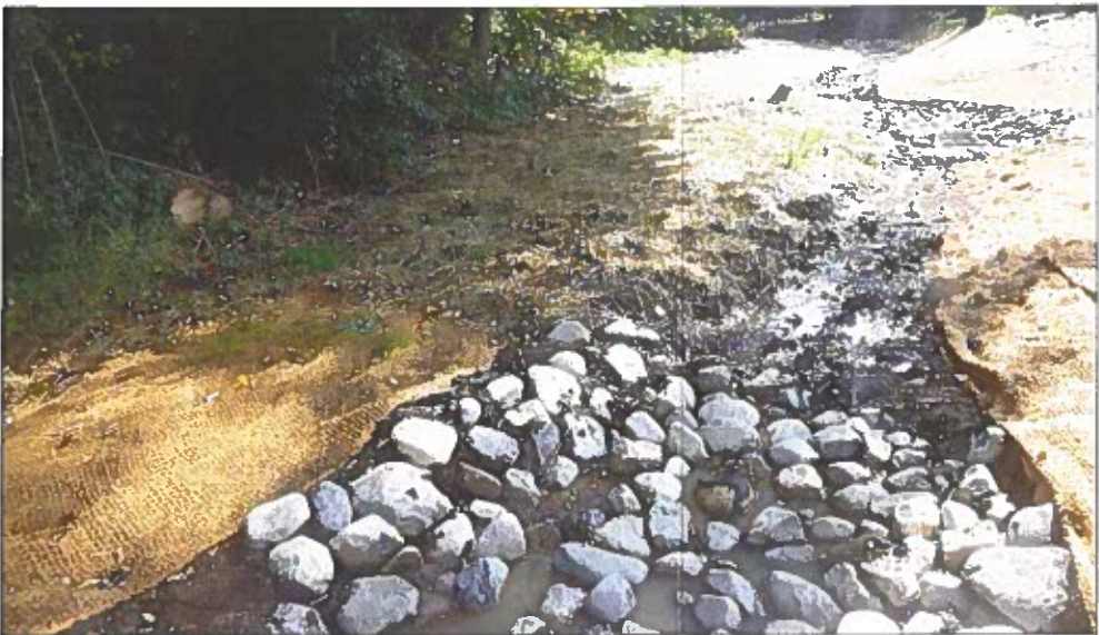
PHOTO 3. EXAMPLE PROJECT DISPLAYING A BANKFULL BENCH AND CONSTRUCTED RIFFLE.
