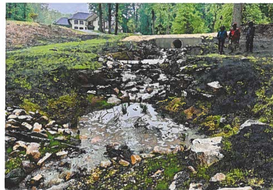
Proposed Condition - Cascade structure
