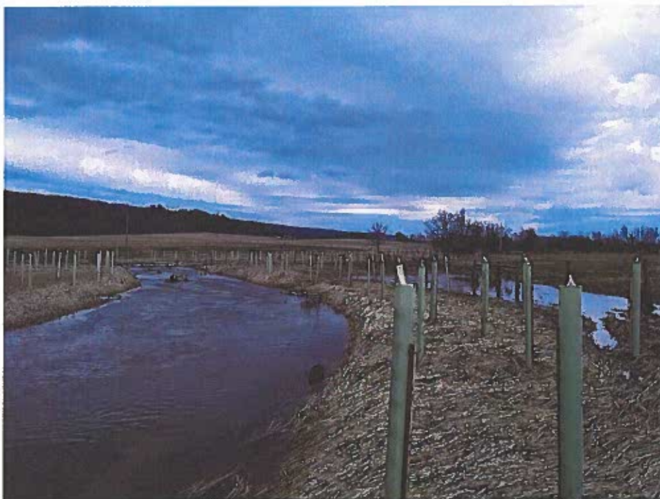
NCD P2 floodplain reconnection and channel realignment, PA.
