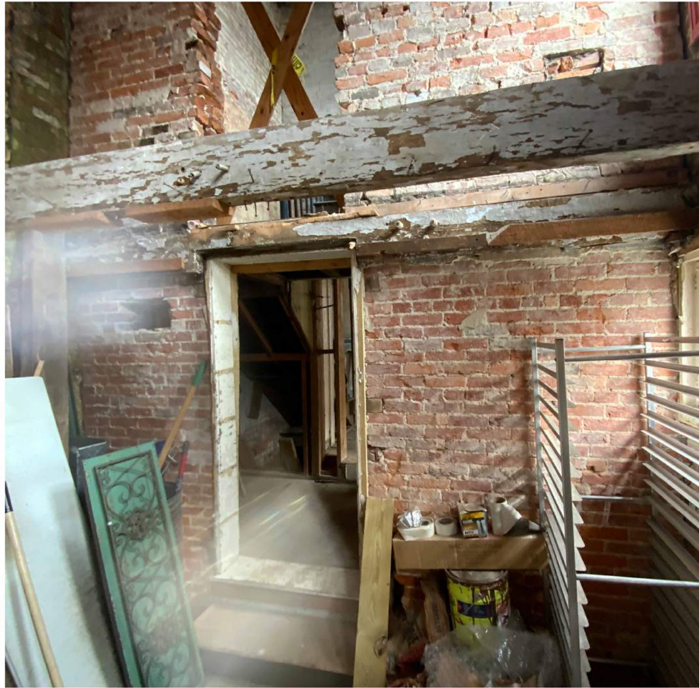
IP-5 VIEW AT ENTRY FLOOR LOOKING EAST
