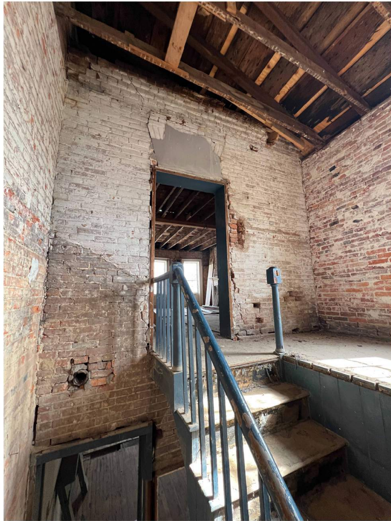
IP-1 VIEW STANDING ON LANDING LOOKING EAST
