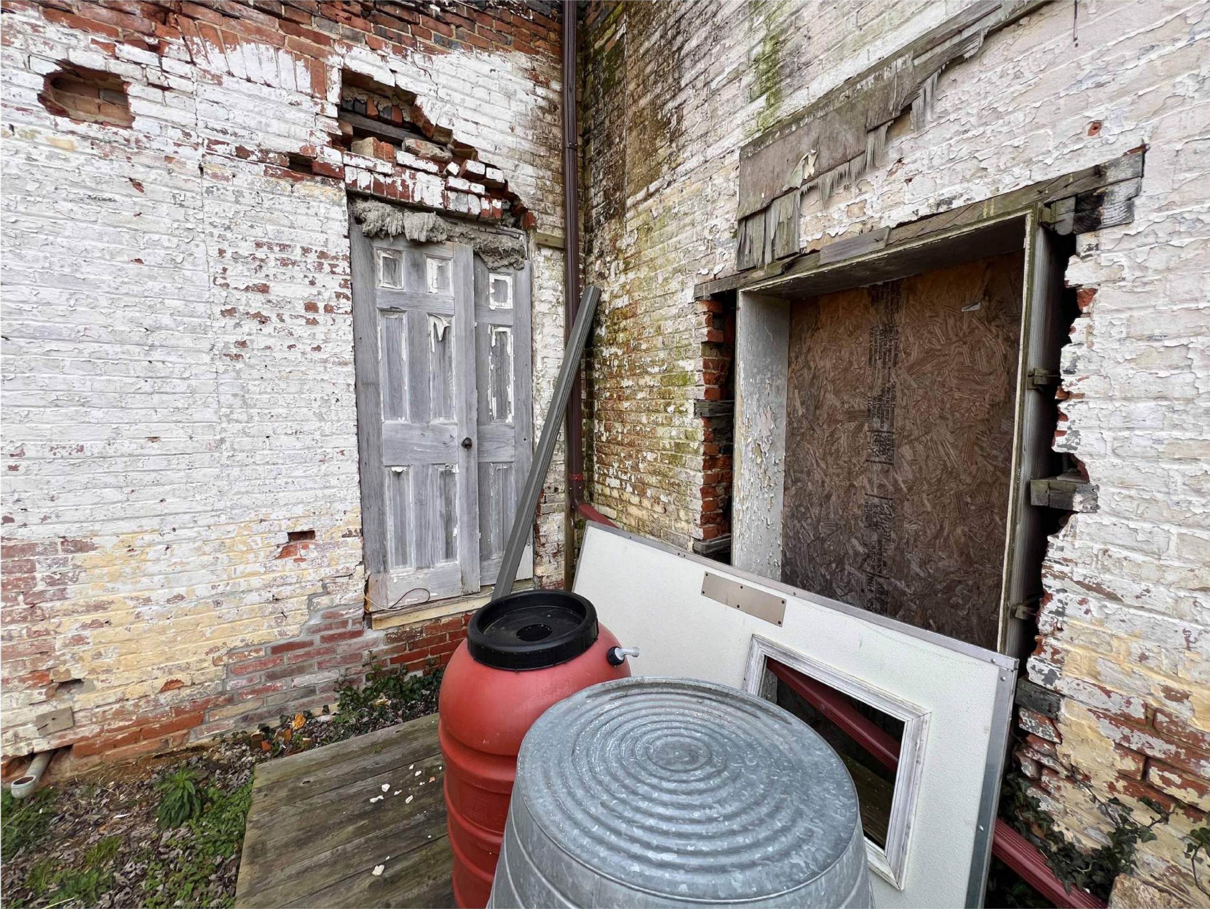
EP-4 VIEW LOOKING EAST, WEST ELEVATION
