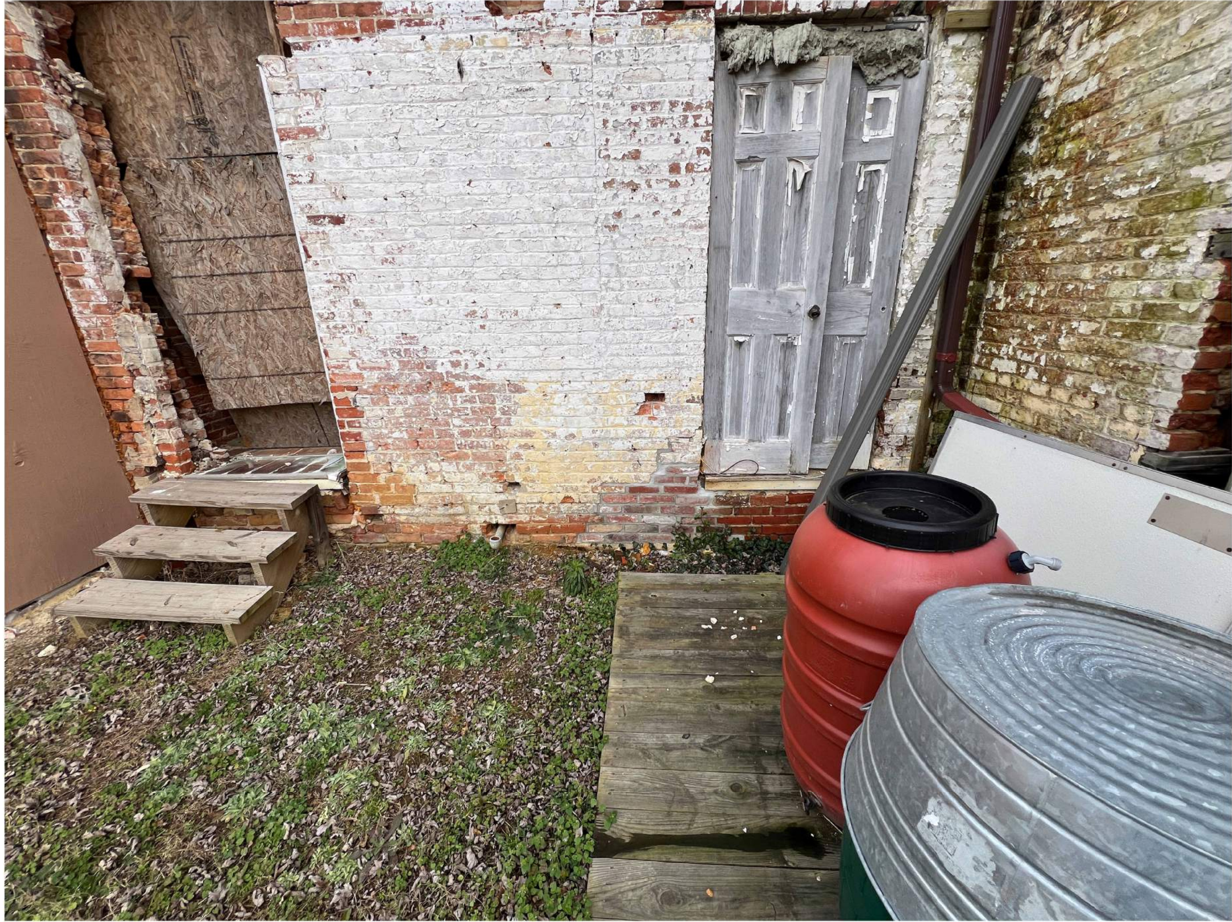
EP-3 VIEW LOOKING EAST, WEST ELEVATION
