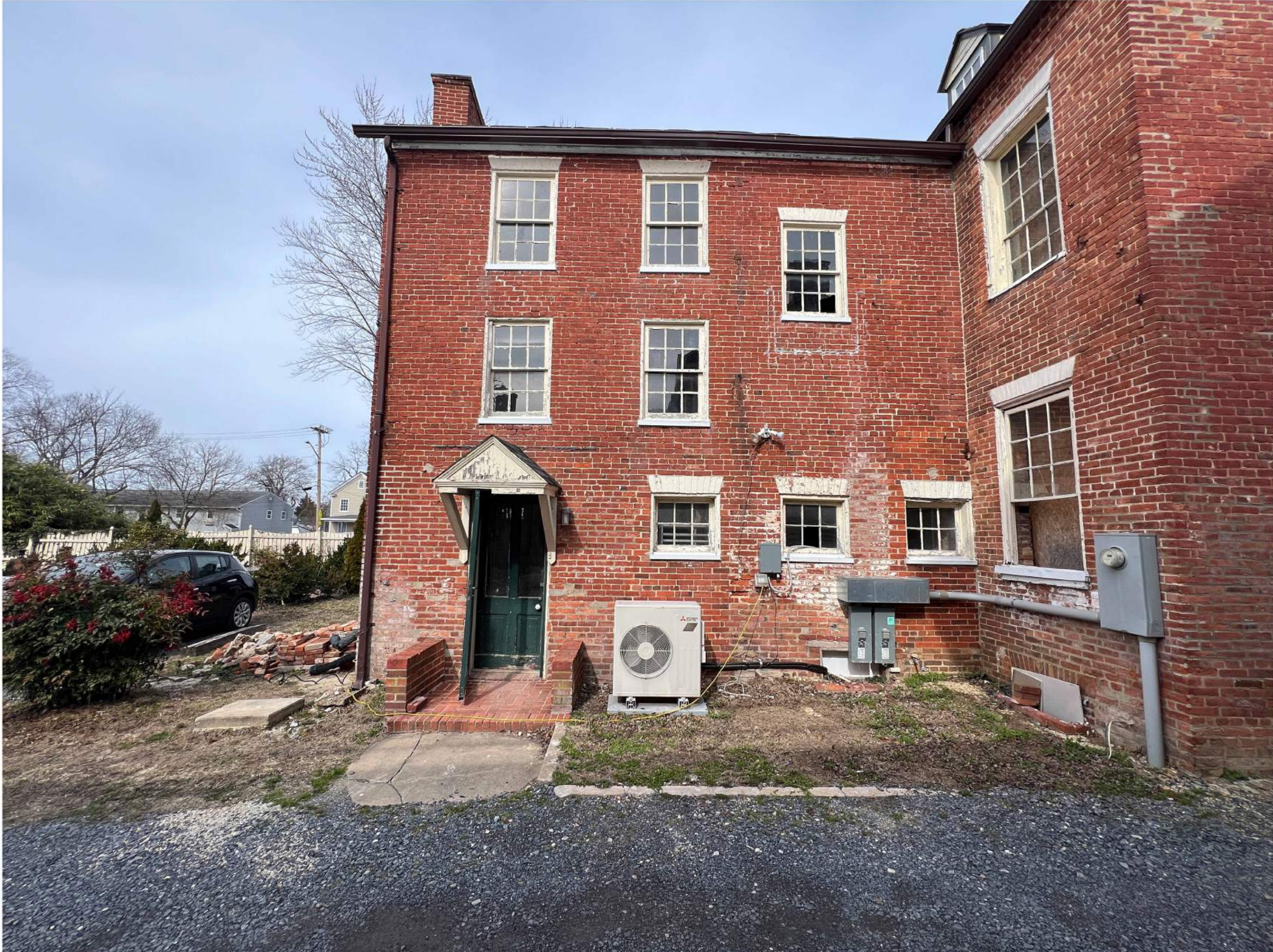
EP-6 VIEW LOOKING NORTH, SOUTH ELEVATION
