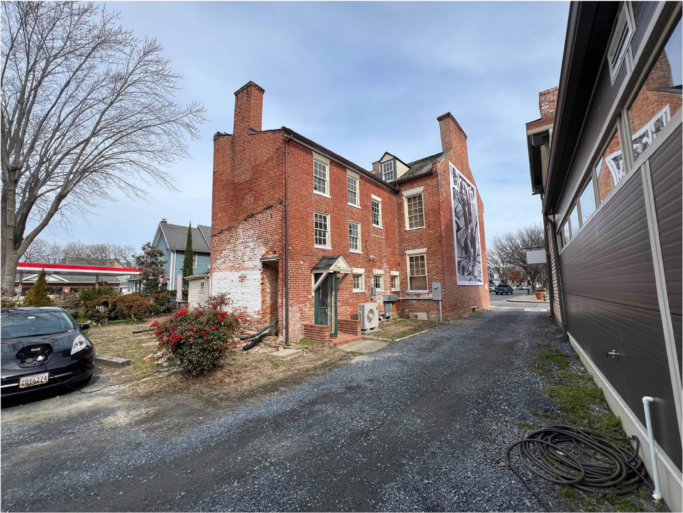
EP-5 VIEW LOOKING NORTH EAST
