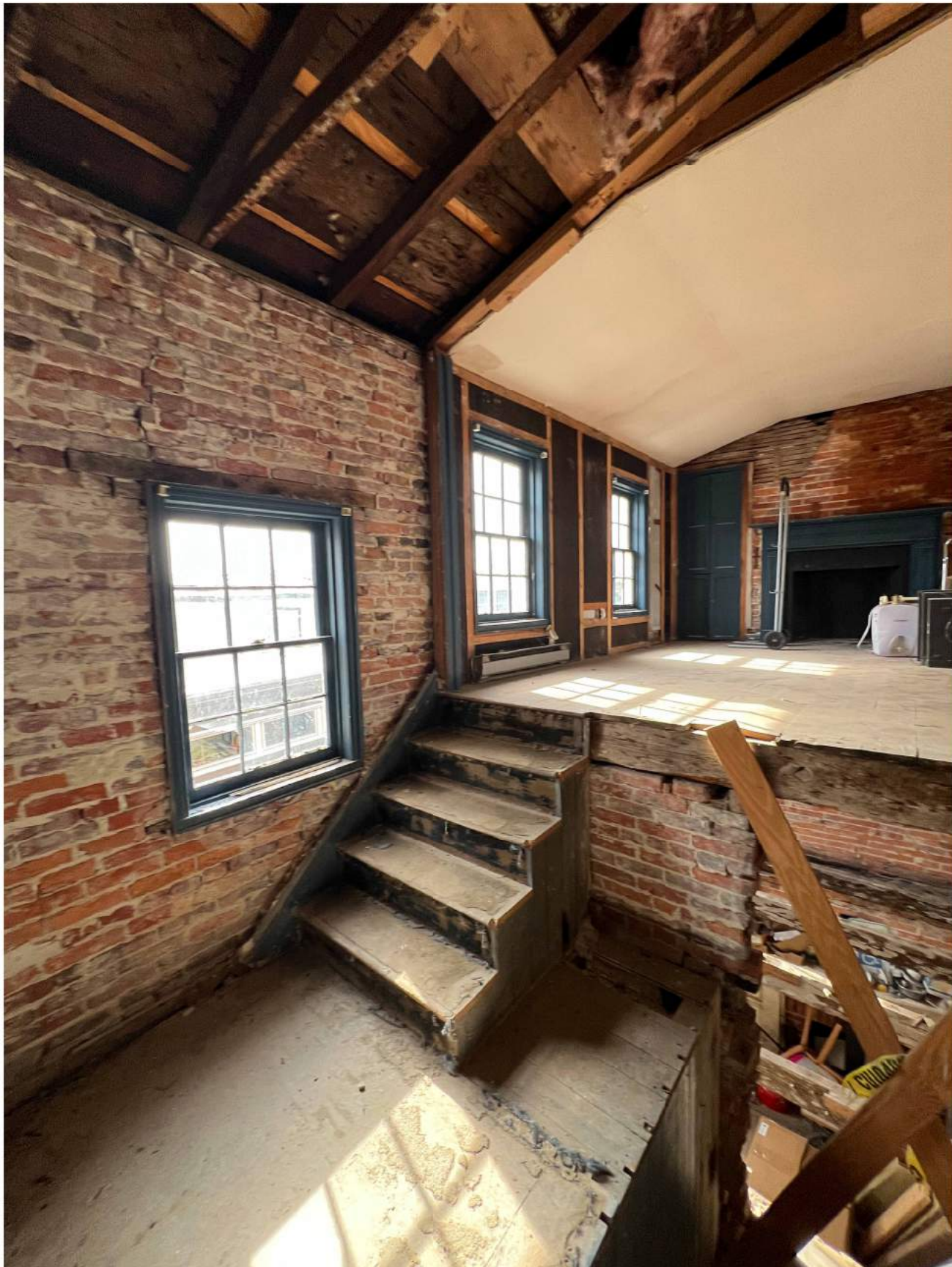
IP-3 VIEW STANDING ON LANDING LOOKING SOUTHWEST
