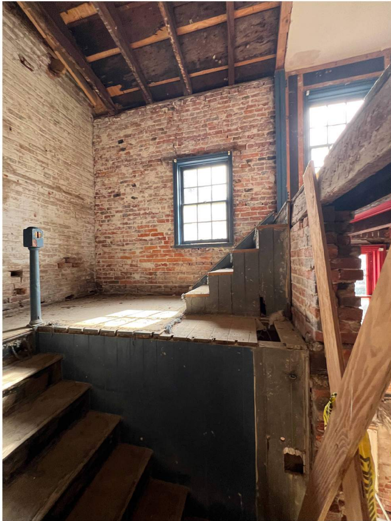
IP-2 VIEW STANDING ON LANDING LOOKING SOUTH
