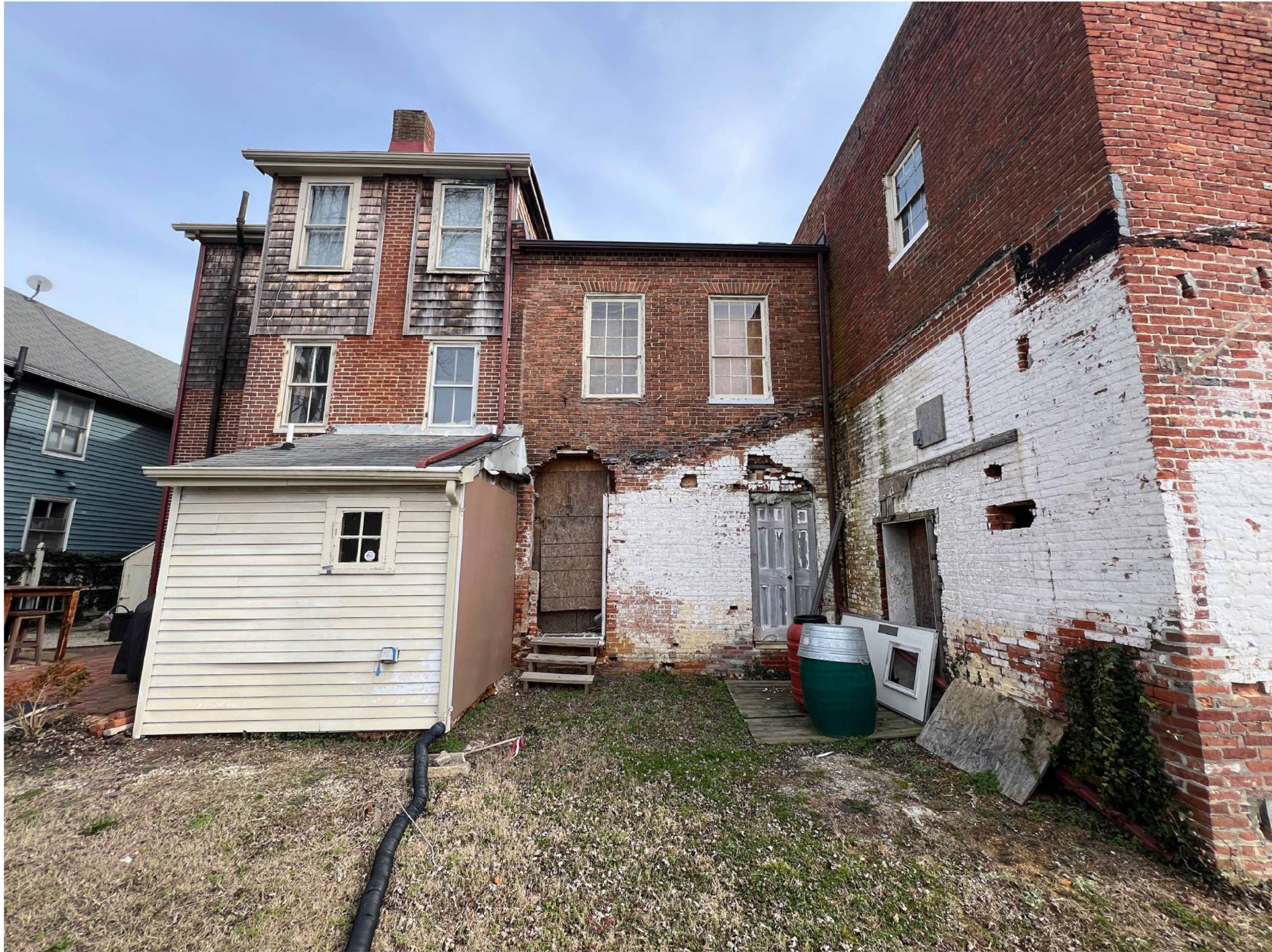
EP-1 VIEW LOOKING EAST, WEST ELEVATION
