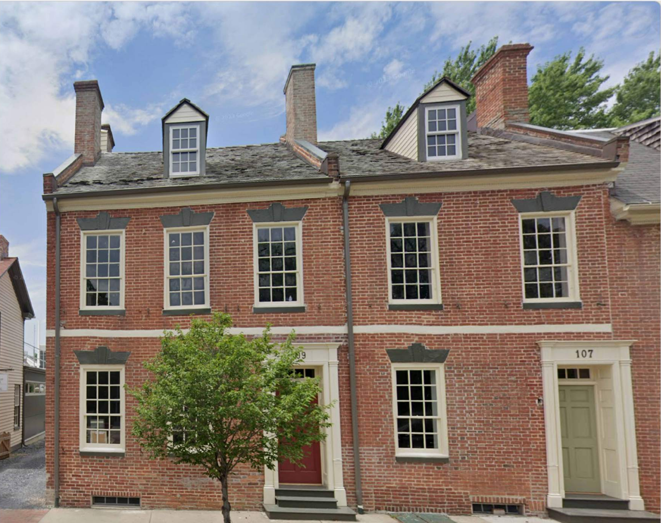
EP-8 VIEW LOOKING WEST, EAST ELEVATION
