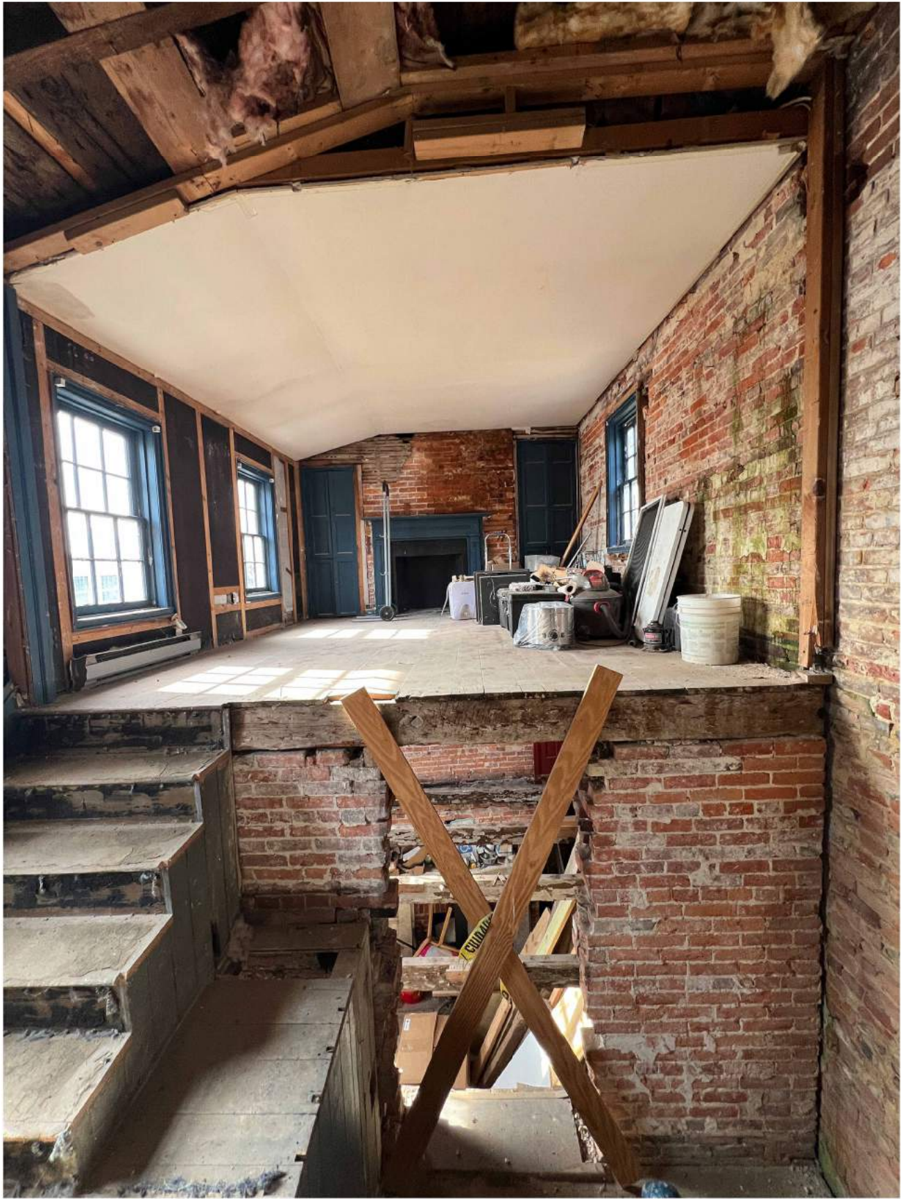
IP-4 VIEW STANDING ON LANDING LOOKING WEST
