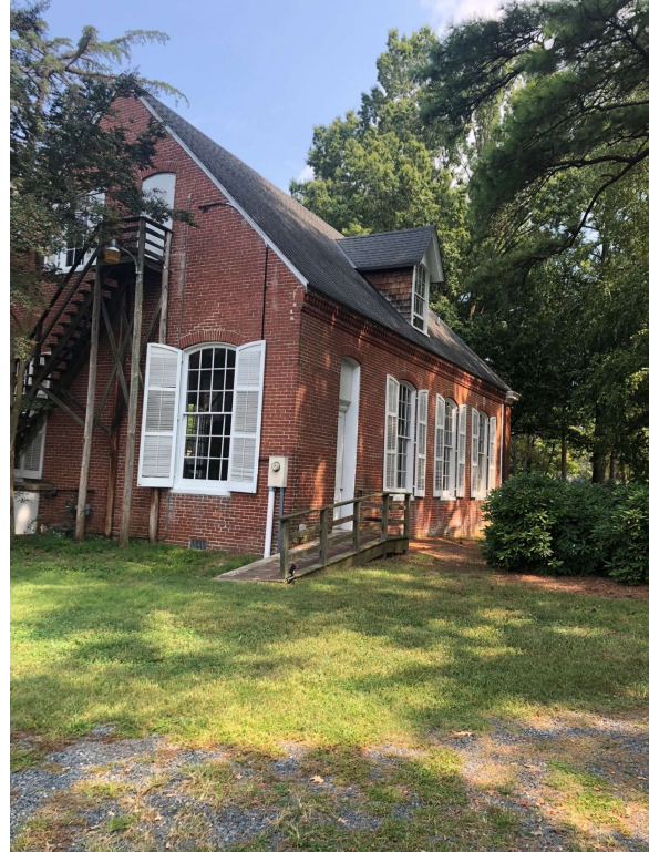
North / South Elevations – showing existing noncompliant ramp
