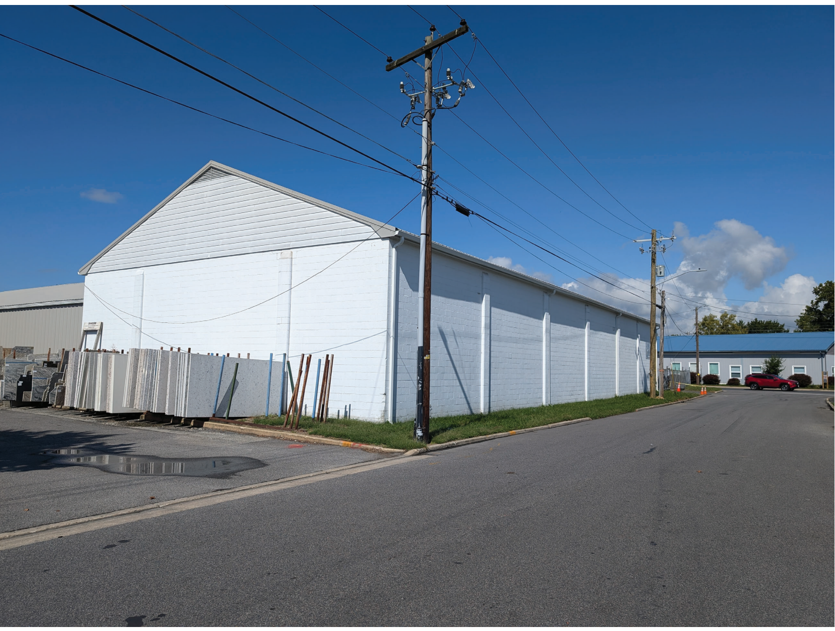
[F] - BUILDING 5 - FUTURE EVENT SPACE FROM SOUTHEAST CORNER AT KEMP LANE
