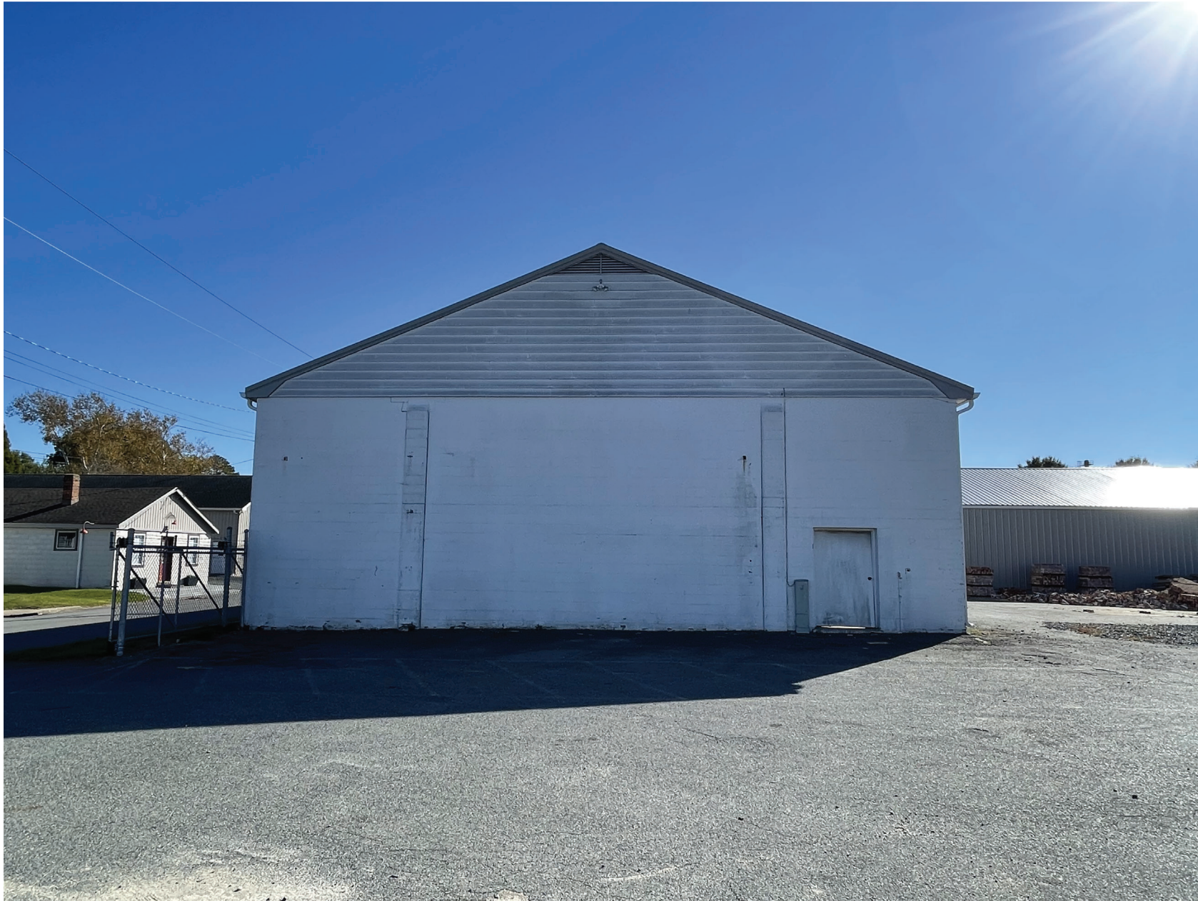
EVENT SPACE MAIN ENTRY FROM NORTH - PRIOR TO RENOVATION
