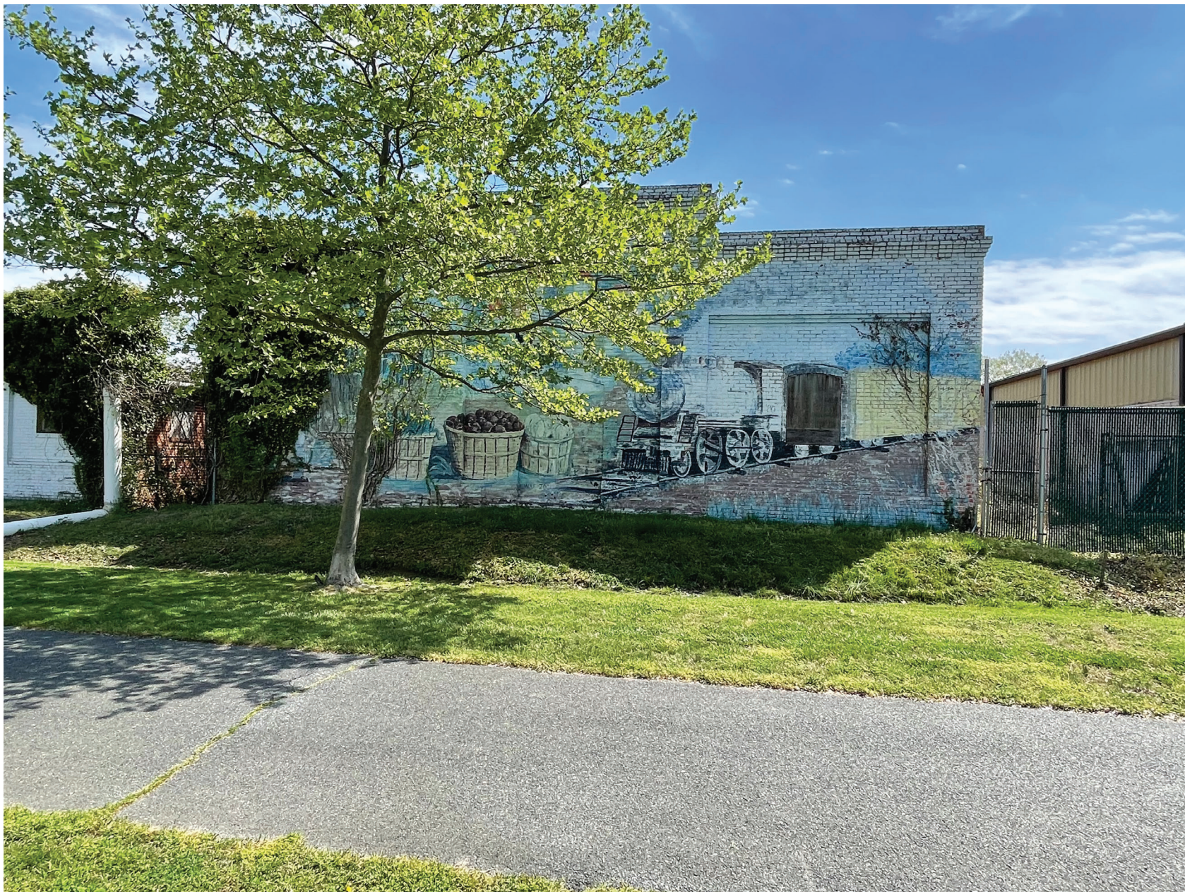
BUILDING 3 - HISTORICAL FACADE FROM WEST AT RAILS TO TRAILS PATHWAY - PRIOR TO RENOVATION
