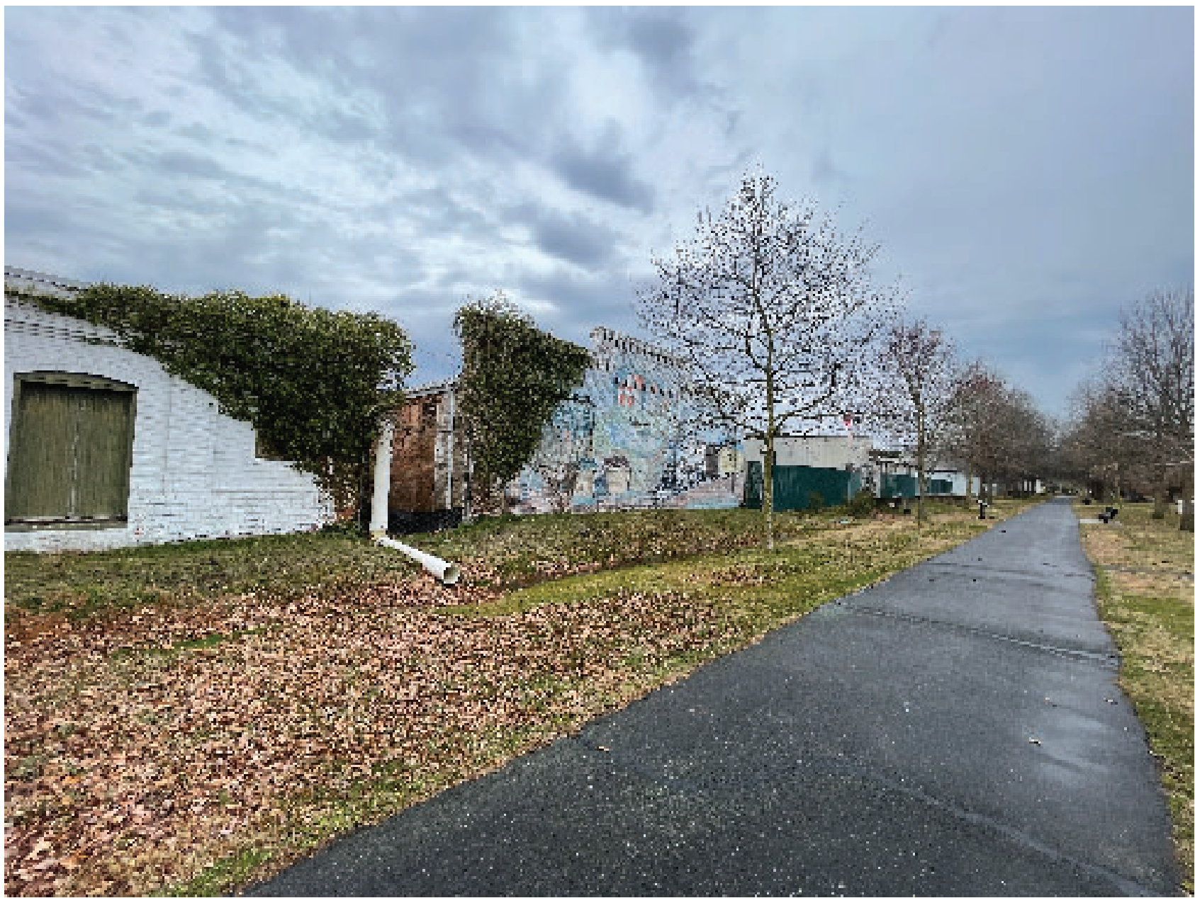
[A] - BUILDING 1 - HISTORICAL FACADE FROM NORTHWEST
