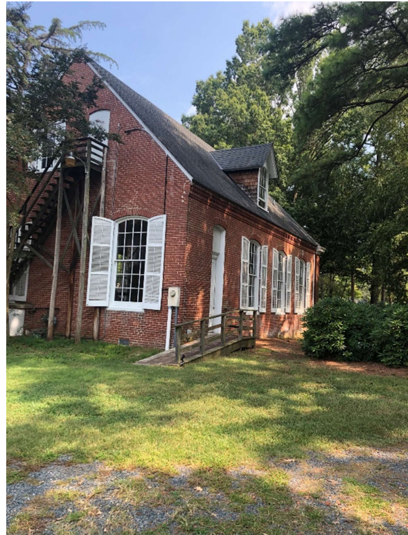
North / South Elevations – showing existing noncompliant stairs & ramp
