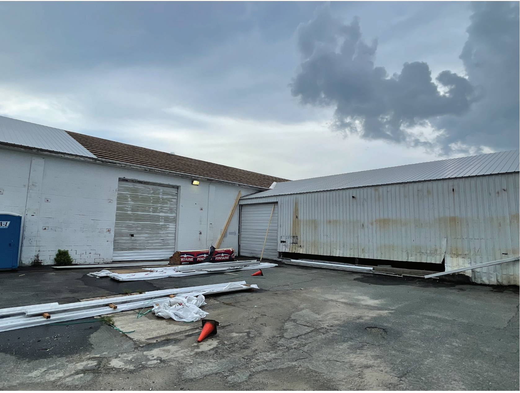
[D] - BUILDINGS 4 & 5 - NW CORNER AT FUTURE MECHANICAL YARD
