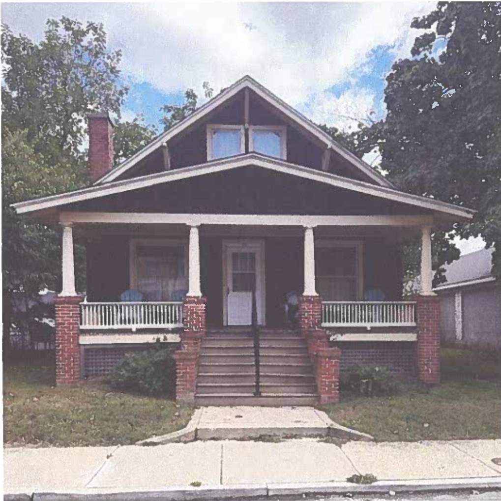
Front Street Facing Elevation
