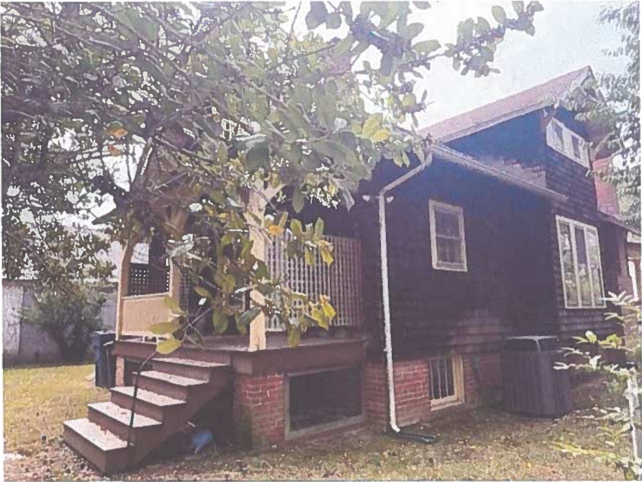
Left rear elevation and gutter type 2
