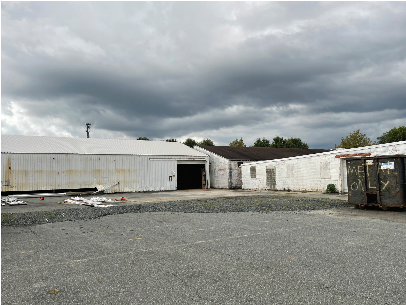
BUILDINGS 3 & 4 - EXISTING FACADE FROM NORTHWEST - PRIOR TO RENOVATION
