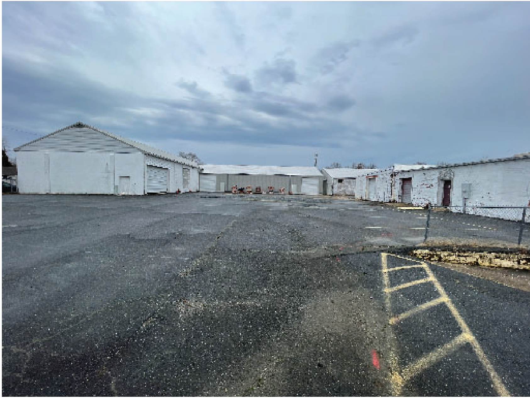
[C] - BUILDINGS 3,4 & 5 - FUTURE PARKING AND MAIN ENTRY FROM NORTH AT DOVER ROAD
