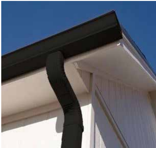
BLACK GUTTER AND DOWNSPOUTS
