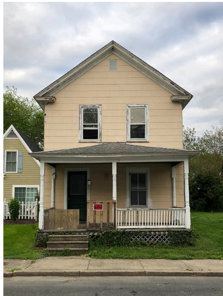
Existing West Elevation Photo
