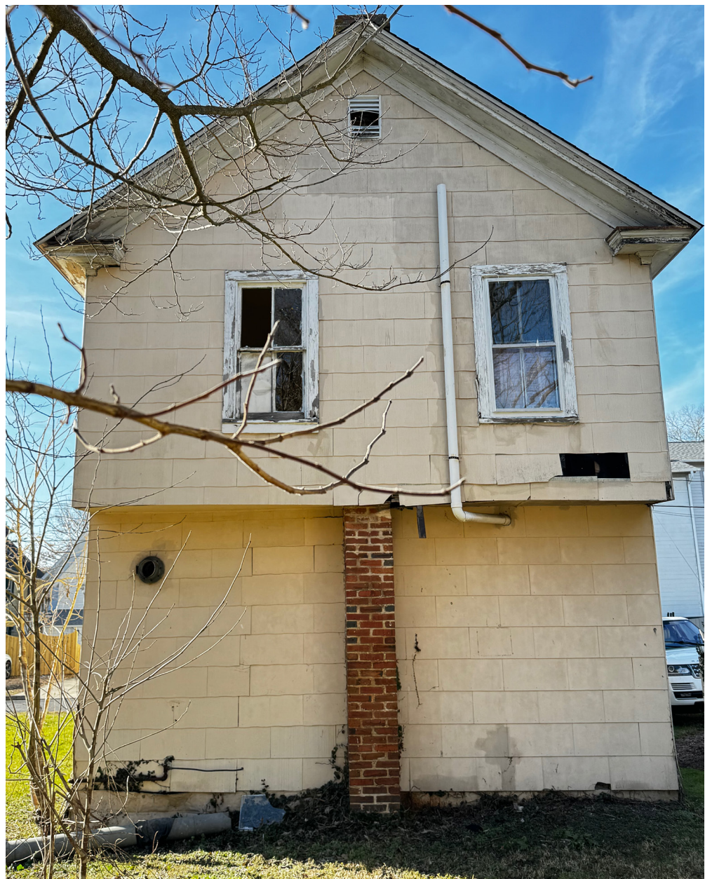
Existing East Elevation Photo
