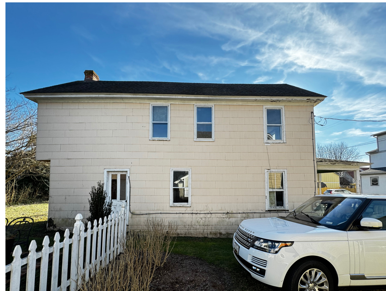
Existing North Elevation Photo
