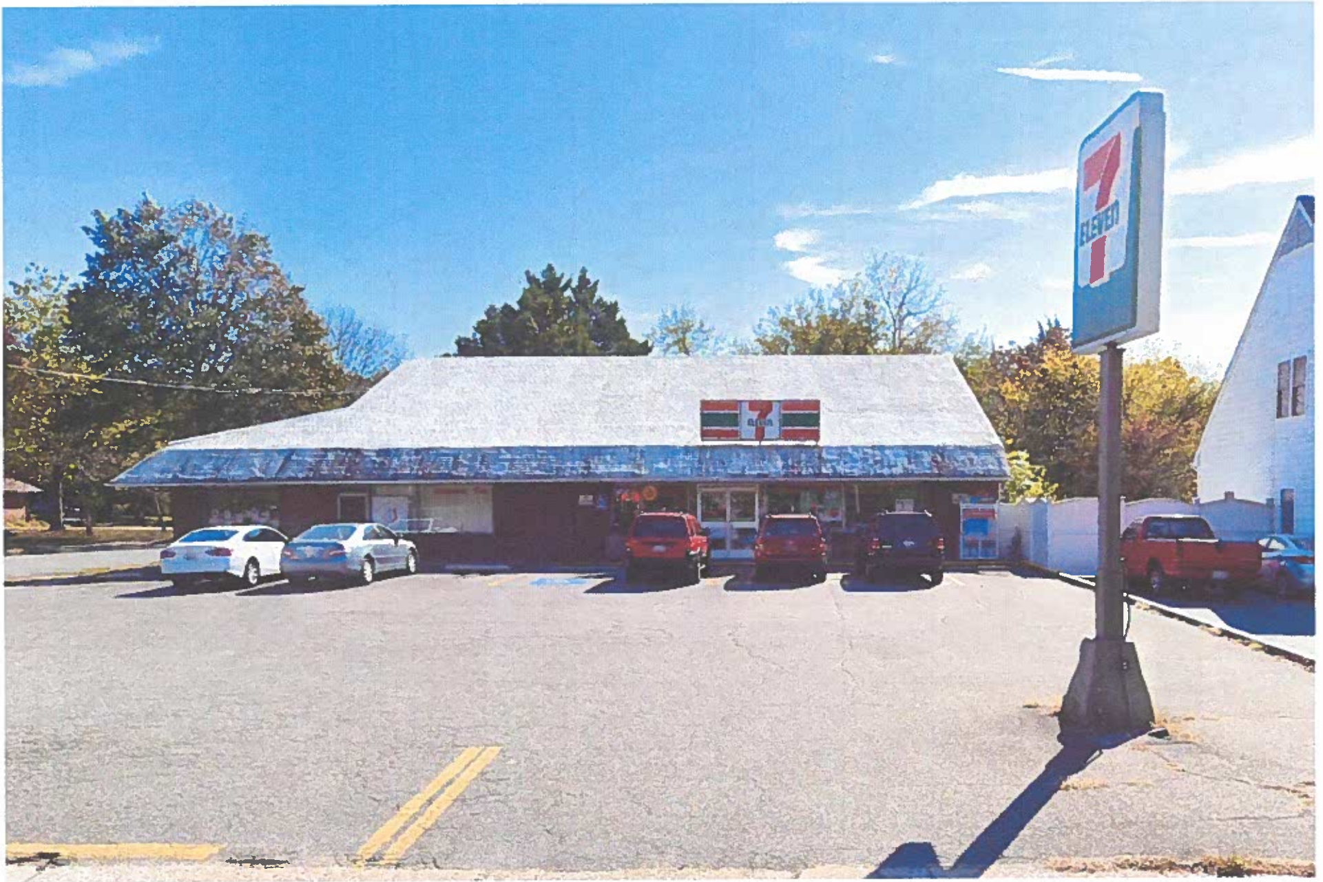
Sign before it was damaged
