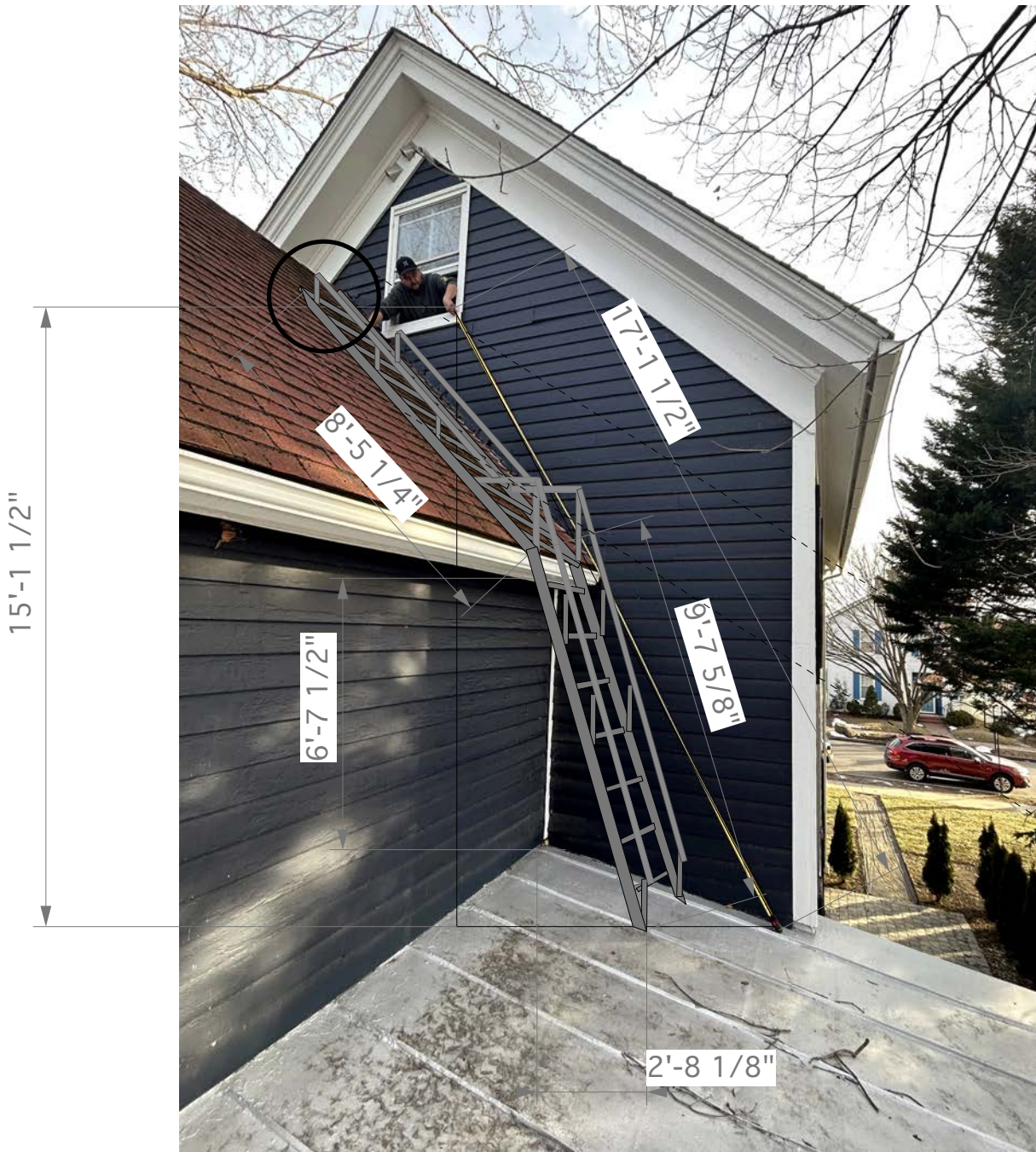
VIEW FROM FIRST FLOOR ATOP OF SHED ROOF Looking at second to thrid f bor access ladders
