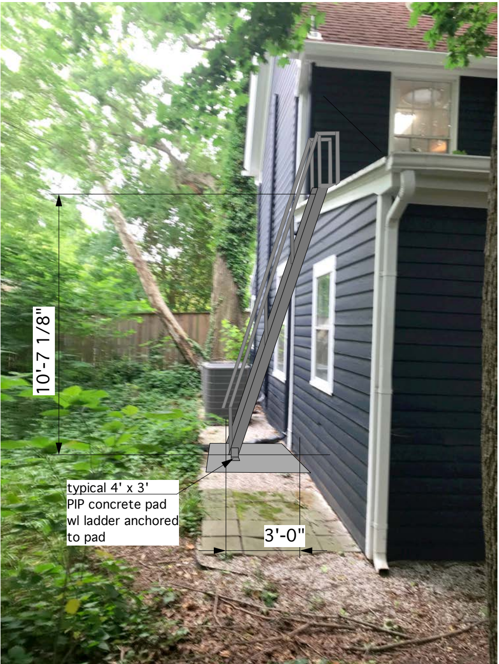
VIEW FROM GROUND Looking from ground level to first f bor roof access ladder
