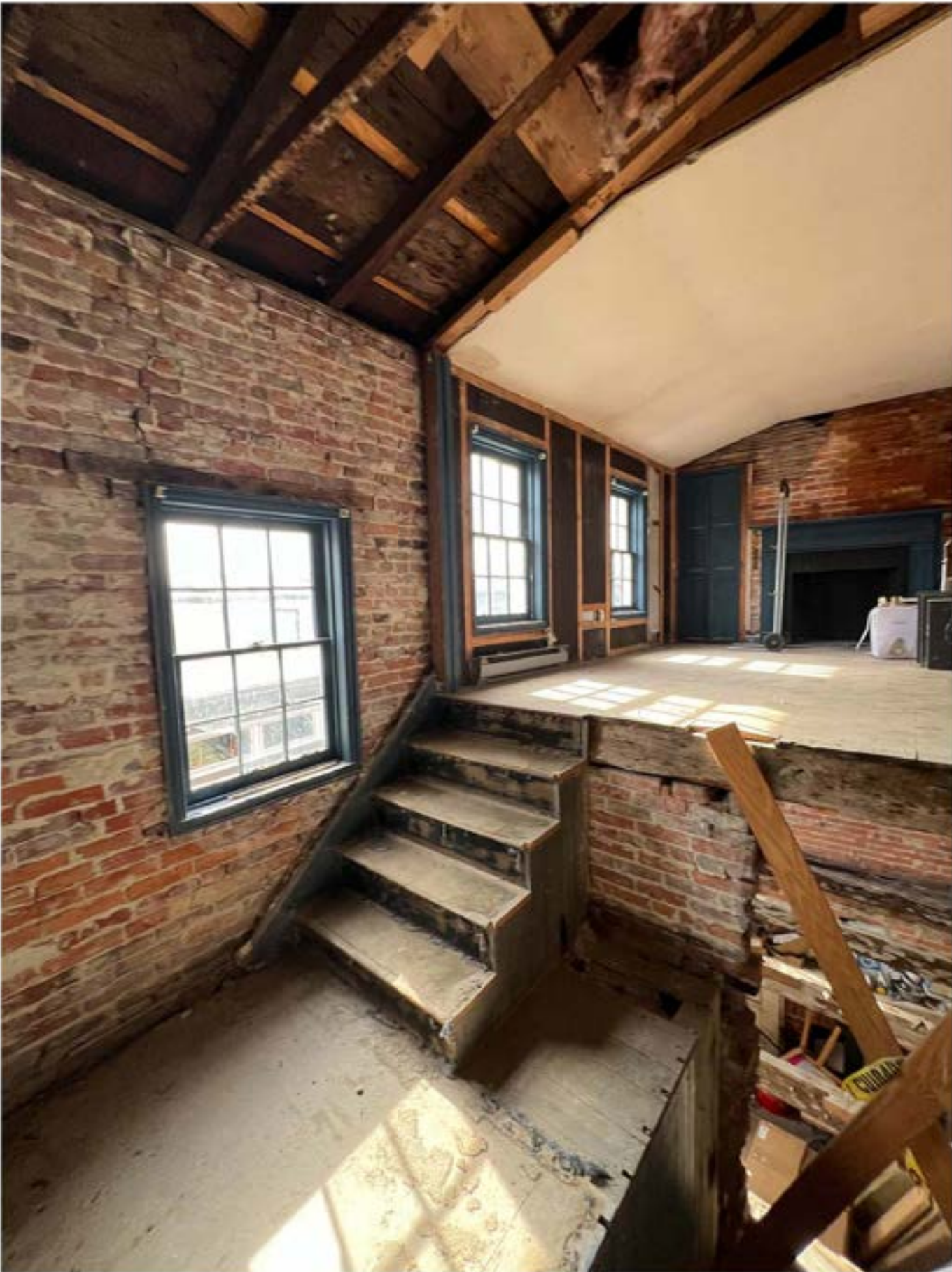
IP-3 VIEW STANDING ON LANDING LOOKING SOUTHWEST
