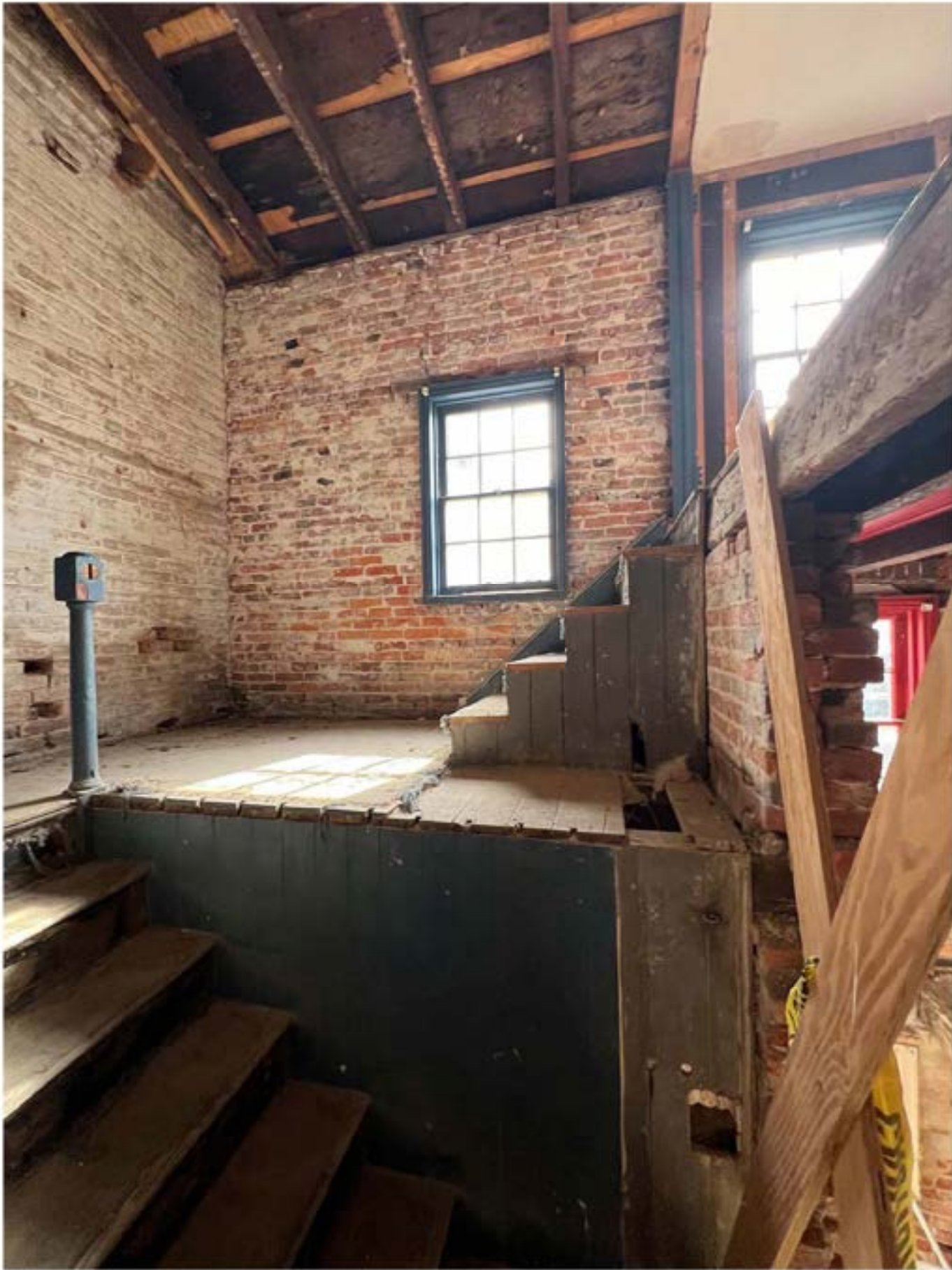
IP-2 VIEW STANDING ON LANDING LOOKING SOUTH
