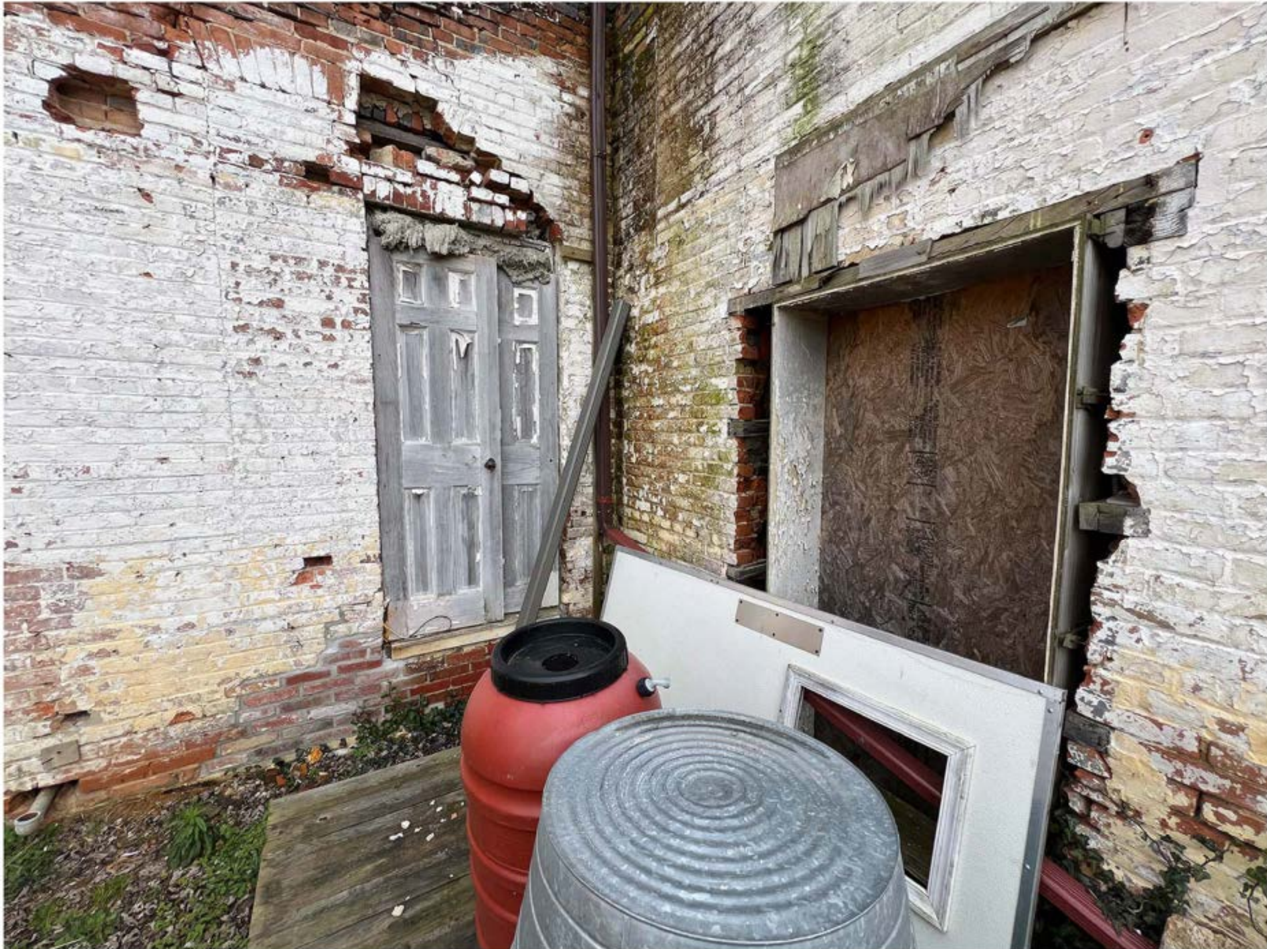
EP-4 VIEW LOOKING EAST, WEST ELEVATION
