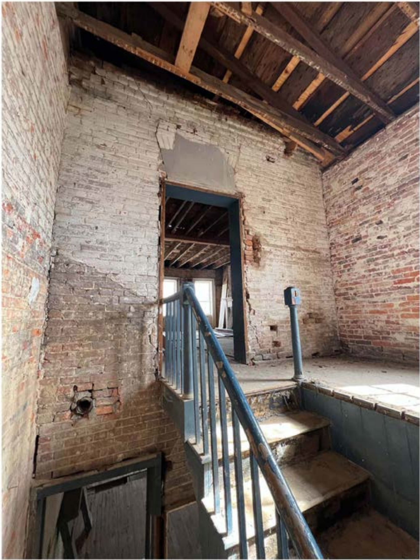
IP-1 VIEW STANDING ON LANDING LOOKING EAST
