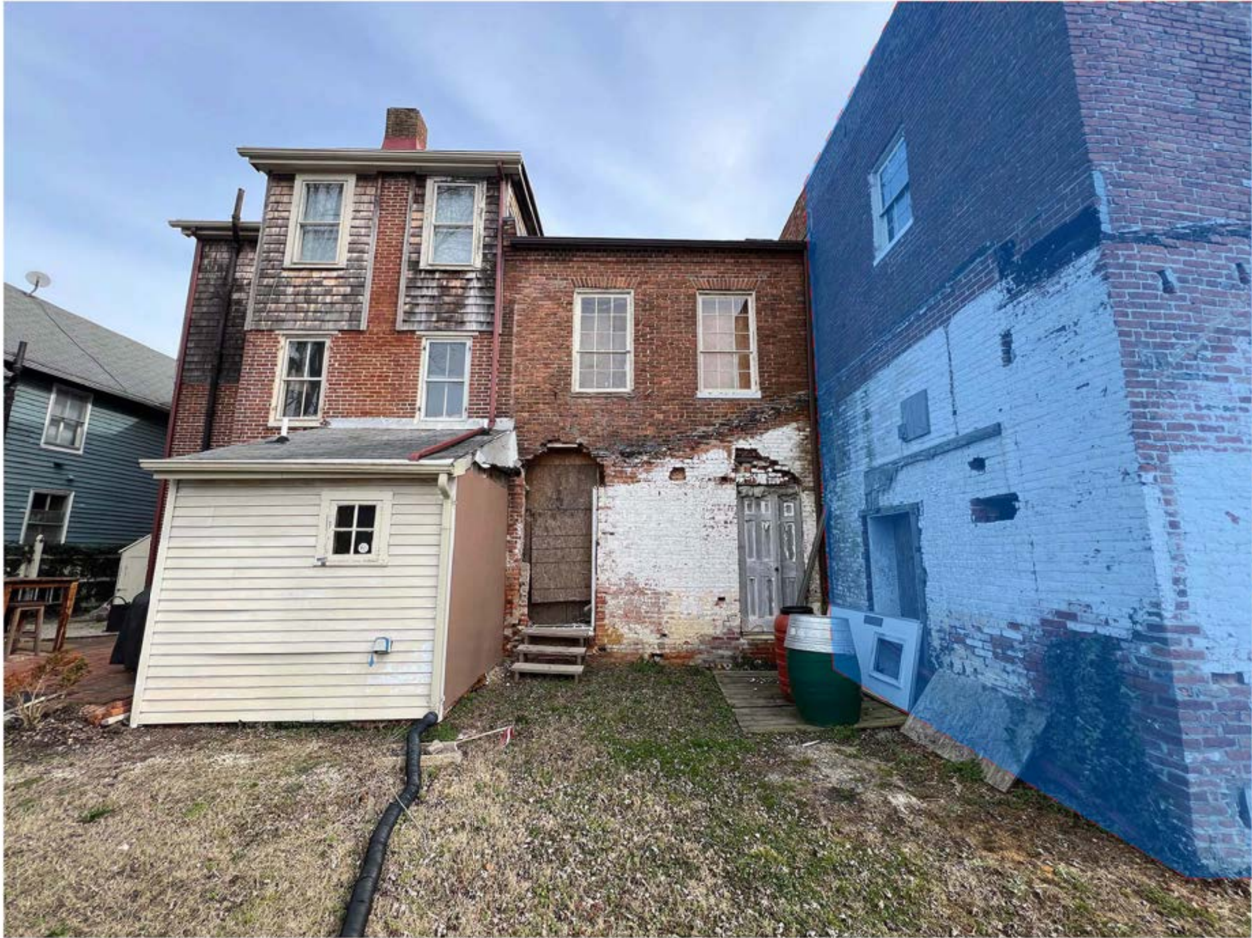
EP-1 VIEW LOOKING EAST, WEST ELEVATION
