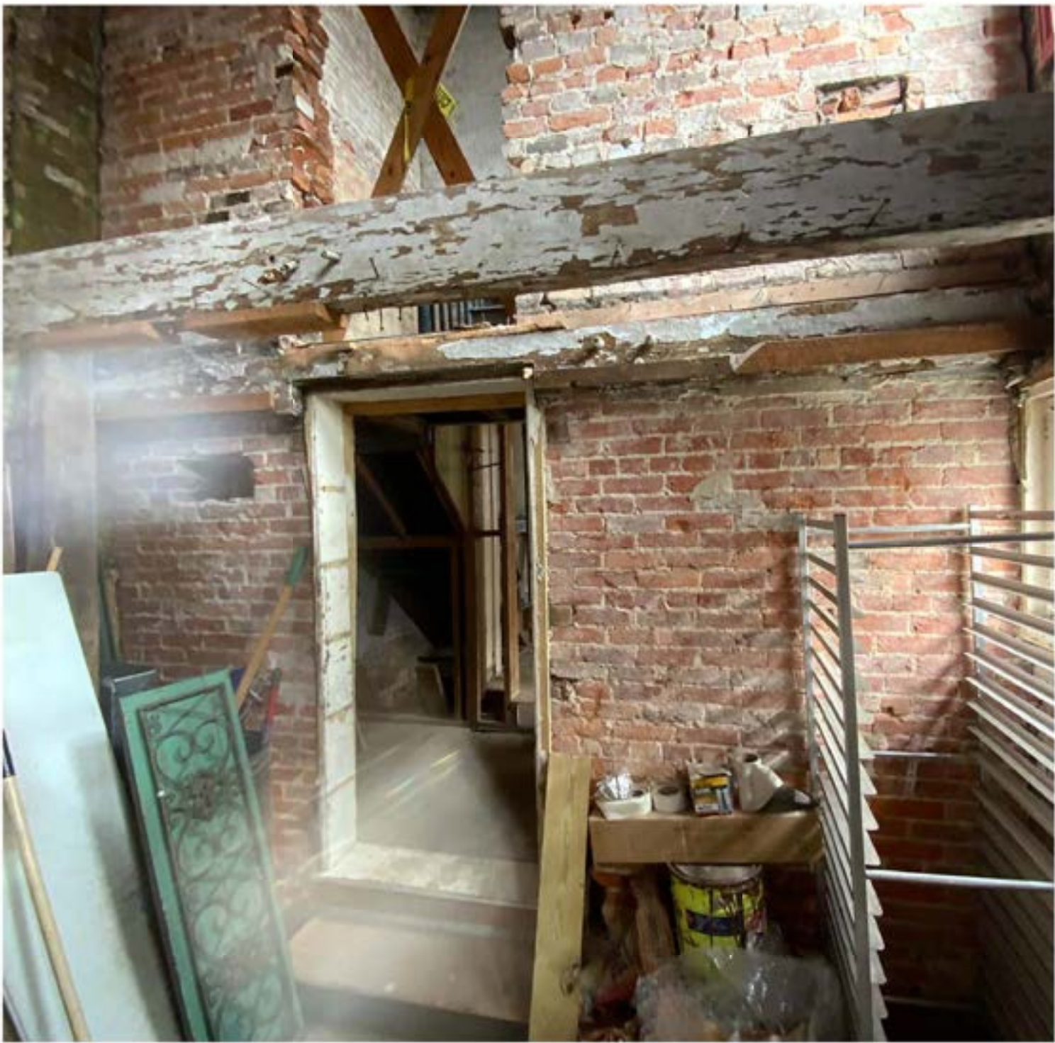
IP-5 VIEW AT ENTRY FLOOR LOOKING EAST
