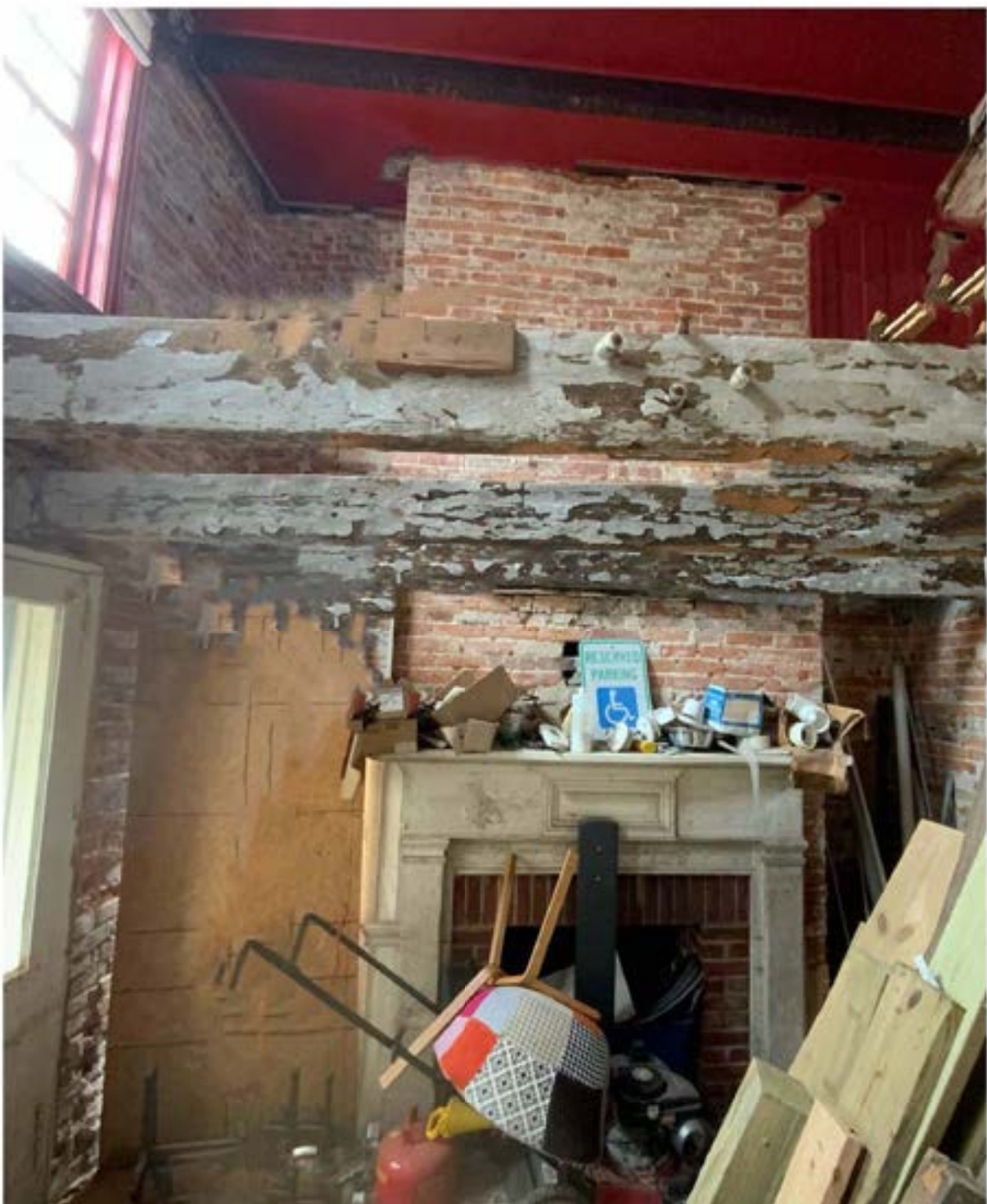
IP-7 VIEW AT ENTRY FLOOR LOOOKING WEST
