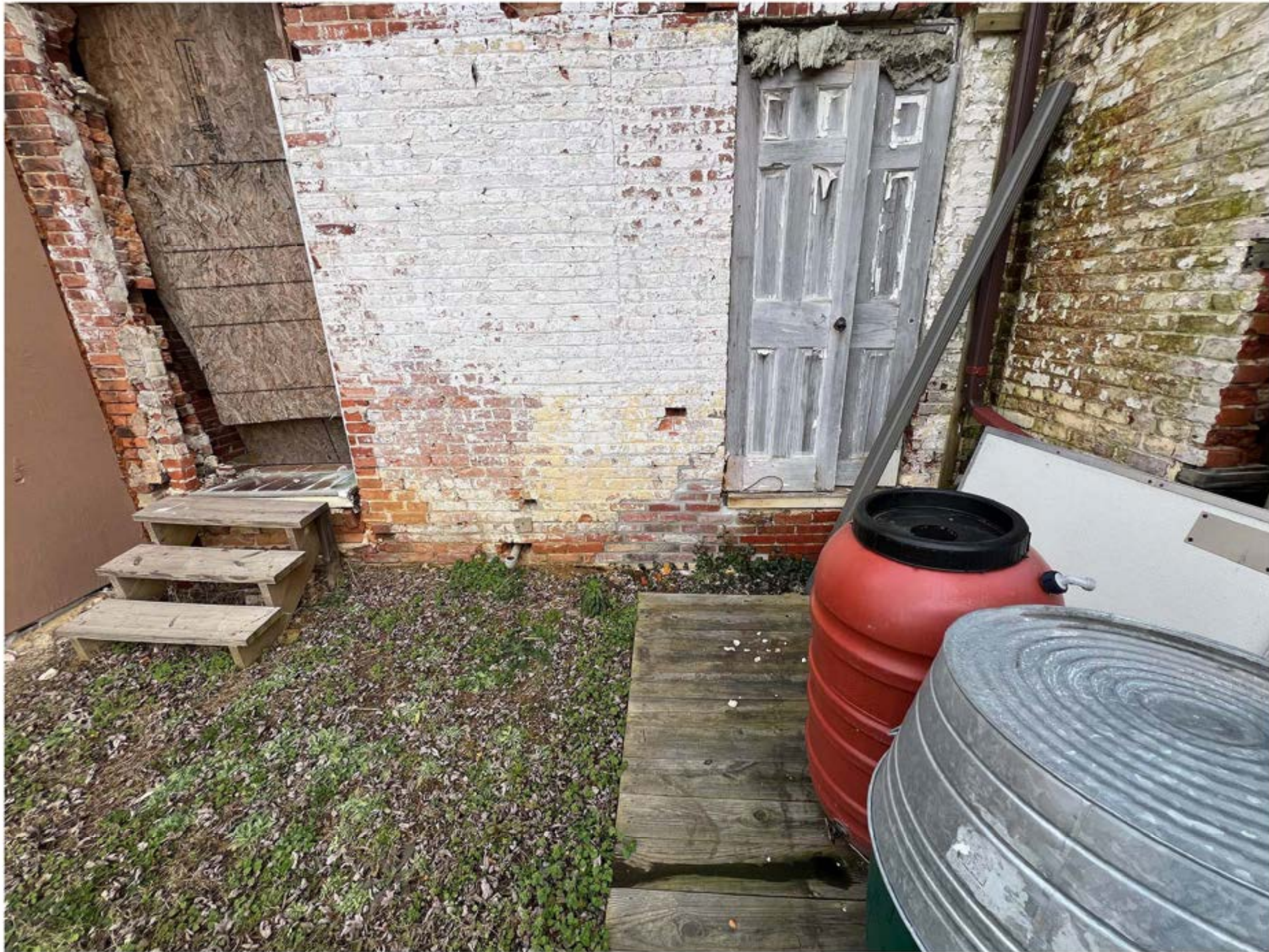
EP-3 VIEW LOOKING EAST, WEST ELEVATION
