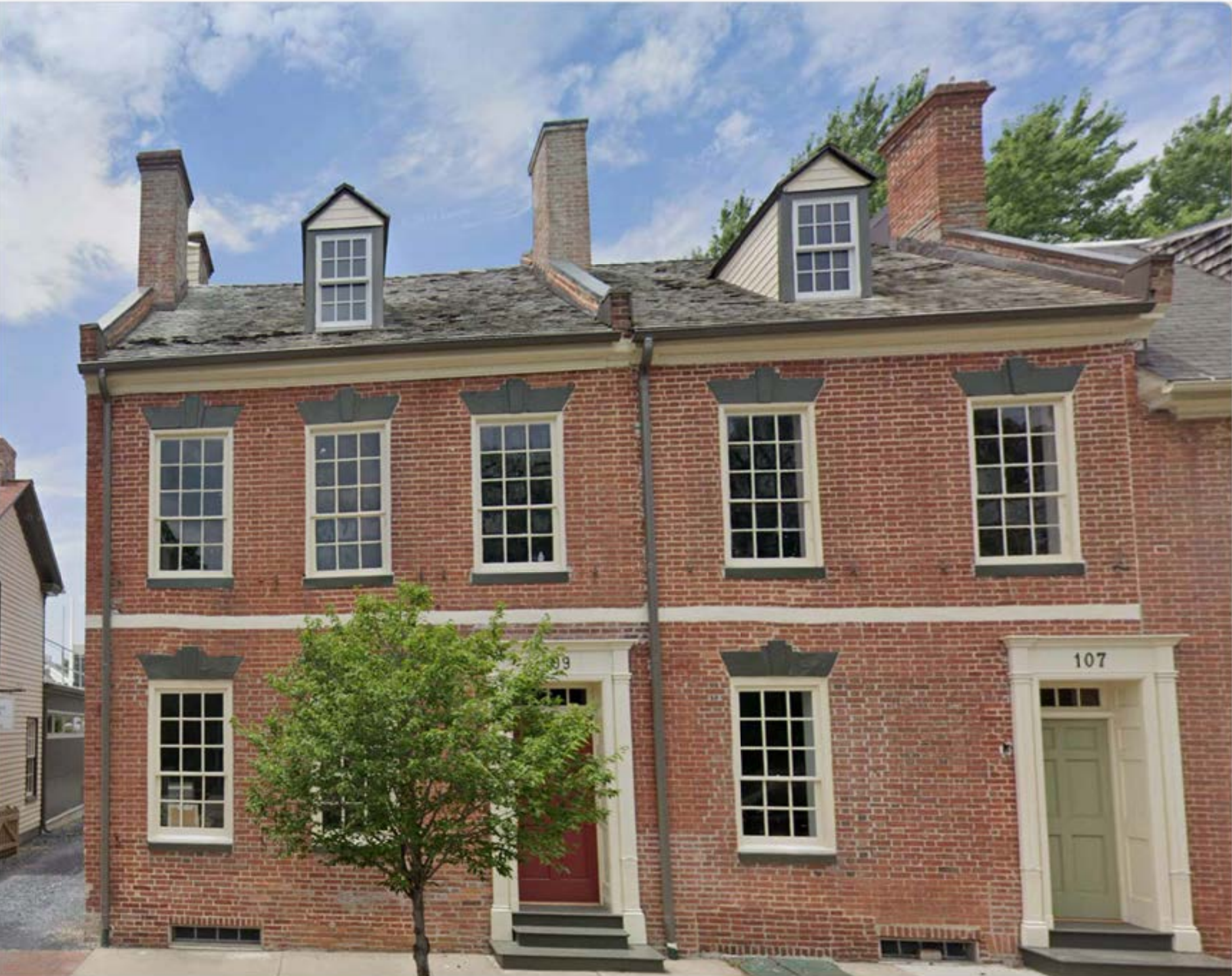
EP-8 VIEW LOOKING WEST, EAST ELEVATION
