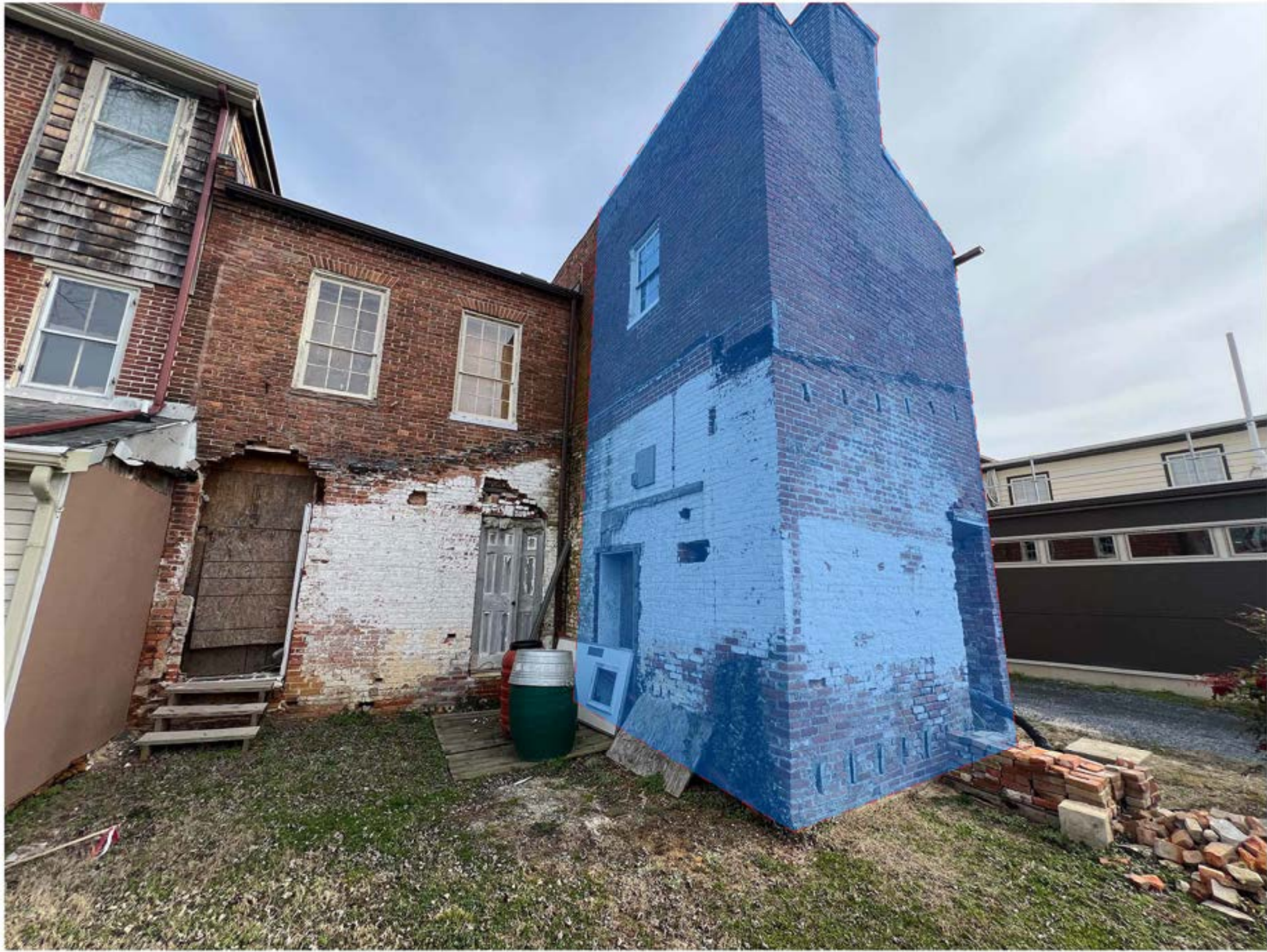
EP-2 VIEW LOOKING EAST, WEST ELVATION
