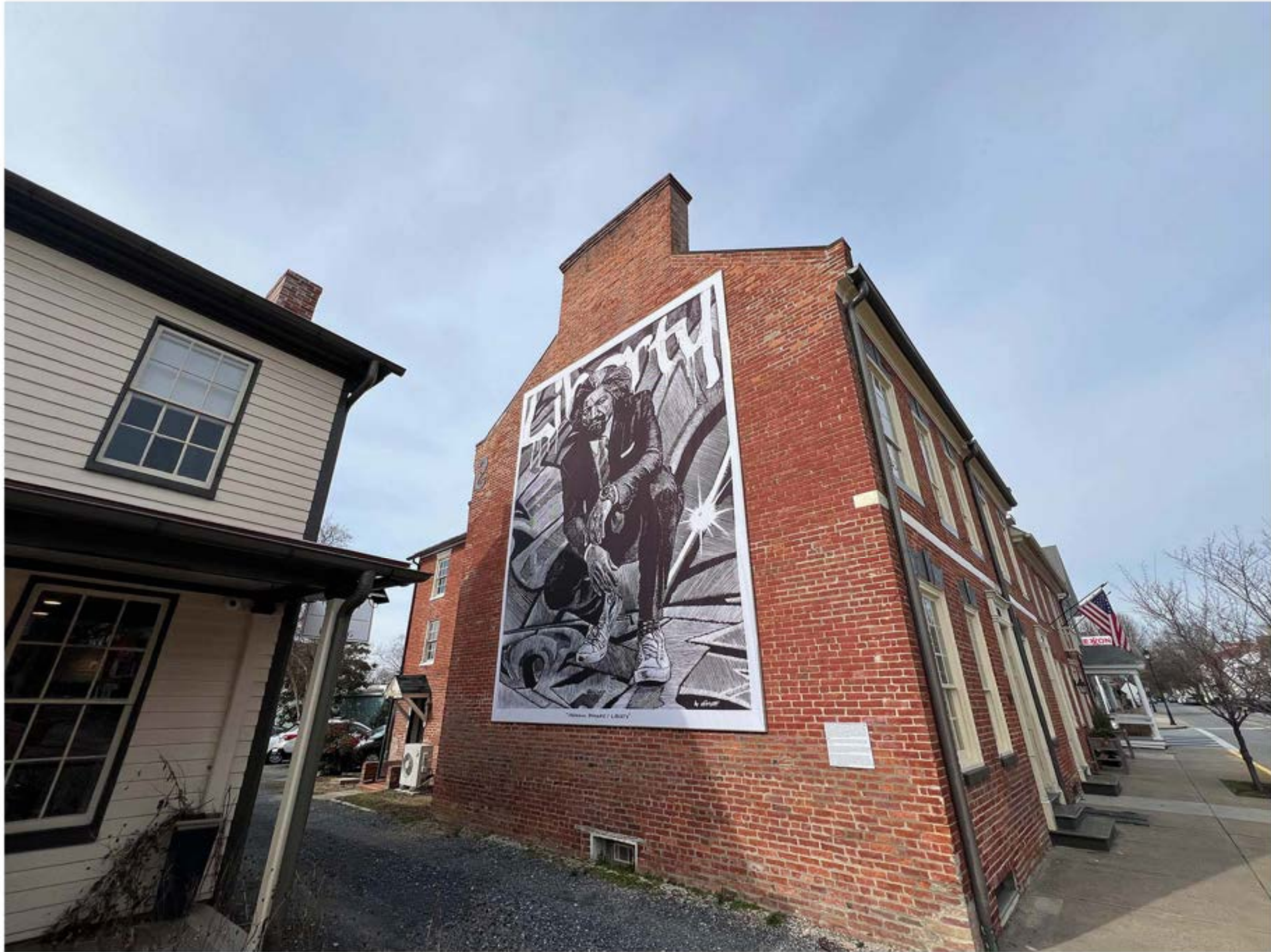
EP-7 VIEW LOOKING NORTHWEST,
