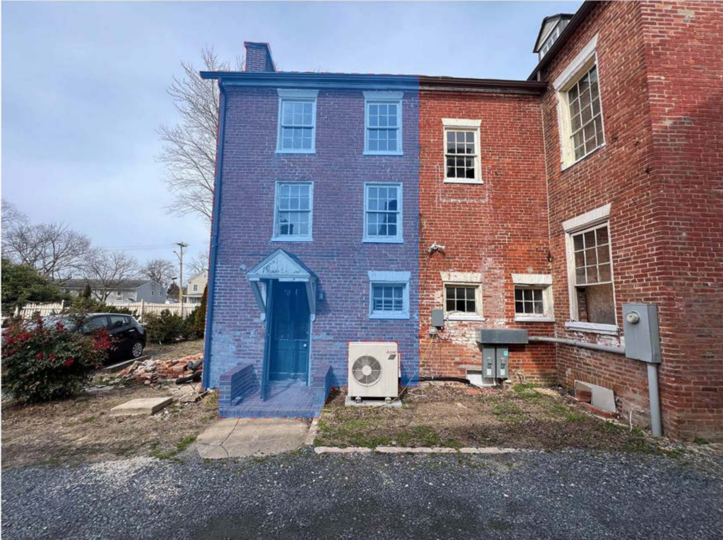
EP-6 VIEW LOOKING NORTH, SOUTH ELEVATION
