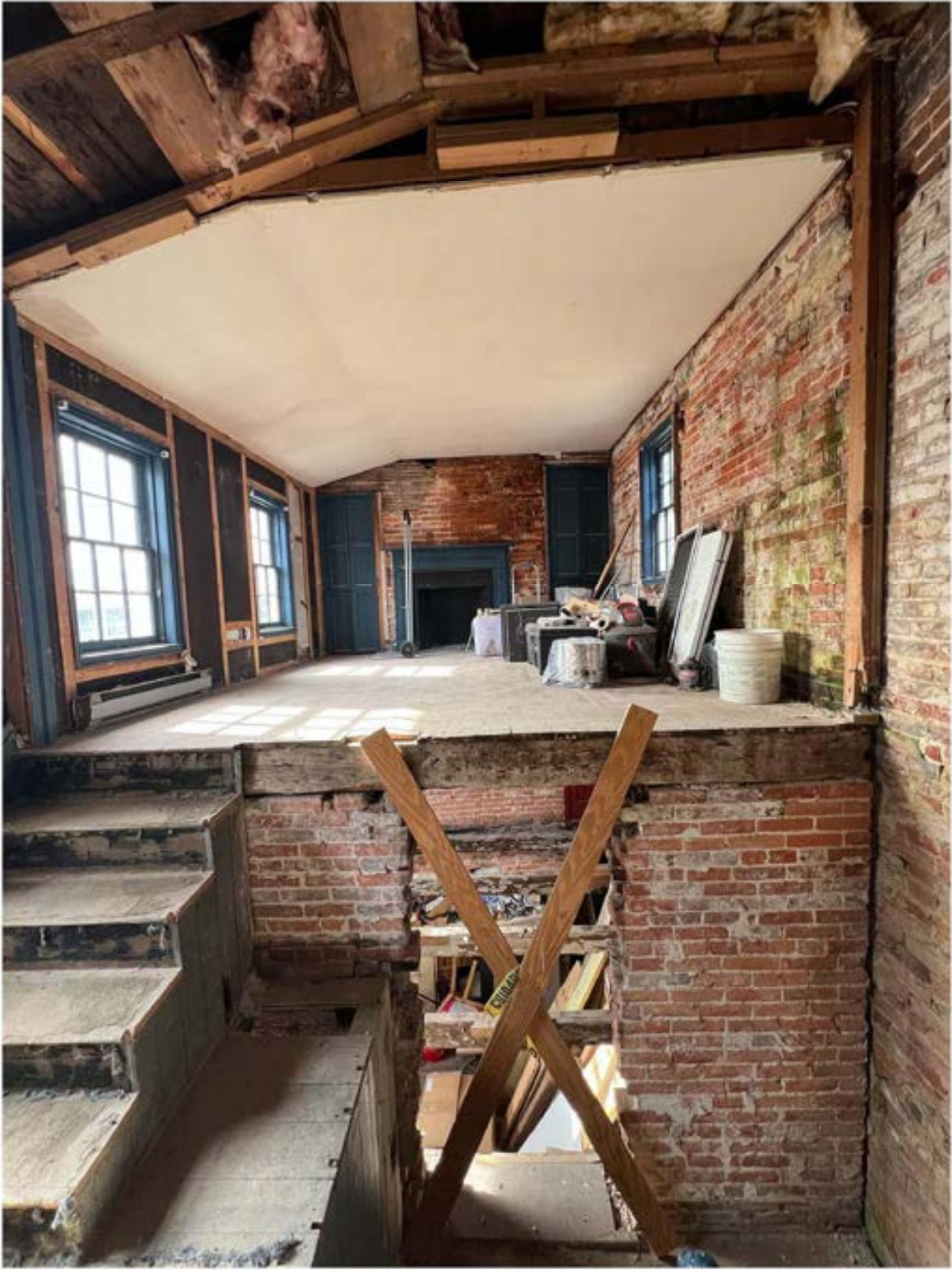
IP-4 VIEW STANDING ON LANDING LOOKING WEST
