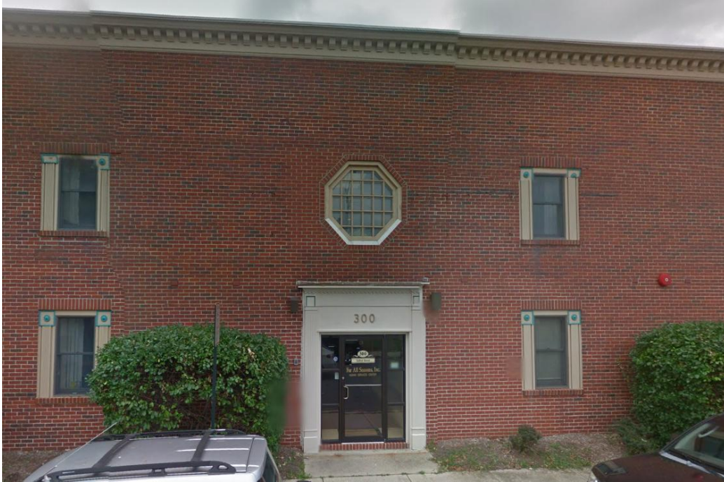
Talbot Street view – North Elevation
