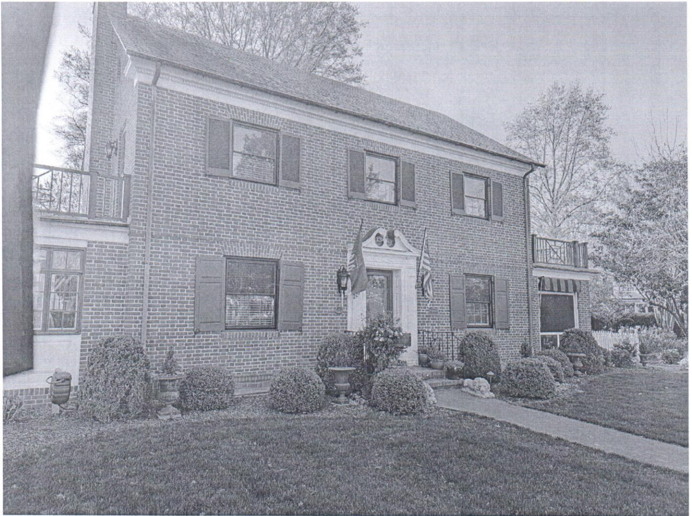
Existing Conditions Photo
