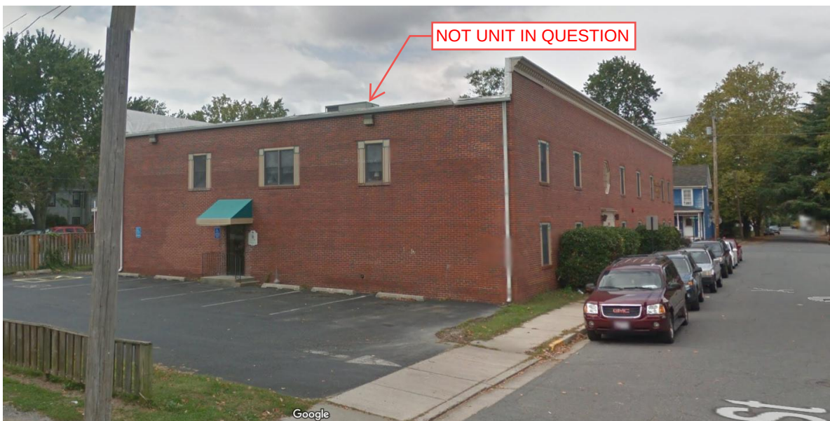
Talbot Street / parking lot view – Northeast elevation
