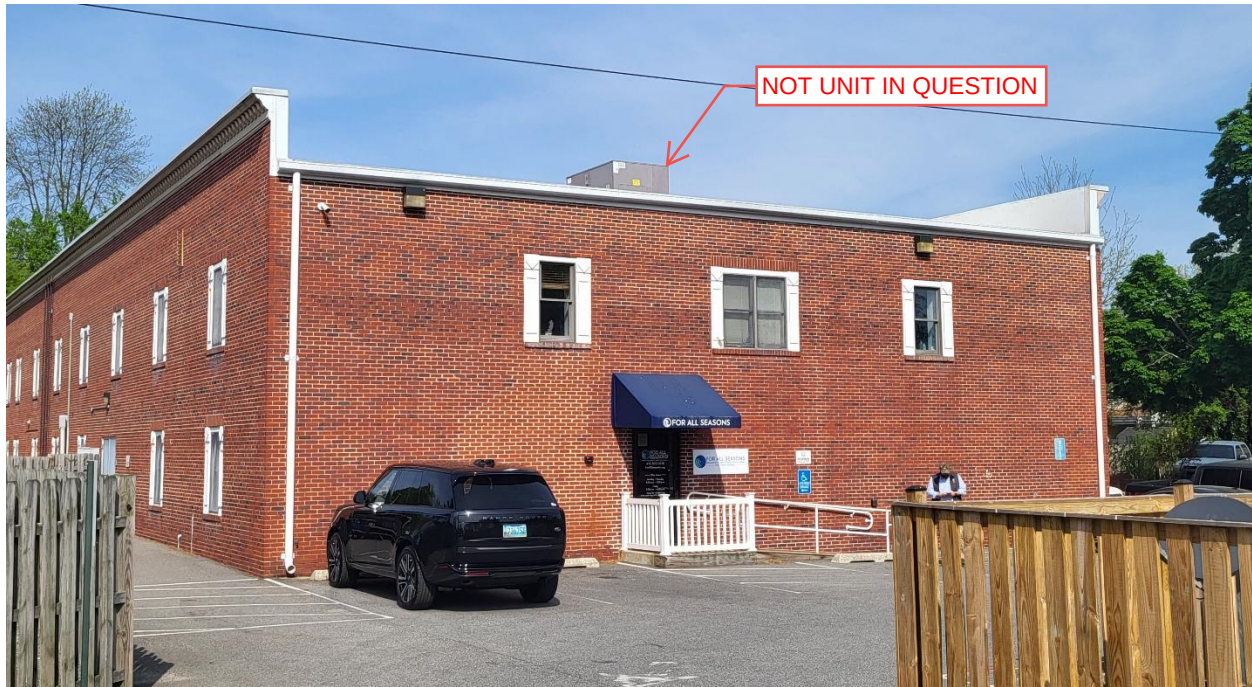
Parking lot view - Southeast elevation – HVAC units in question not visible
