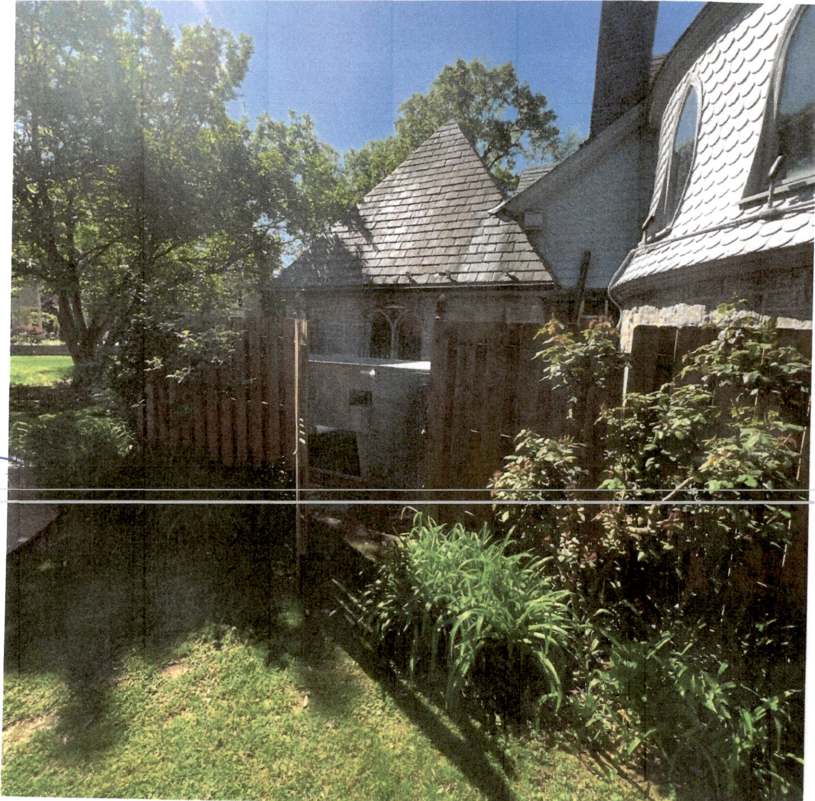
Existing Outdoor enclosure fence for Condenser
