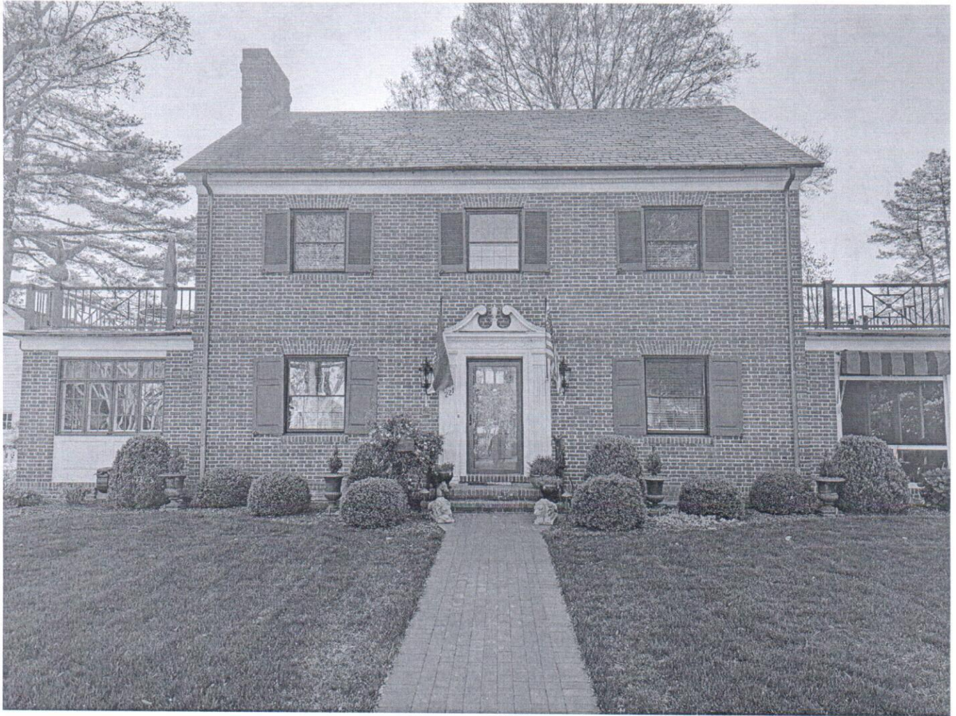
Existing Conditions Photo
