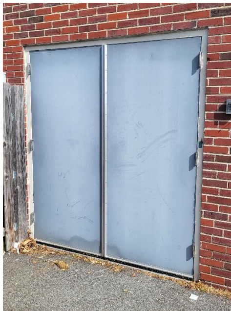
Utility exit – blocked from public view by fence
