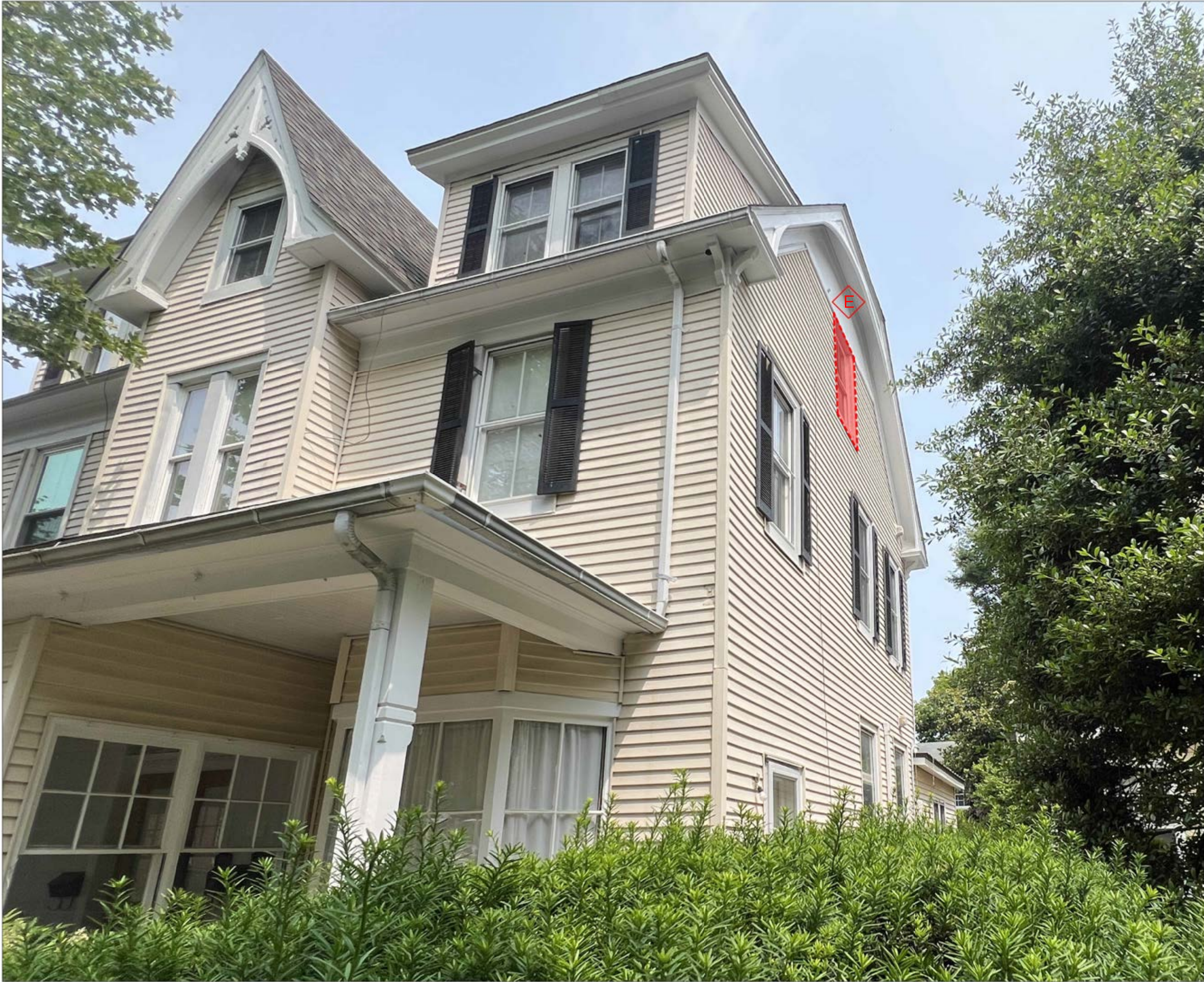
2 THIRD FLOOR WINDOW E
