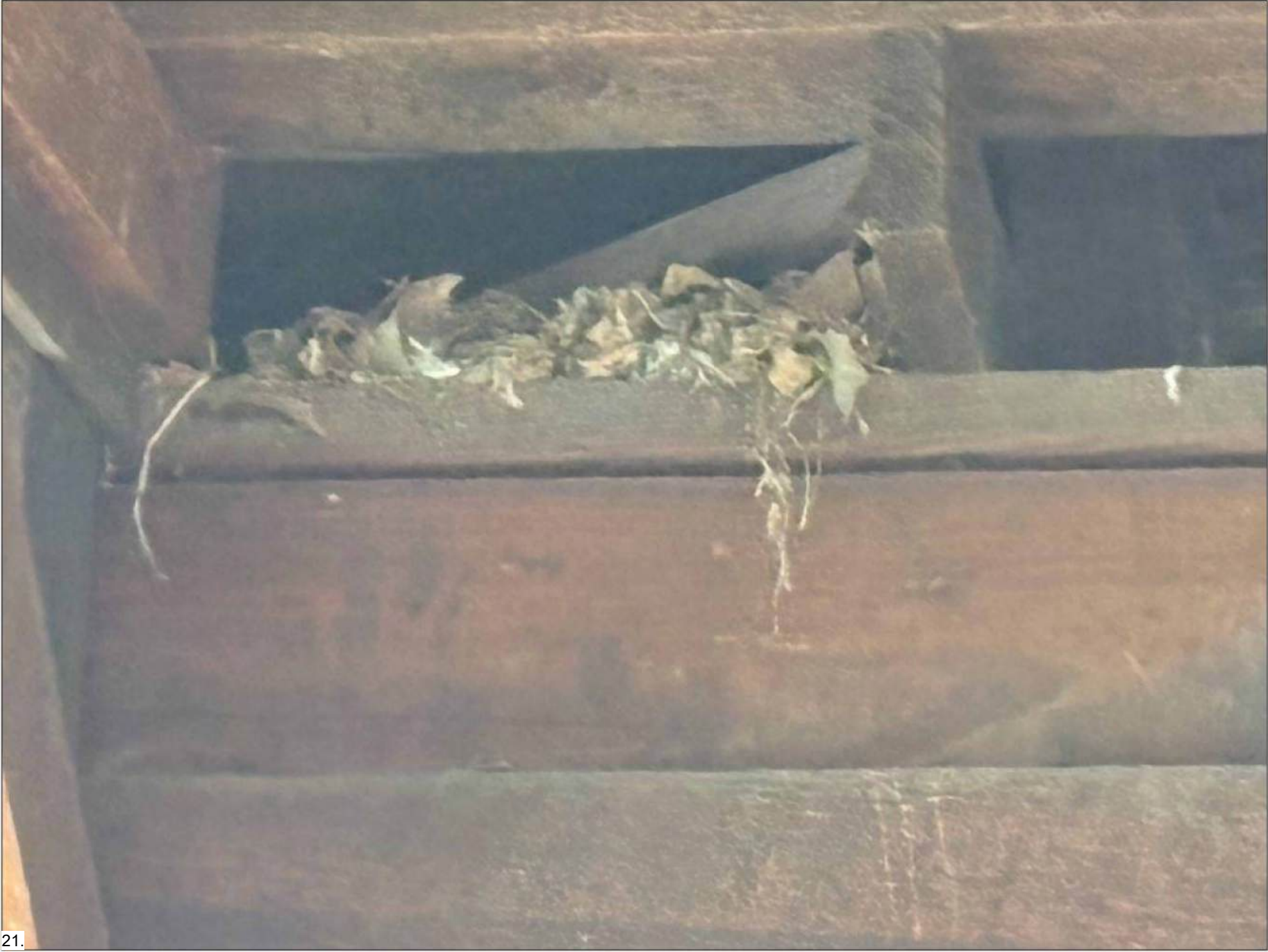
21. RAFTER TRUSS DETAIL AT BEARING ANIMALS NESTING
