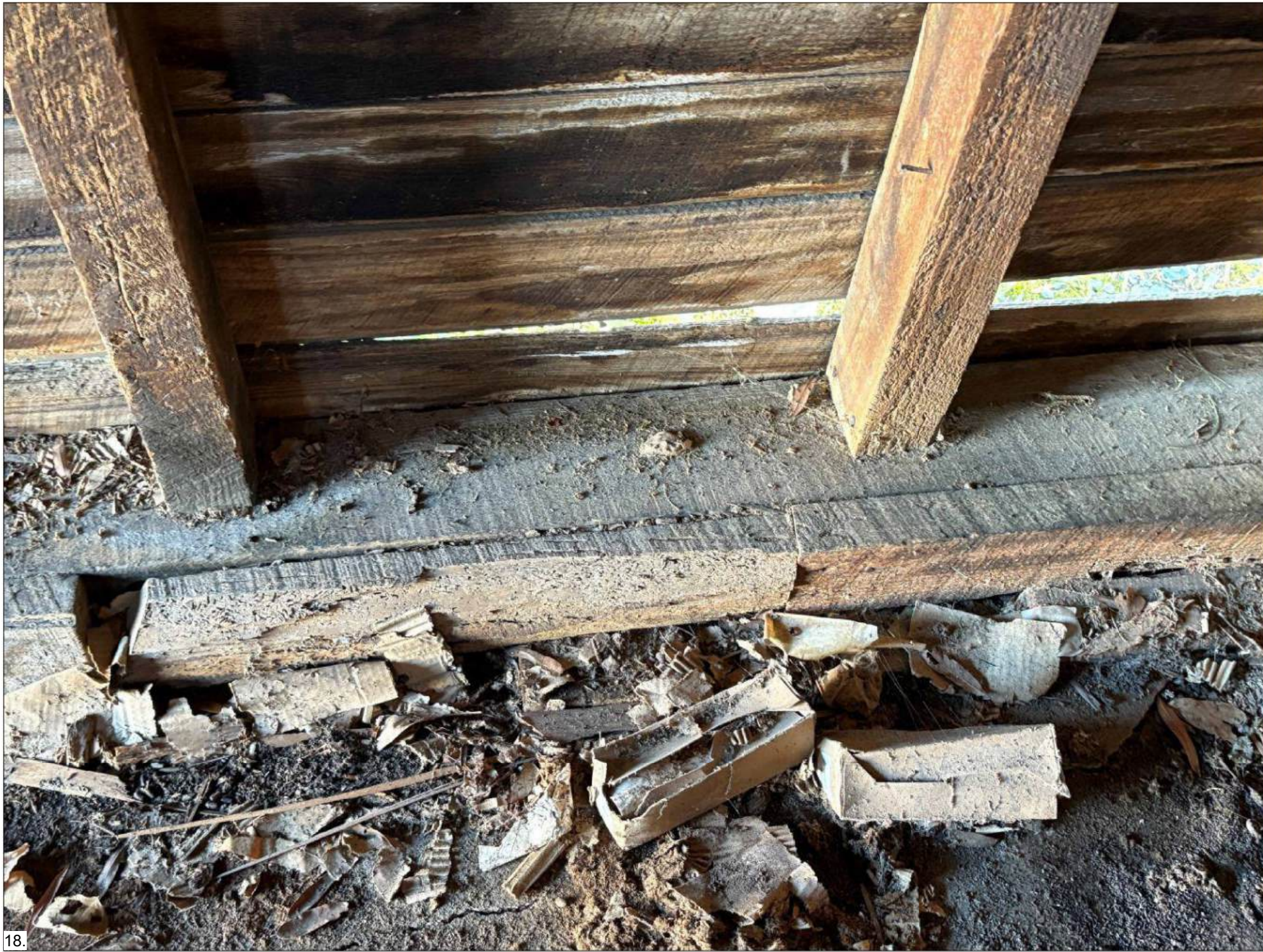
18. SILL PLATE DETAIL VOIDS IN SILL PLATE THAT HAVE BEEN PATCHED WITH WOOD BLOCKING, CONCRETE SLAB NEEDS TO BE REPLACED
