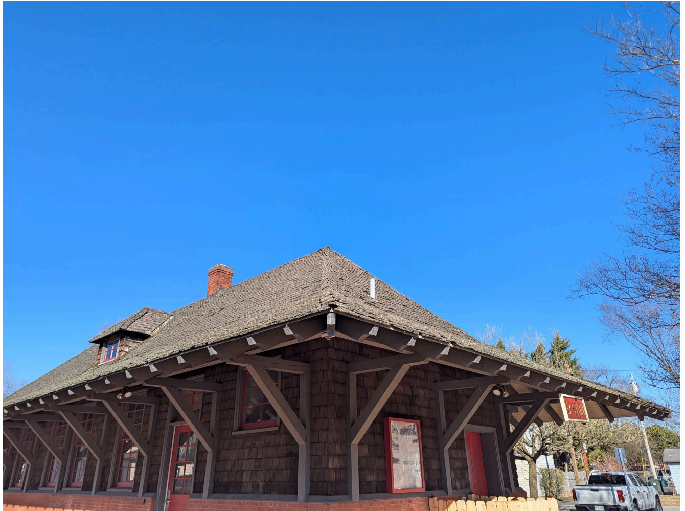
Example of Roof Support and Rafters of the Southwest Corner of the Station
