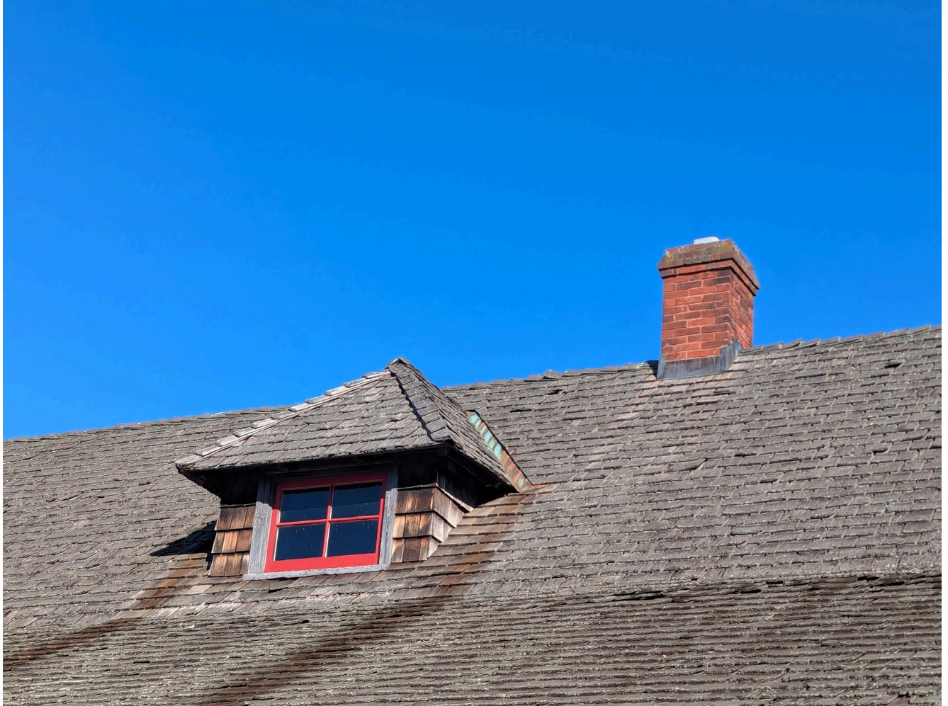
Dormer Located on Western Roof Face, Exposed Copper Valley Flashing and Chimney with Exposed Flashing
