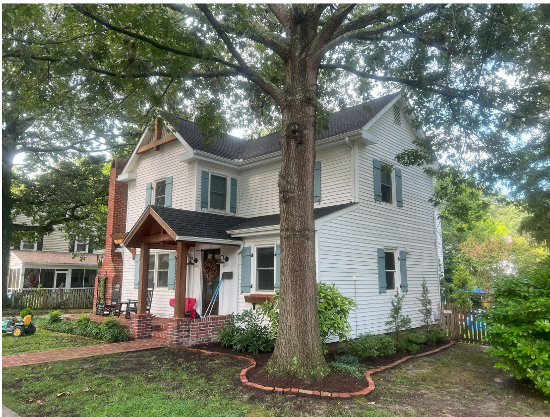
East (Street) and North Side
