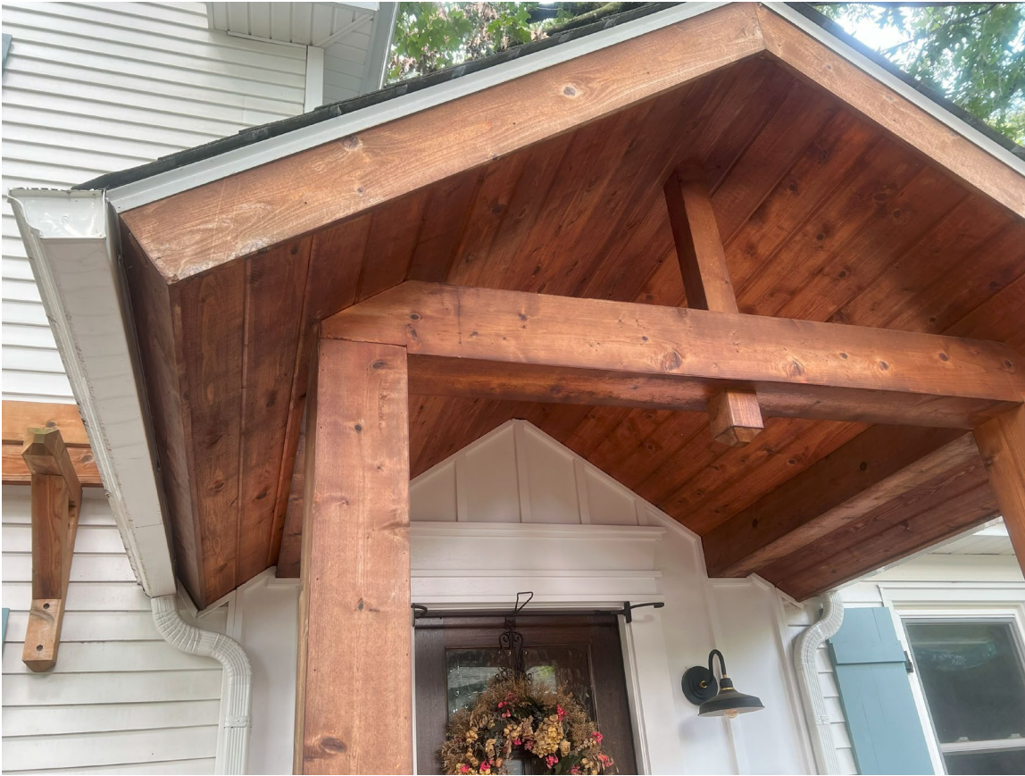
Front Porch Detail
