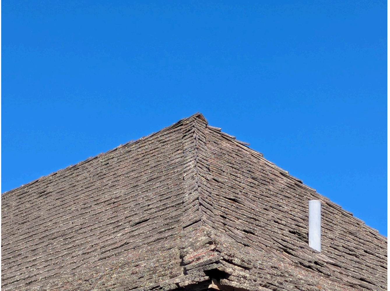
Example of Hip Ridge Condition of the Southwest Corner of the Station
