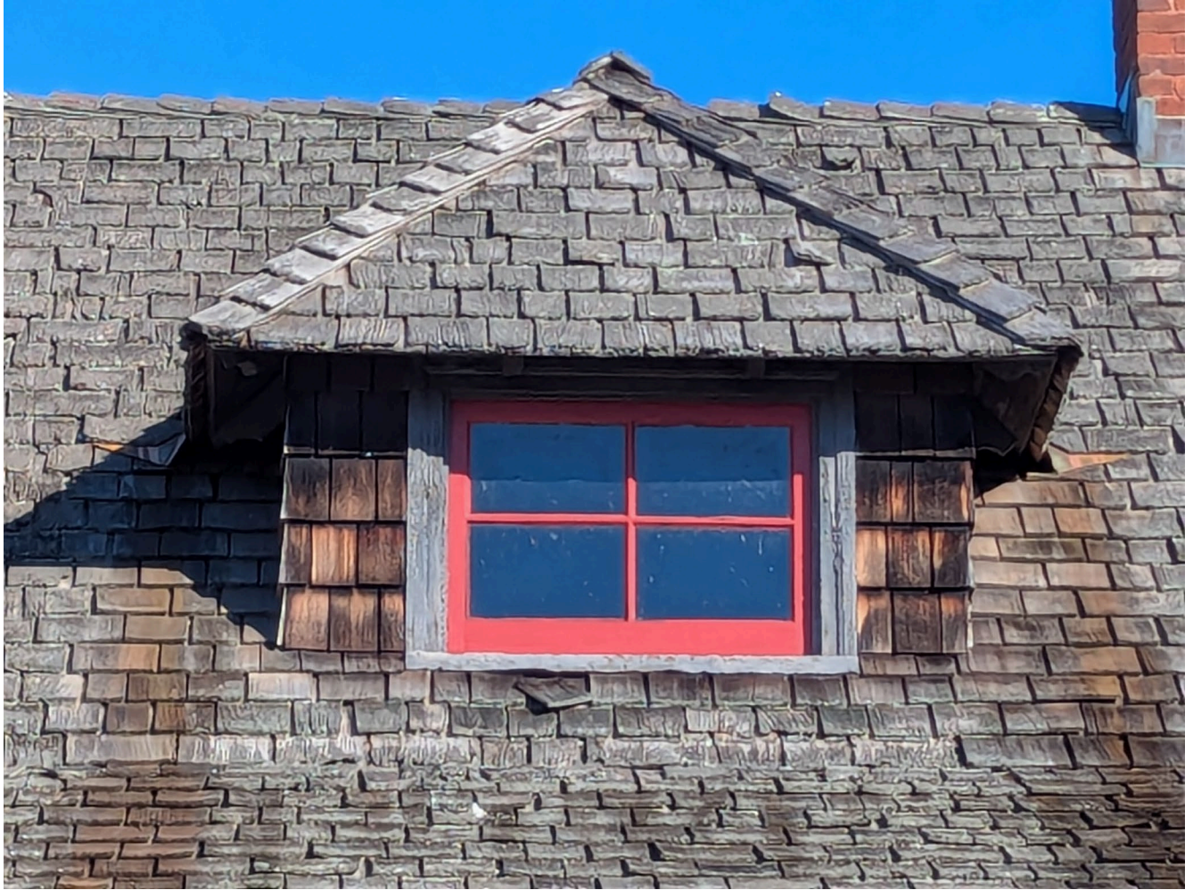
Dormer Located on Eastern Roof Face
