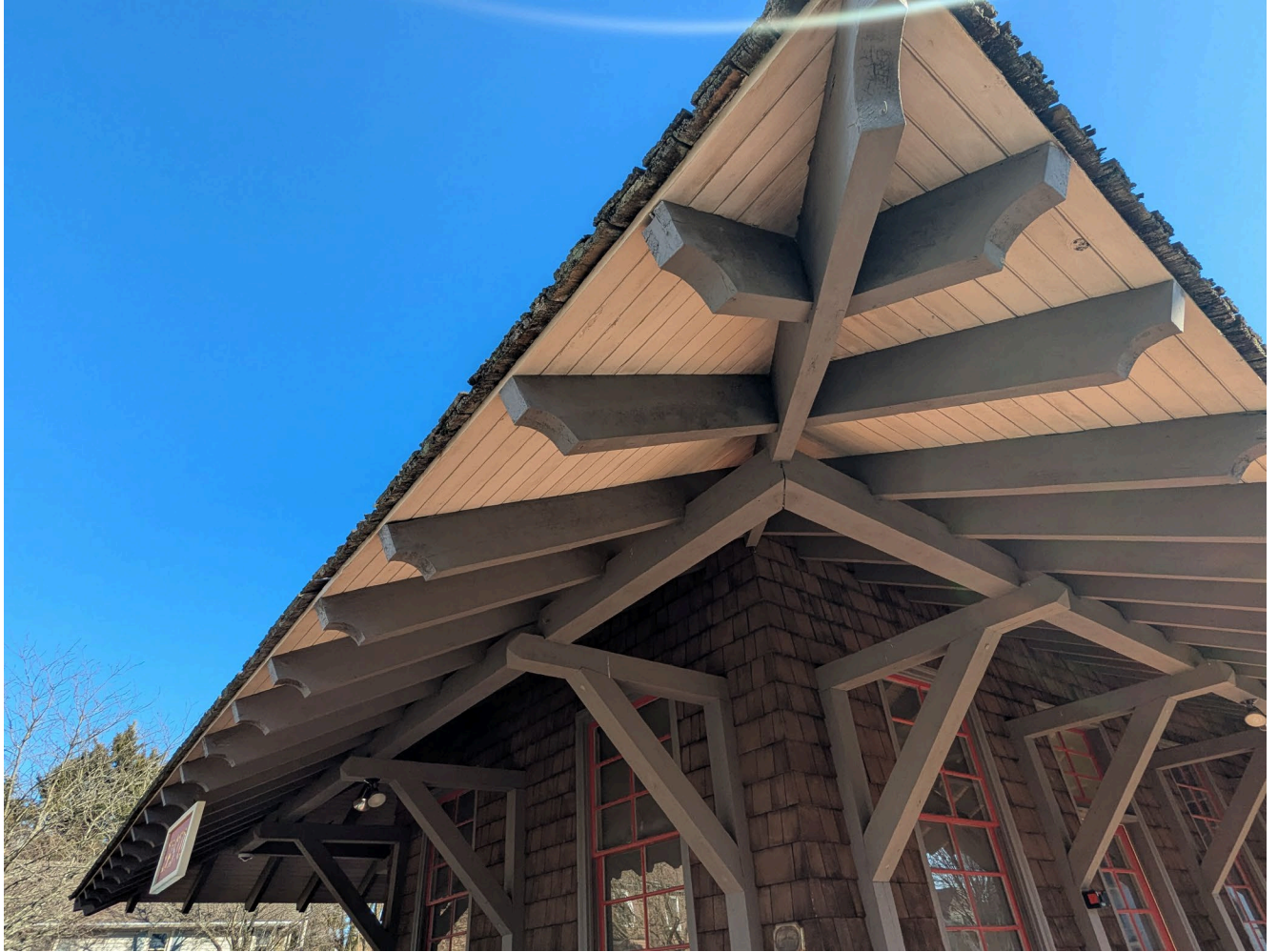
Example of Hip Rafters, Jack Rafters, and Tongue and Groove Roof Decking, Northwest Corner
