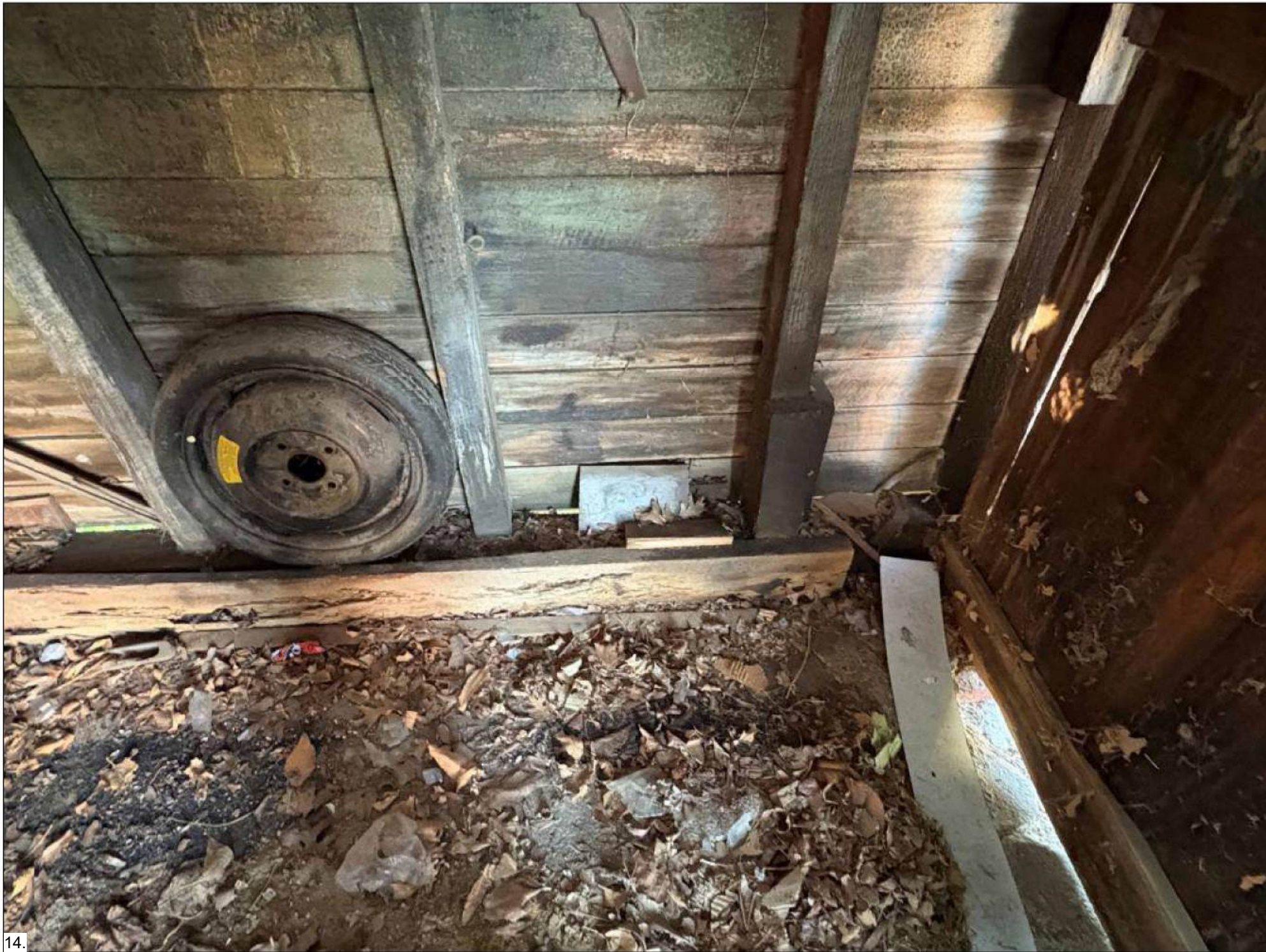
14. INTERIOR SOUTHWEST CORNER EXTENSIVE TERMITE DAMAGE AND ROT AT SILL PLATE, STUDS ARE LEANING
