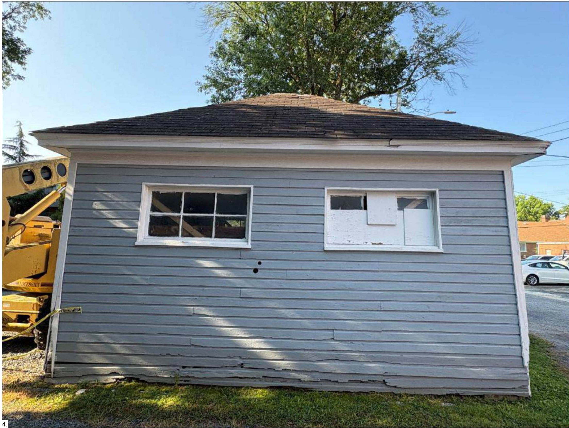
NORTH ELEVATION ROT AND TERMITE DAMAGE AT SILL, HOLES IN SIDING, WINDOW NEEDS REPLACEMENT. SOME WINDOWS ARE SALVAGEABLE BUT WILL REQUIRE NEW GLAZING AND MUNTIN WORK. ROOF SLATE NEEDS TO BE REPLACED.
