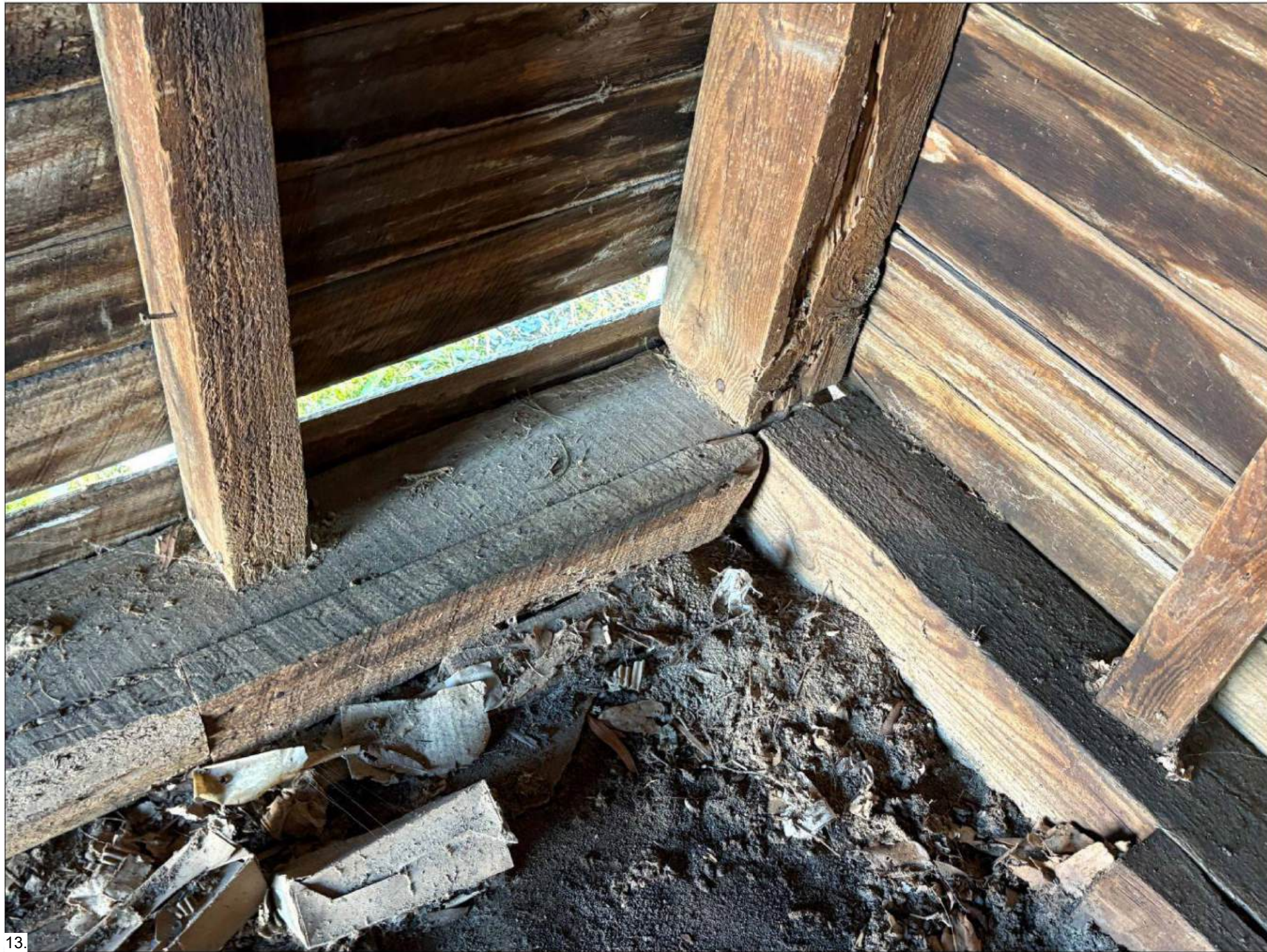
13. INTERIOR NORTHEAST CORNER TERMITE DAMAGE AT CORNER COLUMN AND STUDS, INTERIOR SIDING SHOWS MOLD AND WATER DAMAGE
