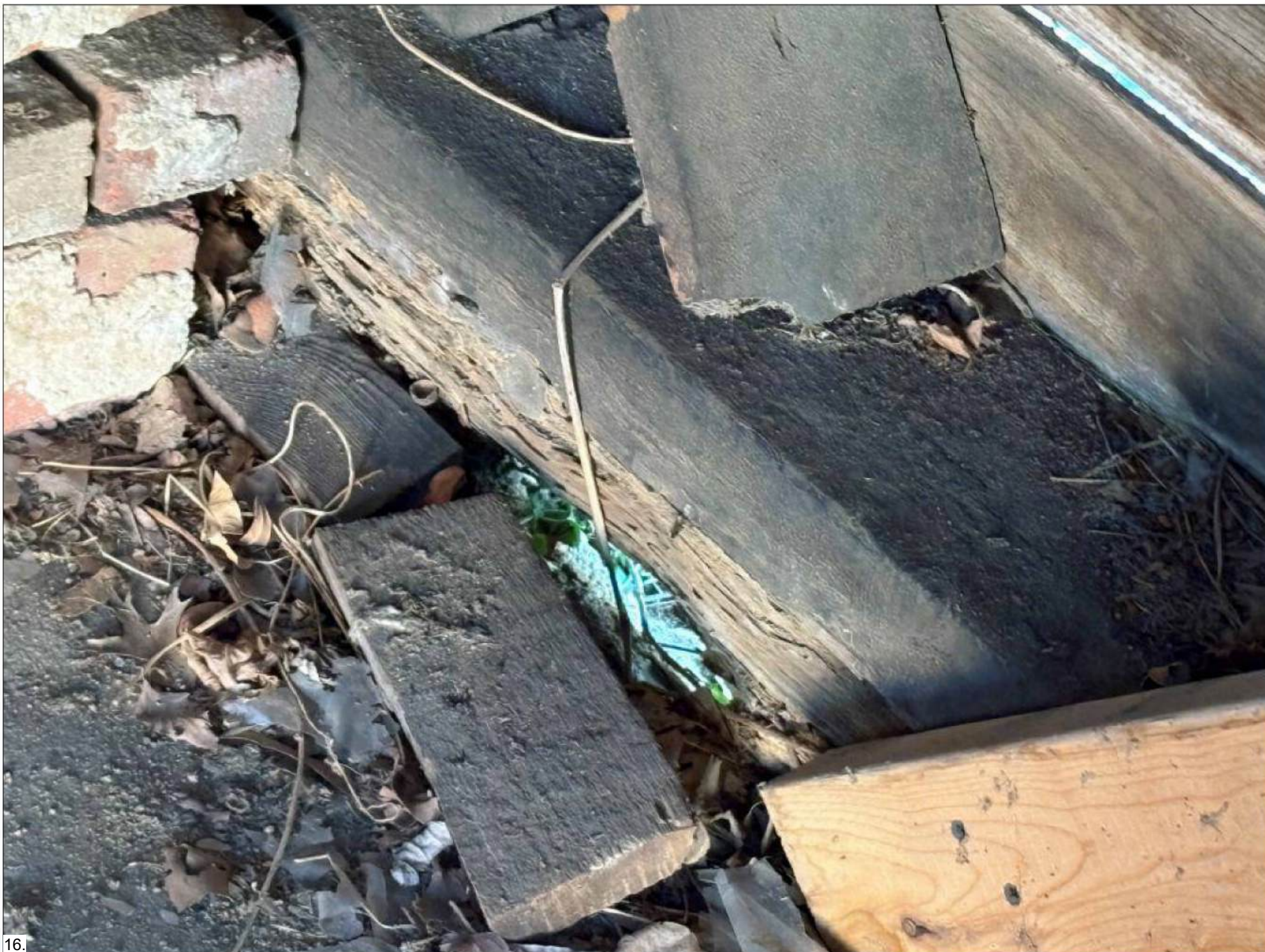
16. SILL PLATE DETAIL SEVERE TERMITE DAMAGE AND ROT CAUSING THE BUILDING TO LEAN
