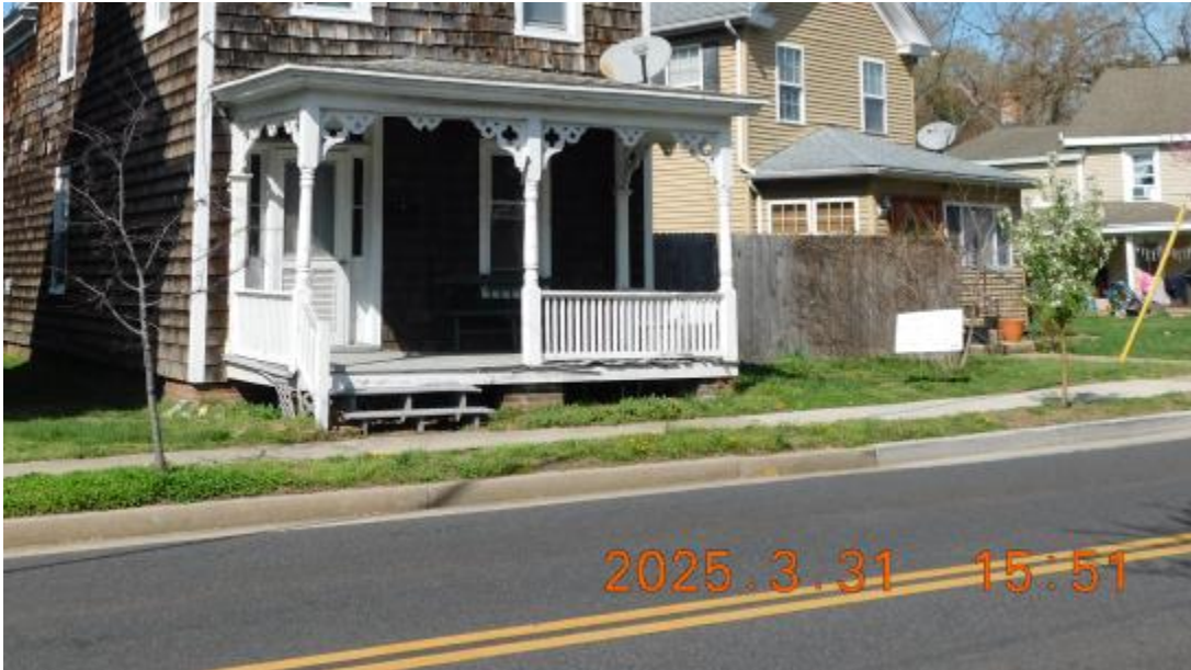
Figure 1 Front Porch Prior to Work Commencing
