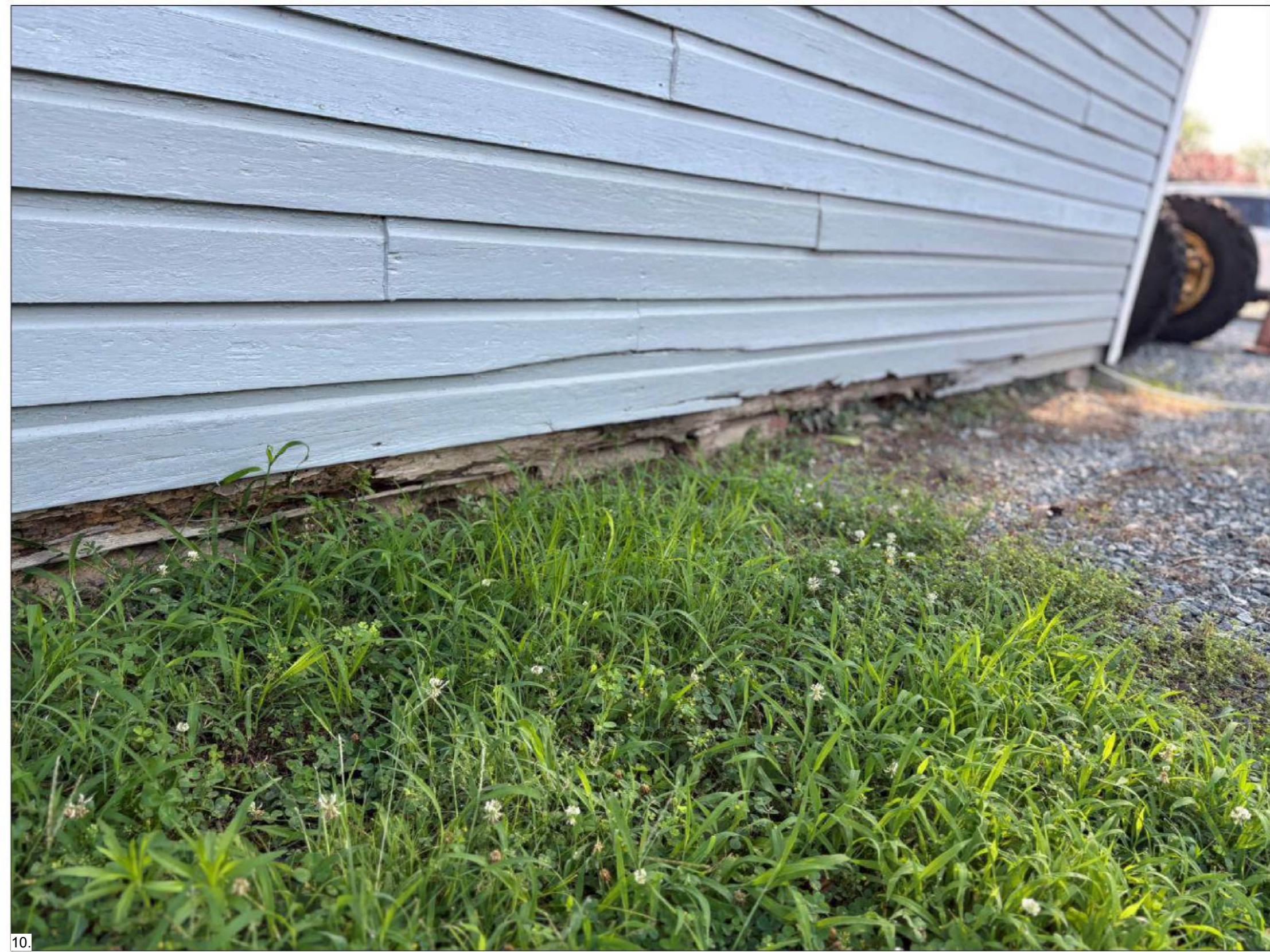
10 SOUTH SILL PLATE SEVERE TERMITE DAMAGE AND ROT CAUSING THE BUILDING TO LEAN, UNCLEAR ABOUT INTEGRITY OF FOUNDATION BUT INTERIOR SLAB HAS CRACKING
