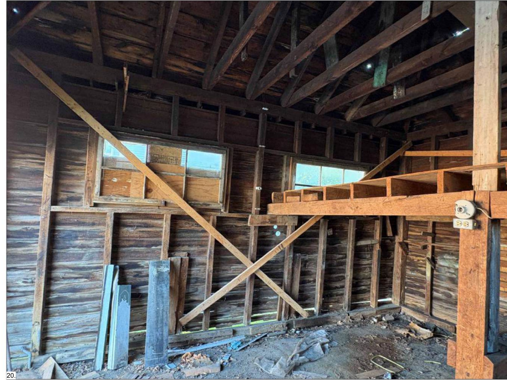
20. INTERIOR NORTH WALL
