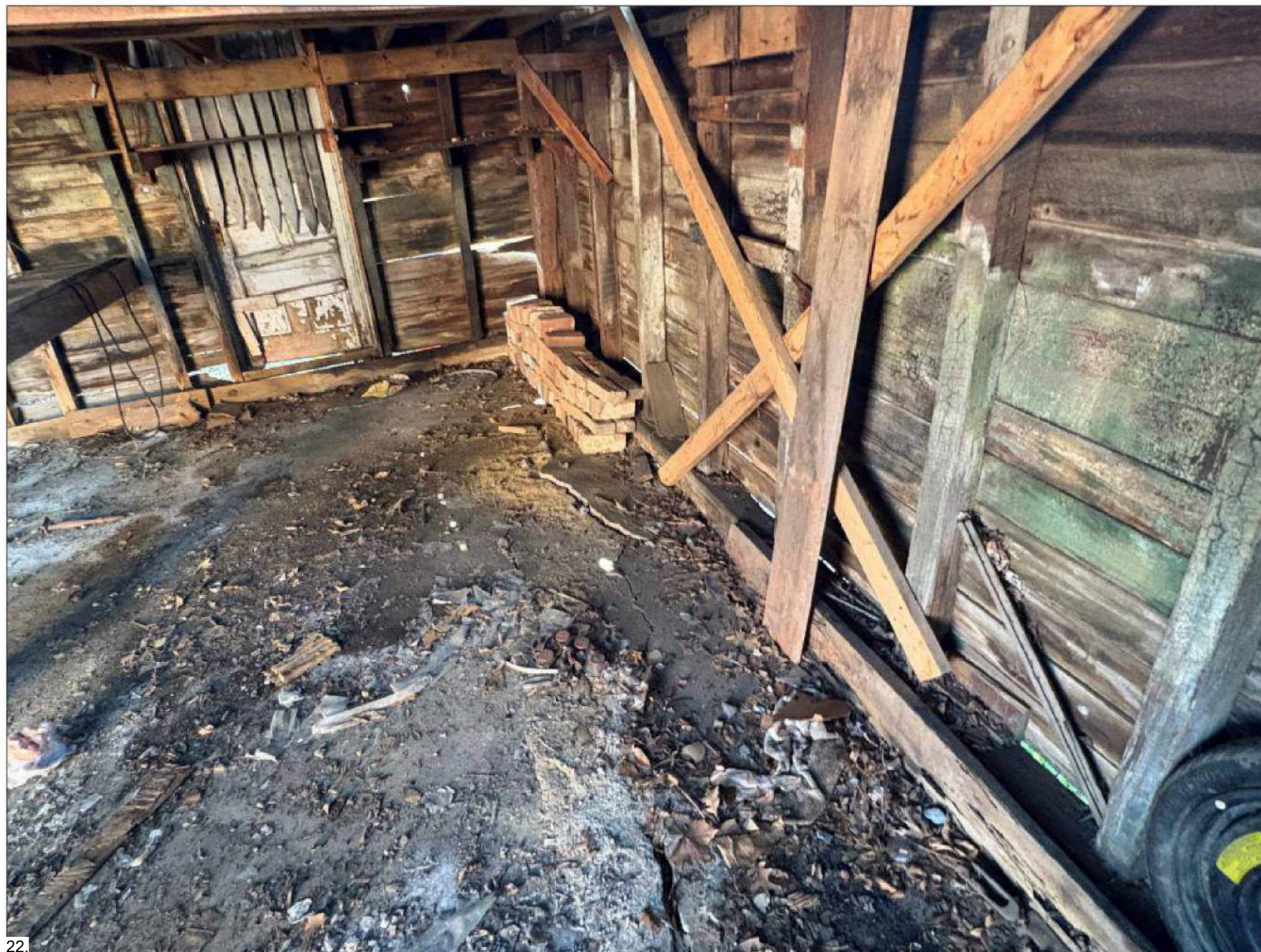
22. INTERIOR SOUTH WALL
