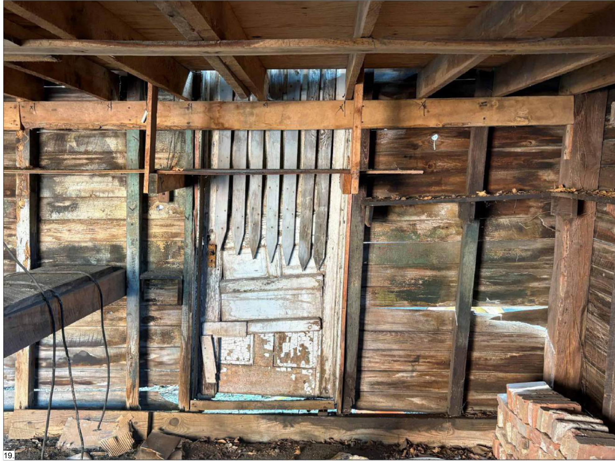
19. INTERIOR EAST WALL
