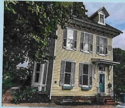
SWS storm windows protect Historic Windows while improving curb appeal.
