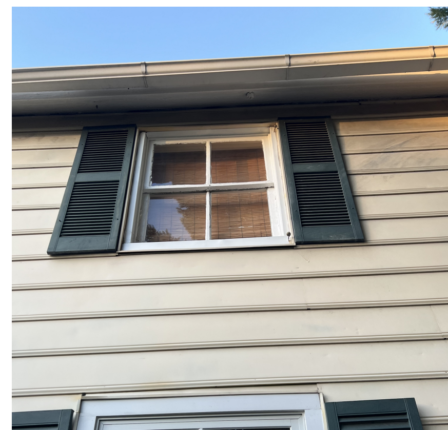
WOOD WINDOW WITH ALUMINUM TRIM VINYL SHUTTERS
