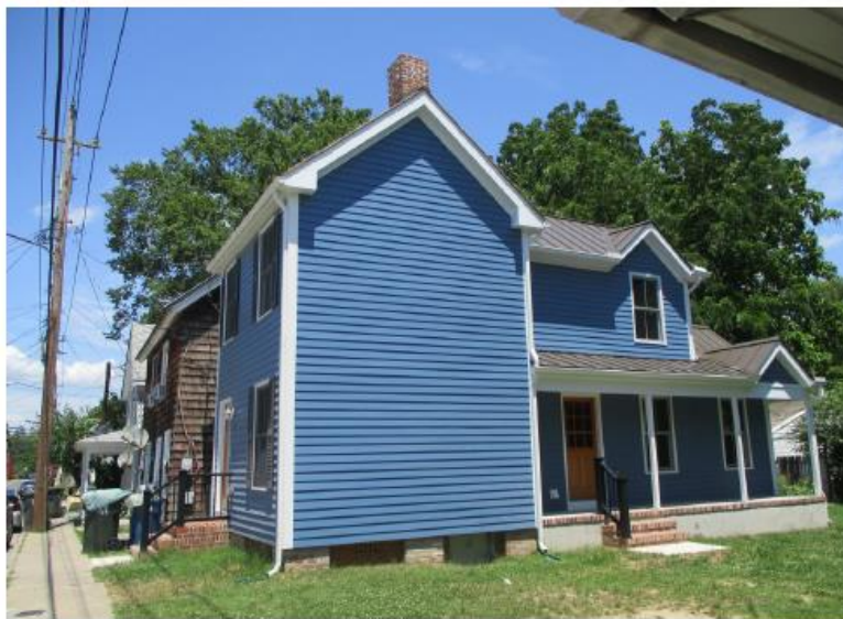
Figure 51: Many historic homes were constructed with rear or side porches. When visible from the public right-of-way, new porches should integrate with the setting.
