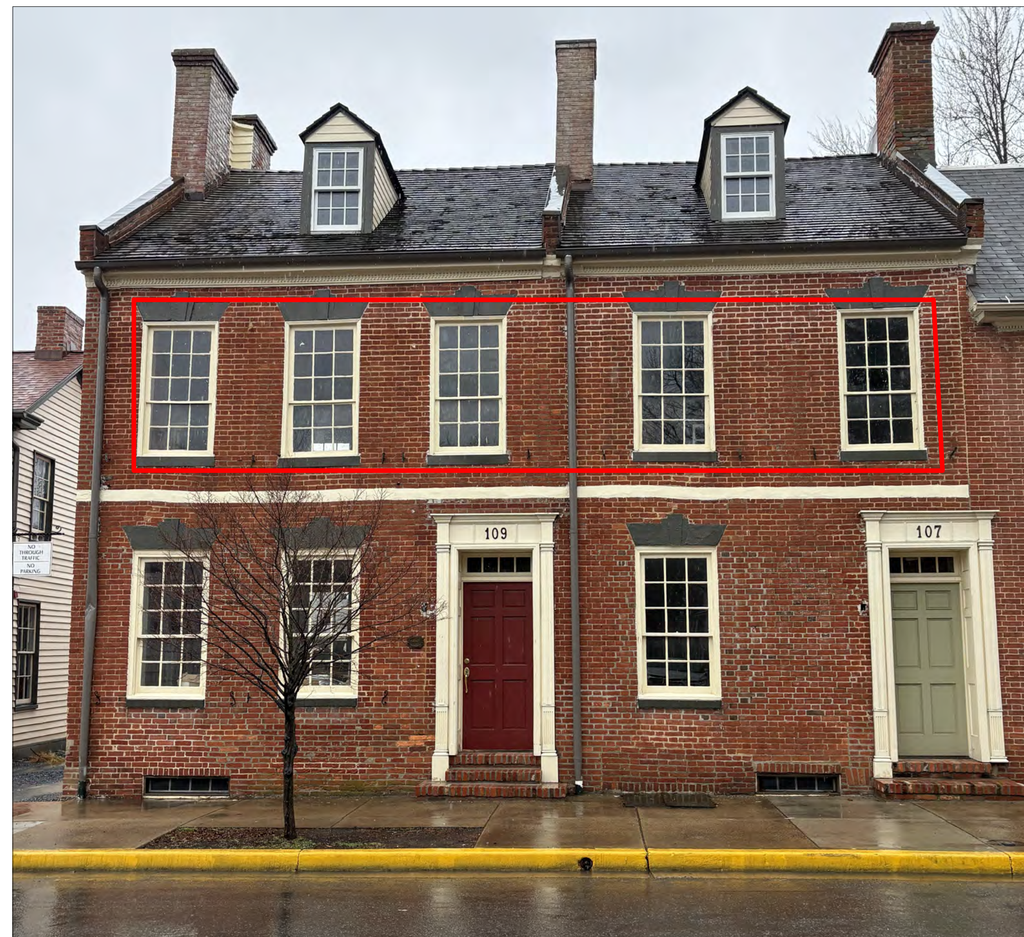
4 EAST FACADE EXISTING PHOTO HD2.1
