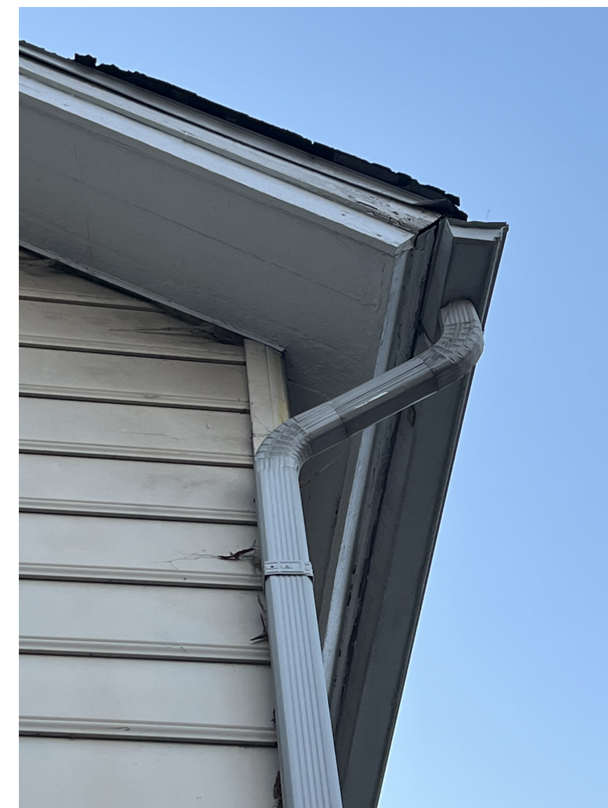
SIDING, SOFFIT, FASCIA GUTTER
