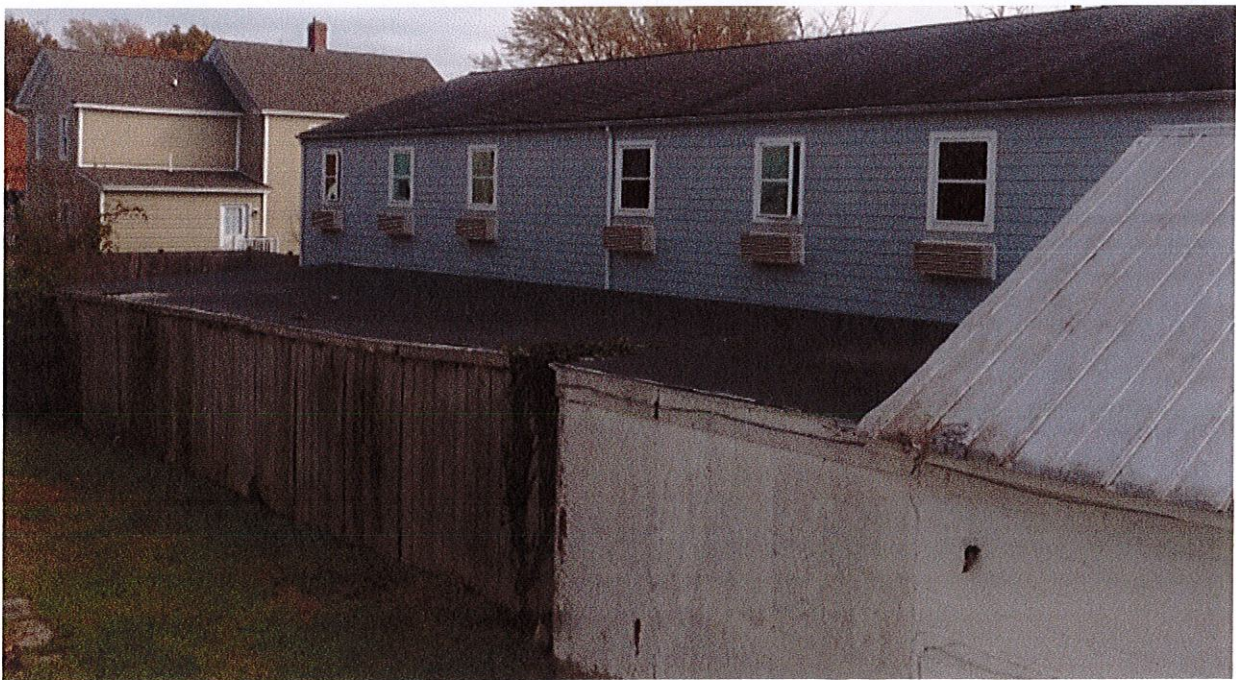
Roof – Original Structure to Remain
