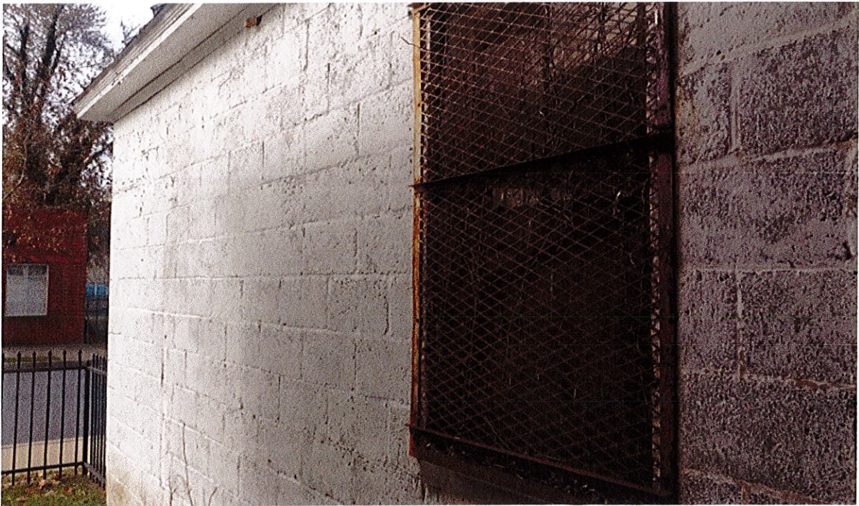
Southern Window Opening
