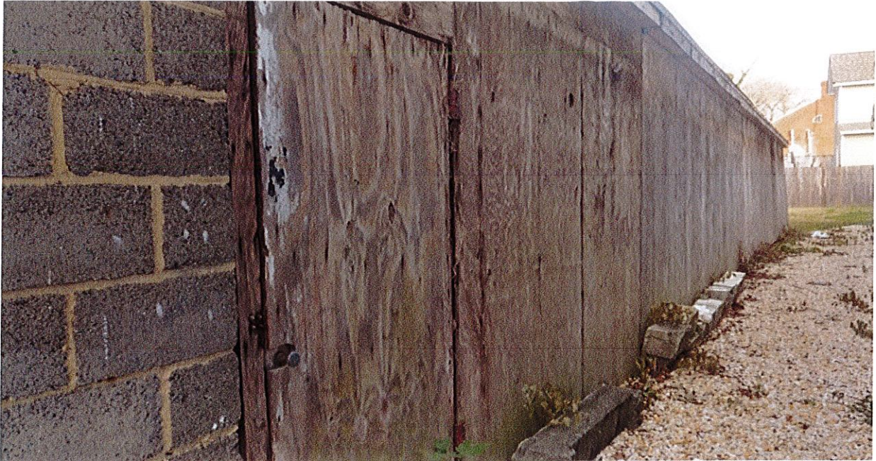
Southern Façade Looking East
