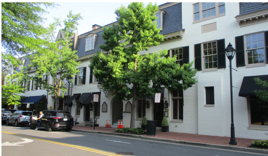
Figure 41: Chose a paint scheme that harmonizes with the environment and other building materials.
