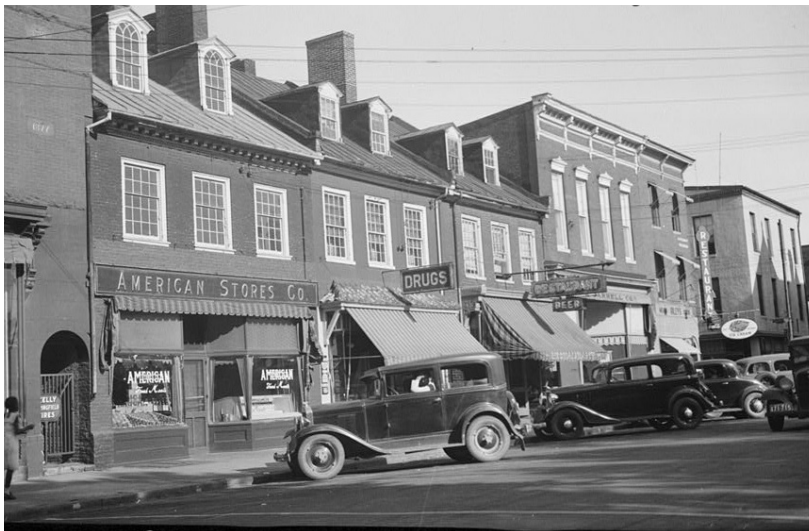
Figure 13: This view of Easton's commercial neighborhood on South Washington Street was taken in the 1930s.
