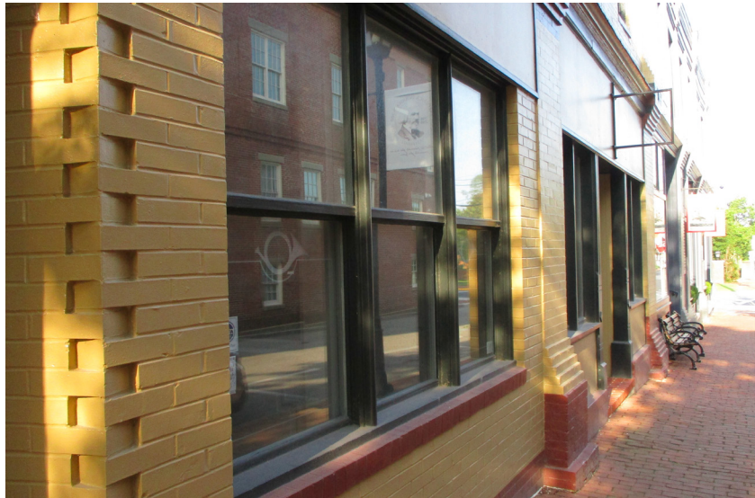
Figure 40: Some historic brick buildings were meant to be painted. Always use a masonry paint and never paint previously unpainted bricks.
