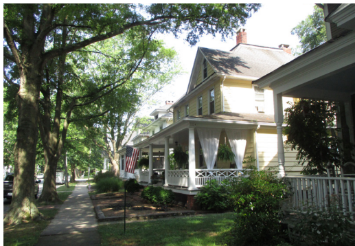
Figure 5: Historic homes often include sustainable features like operable transoms and porches that help to shade and cool the interior spaces.
