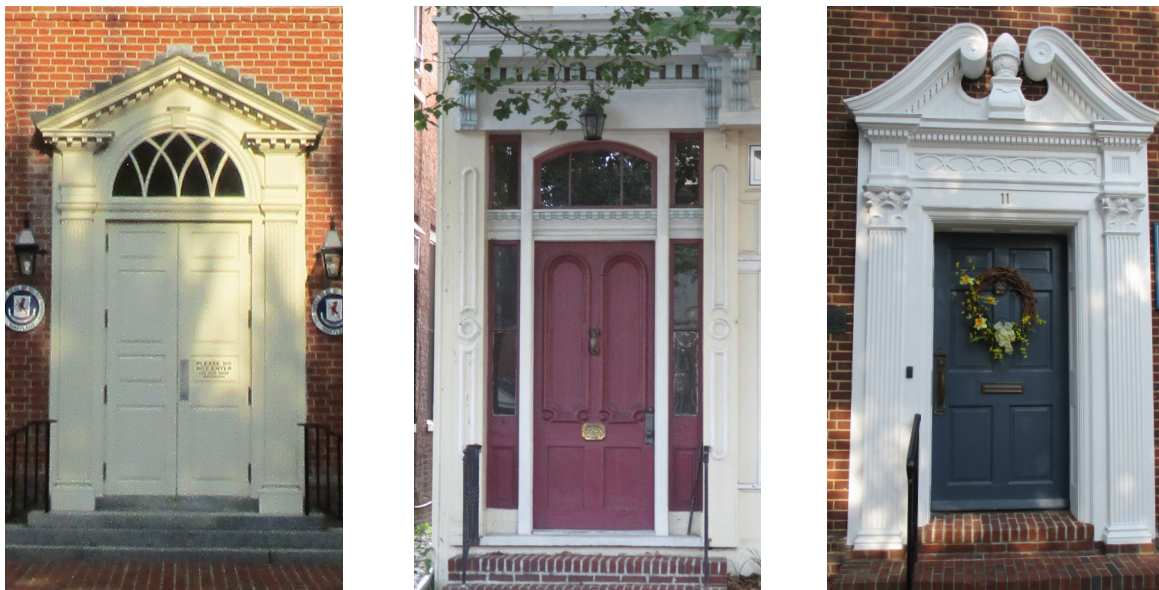
Figure 36: Doors are character-defining features that usually incorporate stylistic elements. From left to right: Federal, Italianate, and Colonial Revival.
