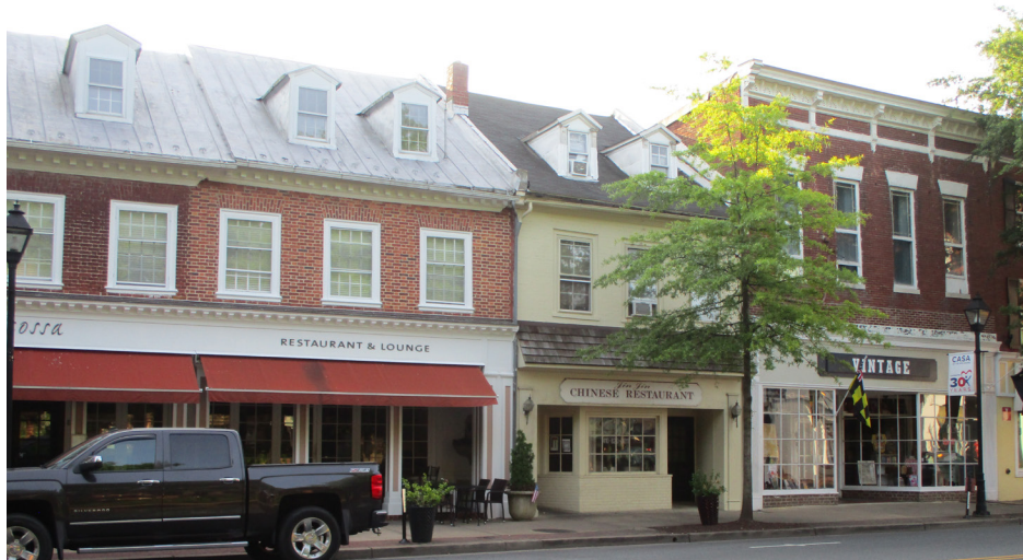
Figure 63: Most historic buildings designed for a commercial function included a signboard area.
