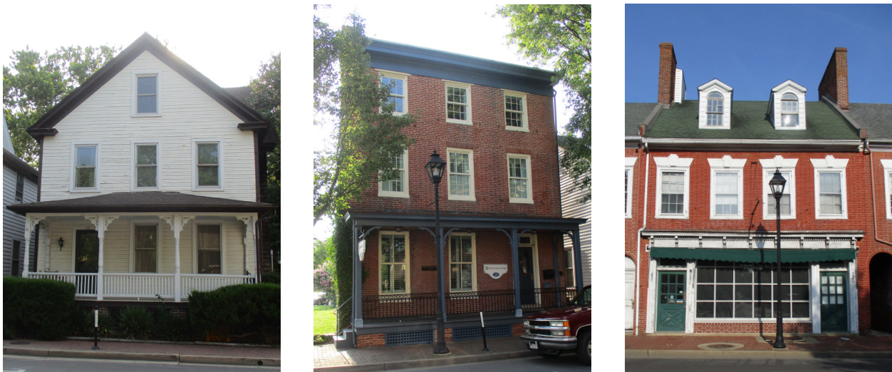
Figure 16: These examples of properties with high historic integrity have all retained their form, materials, and stylistic details.
