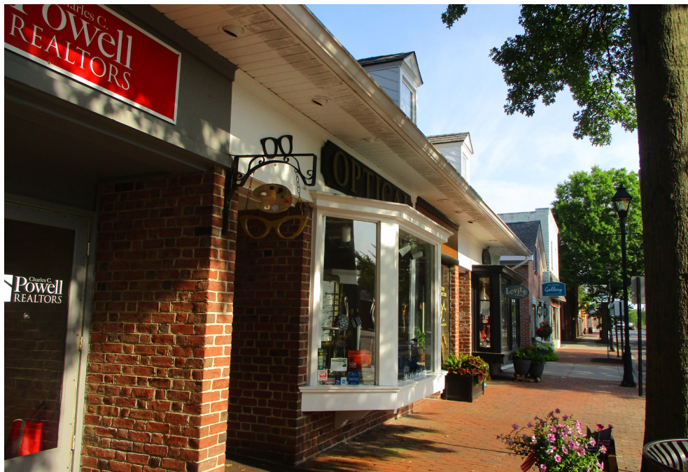
Figure 55: Many of Easton's commercial buildings have recessed entrances. New construction should maintain this street rhythm.
