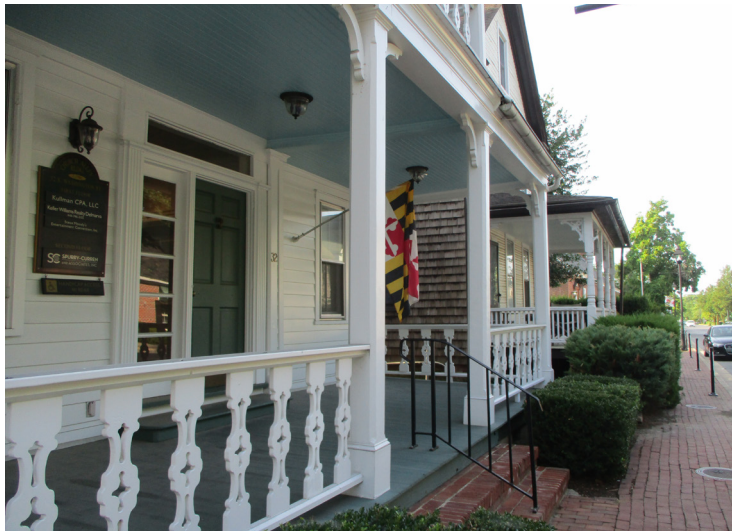
Figure 19: Historic features, like this porch railing, should be maintained or restored as needed.
