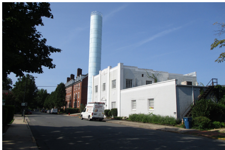
Figure 49: Locate utilities in inconspicuous places like rooftops and rear elevations.
