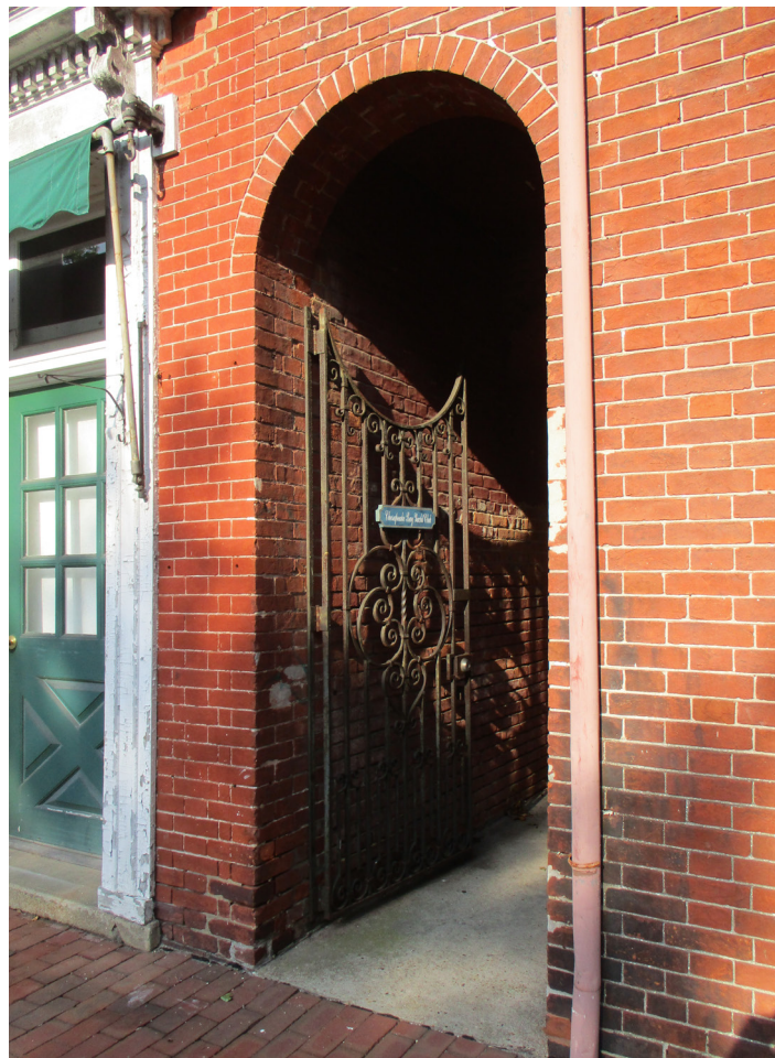
Figure 21: This historic grocer's alley still contains its original wrought iron gate.
