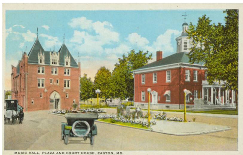
Figure 11: The Courthouse remains a focal point in Easton's historic district.
