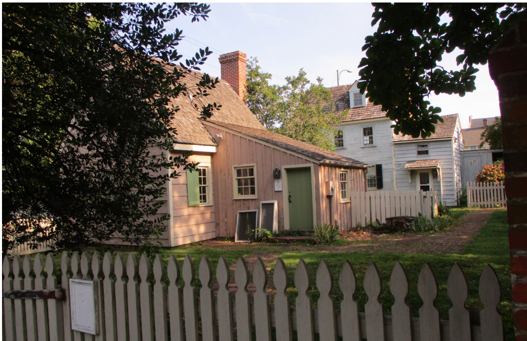
Figure 46: Wood siding was historically available in a number of profiles, widths, and configuration, including lapped siding and board and batten siding as shown on the buildings in the image above.
