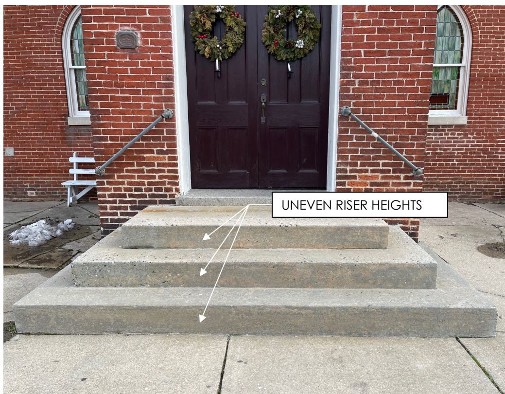
1. Front entry stair looking east.
