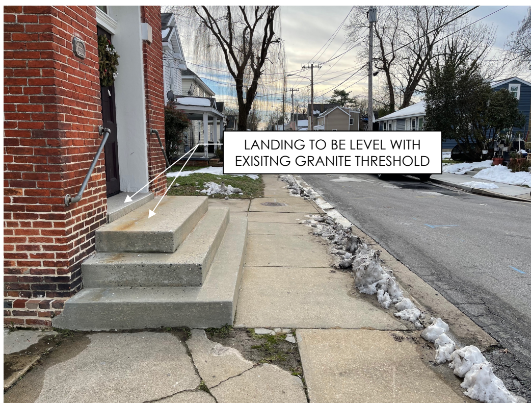
2. Cracked concrete pavement at north stair entry .
