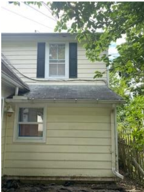
Potential location on lower rooftop for traditional air conditioning unit
