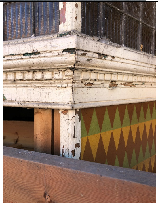
Existing Transom, storefront head & trims. (note glass will be clear not ptd)
