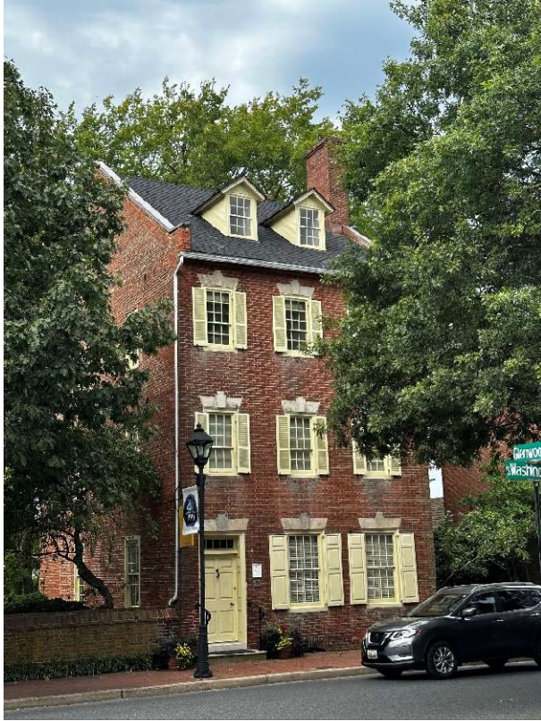
Figure 13: The James Neall House of the Talbot Historical Society with Architectural shingle roof.
