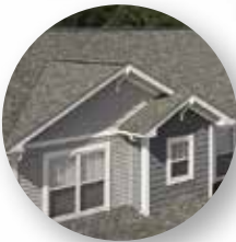
Roofing and Ventilation
