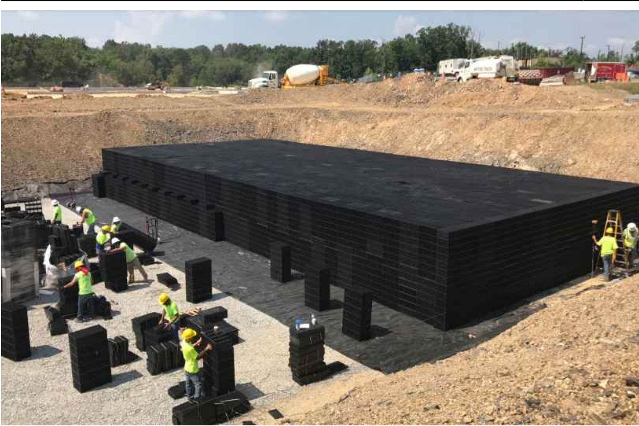
IMAGE: R-TANK STORMWATER MANGEMENT SUBSURFACE CHAMBERS BEING INSTALLED. PHOTO CREDIT: ACF INTERNATIONAL
