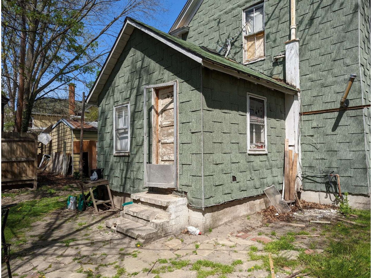
Picture 4: Existing condition rear. Roof over this existing first floor to be removed. Rebuild roof with Same pitch roof to increase interior ceiling height.
