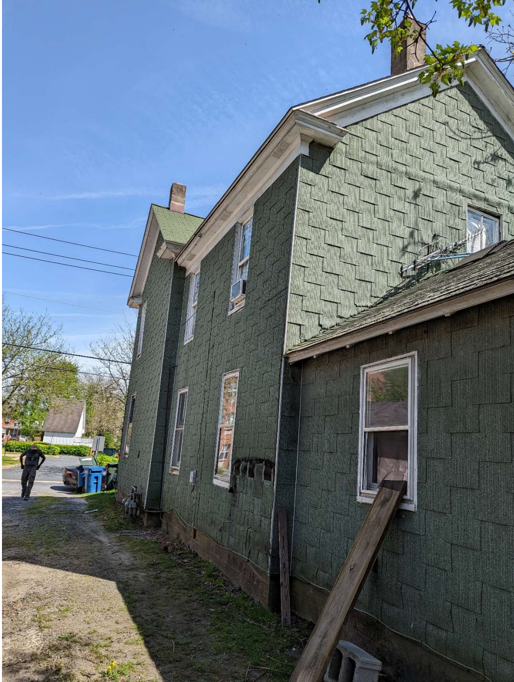
Picture 2: Existing condition right from rear
