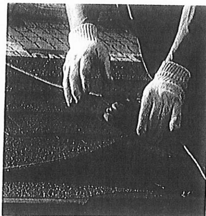
Installs at the eaves and rakes to help prevent shingle blow-off
