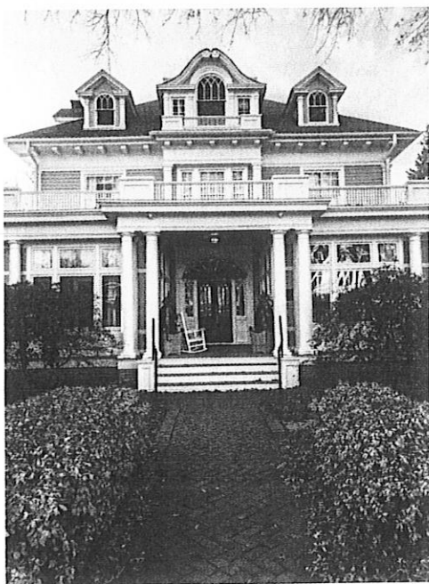
Figure 18: Tidewater Inn's Tidewater House with Architectural Shingle Roof.
