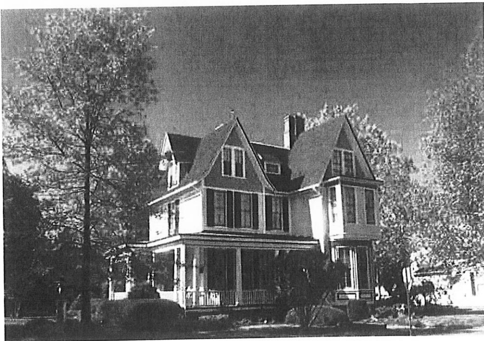
Figure 16: Bishop's House Bed and Breakfast with Architectural Shingle Roof.
