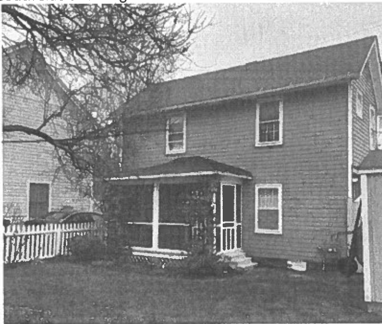
South side of cottage:
