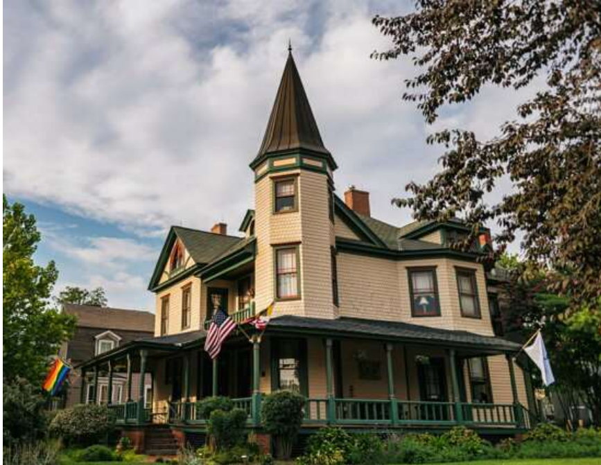
Figure 17: Hummingbird Inn with Architectural Shingle Roof.
