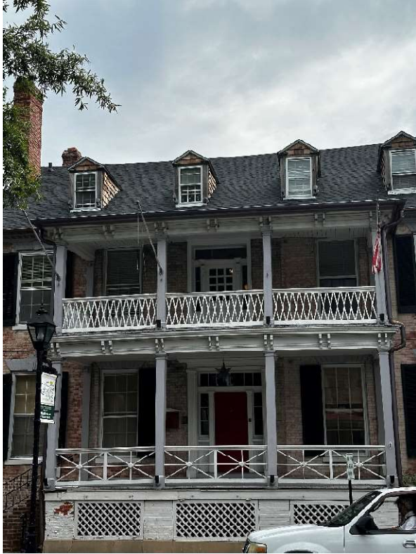
Figure 15: Bluepoint Hospitality's Bartlett Pear with Architectural Shingle Roof.
