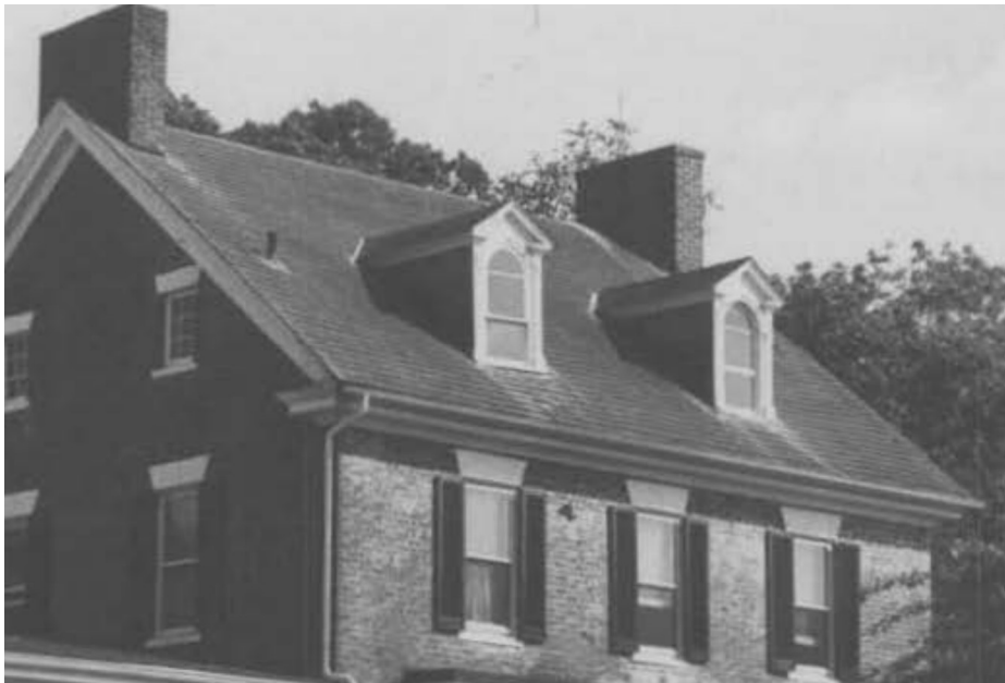
Figure 12: Image of the roof of our home from the Inventory Form For State Historic Sites Survey dated January 25, 1977.
