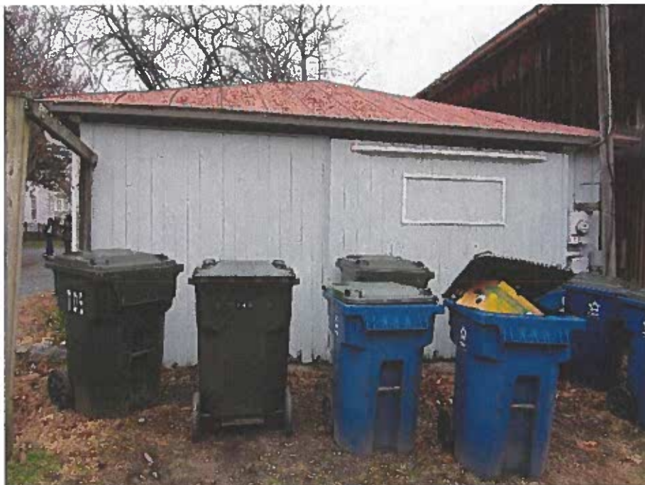
PHOTOGRAPH 22 East elevation of the one-story out-building.
