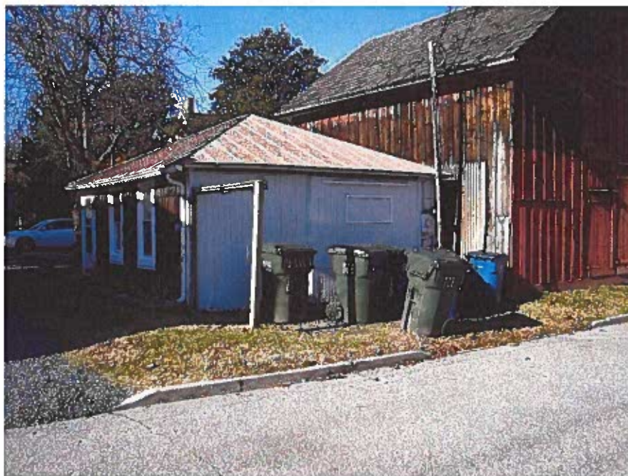
Alley view of the North outbuilding
