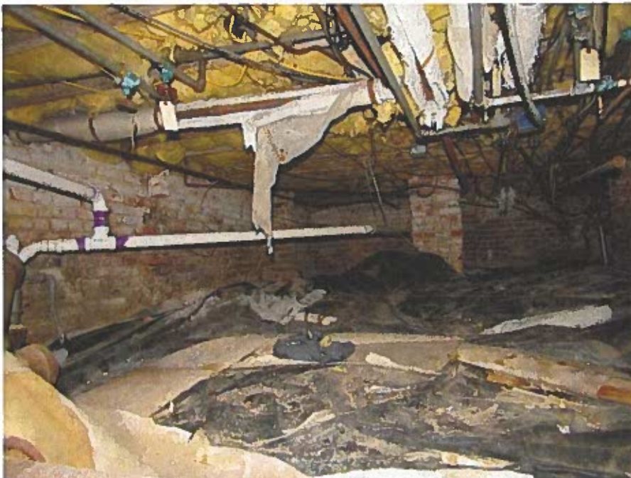
PHOTOGRAPH 6 Overview of the crawlspace at the east end of the main building.
