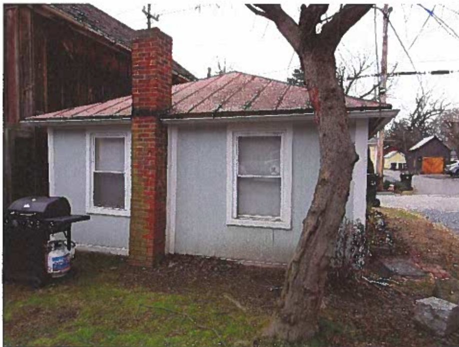
PHOTOGRAPH 20 West elevation of the one-story out-building.
