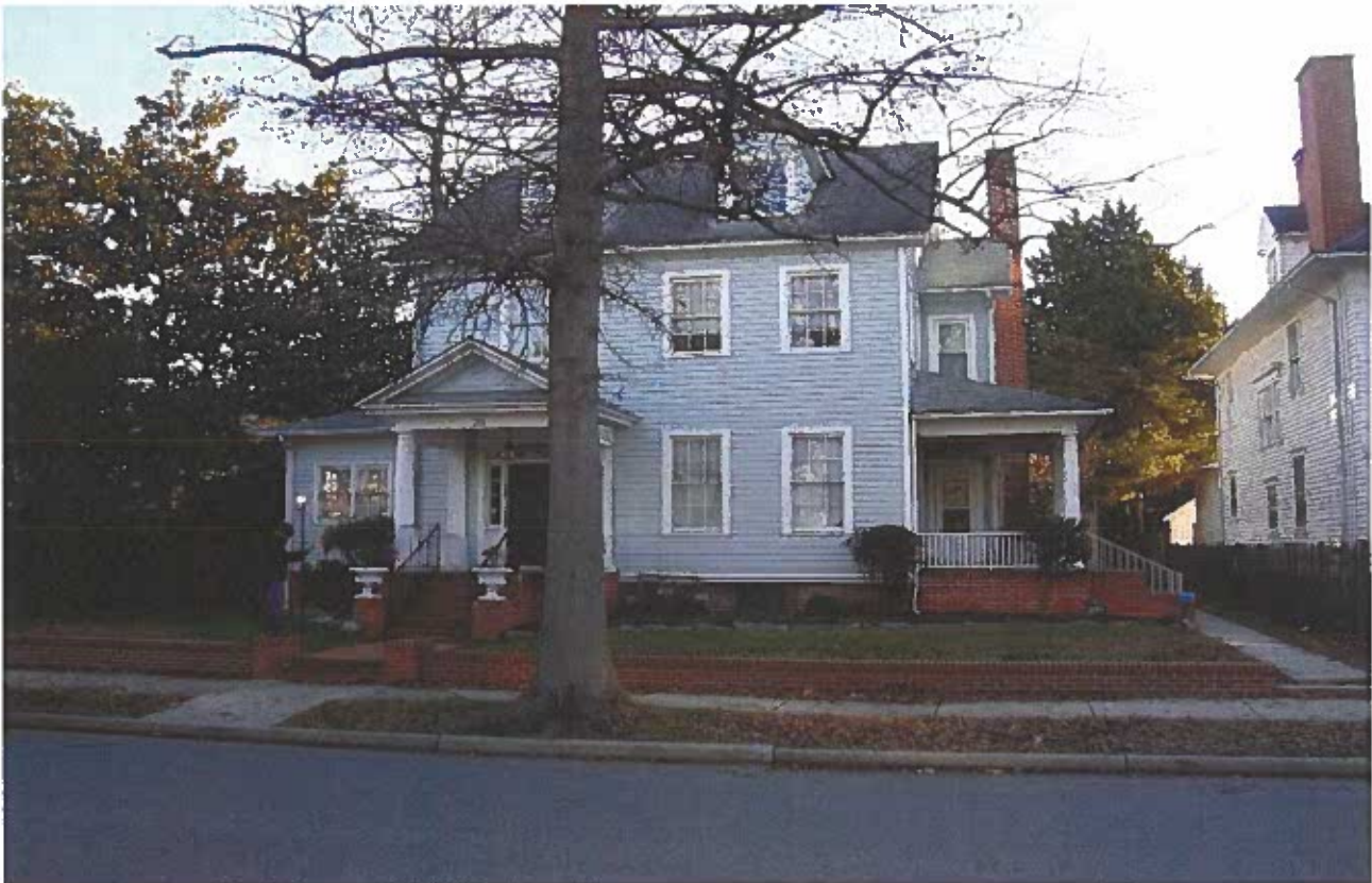
N. Aurora St. view of the main structure
