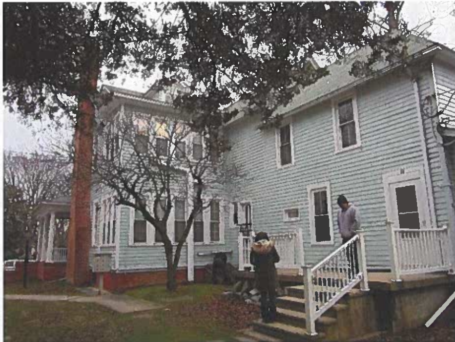
PHOTOGRAPH 5 South elevation of the main building.
