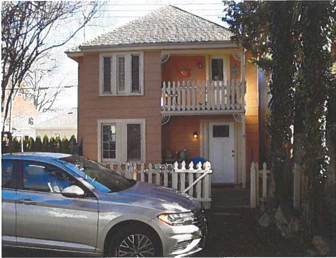
Front view of the South outbuilding
