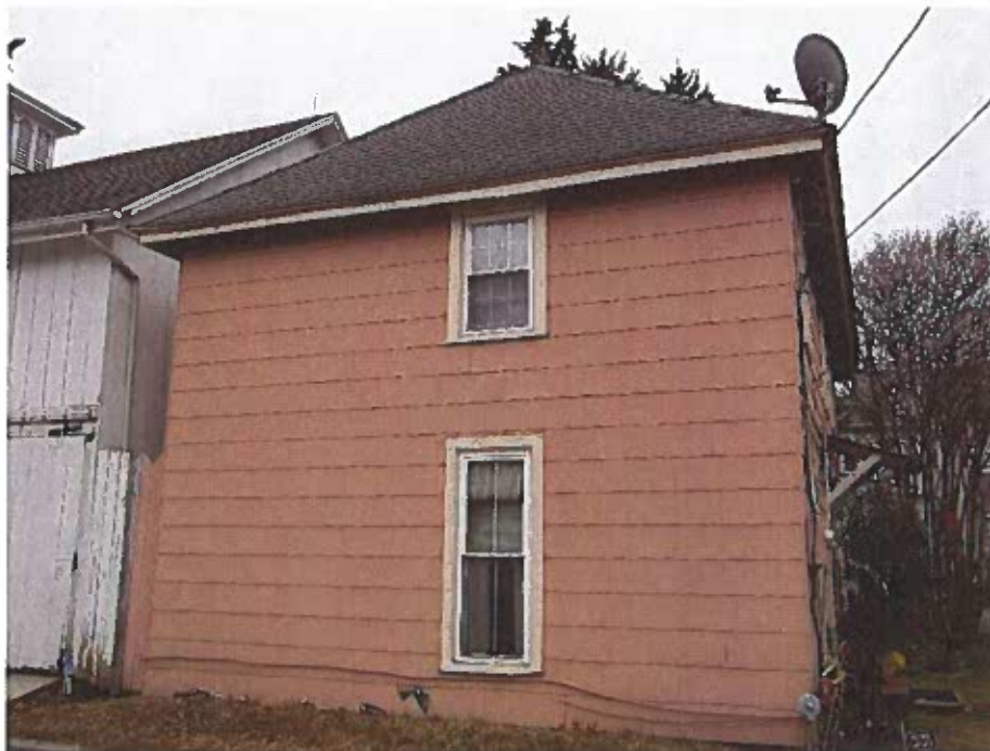
PHOTOGRAPH 15 East elevation of the two-story out-building.
