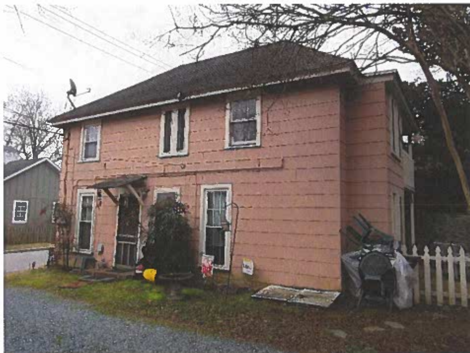
PHOTOGRAPH 14 North elevation of the two-story out-building.
