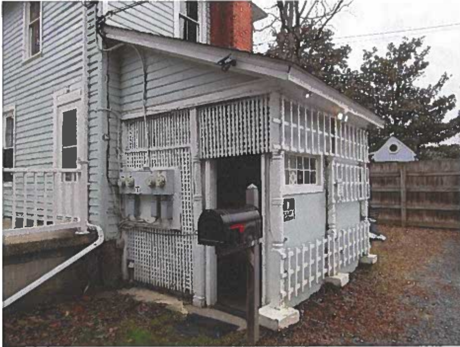
PHOTOGRAPH 9 East end of the main building.
