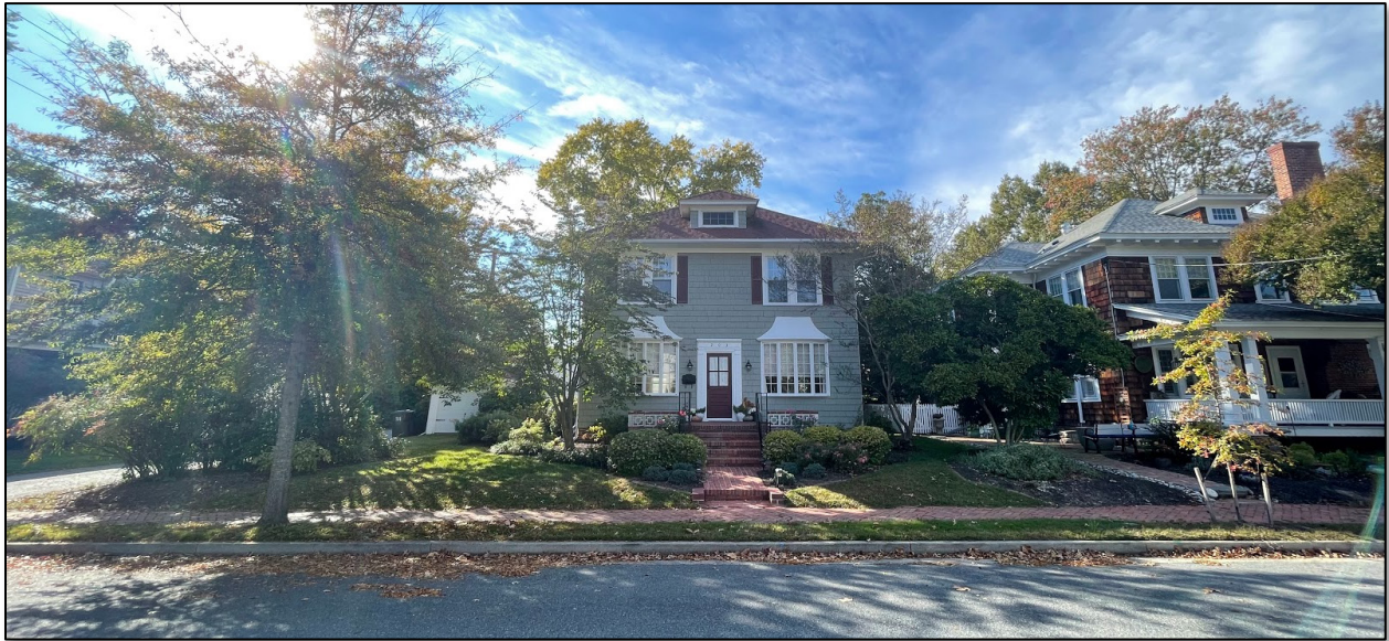
Front of house (view looking West from Hanson Street). Brook Lane is to the left (South), and 112 Brookletts Avenue property can be seen to the right (North).
