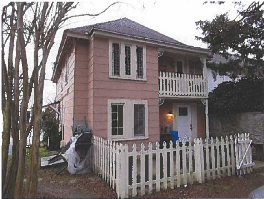
PHOTOGRAPH 13 West elevation (front) of the two-story out-building.
