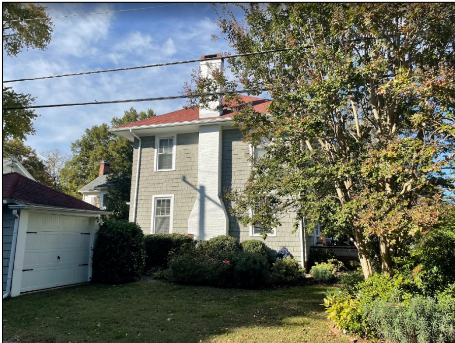
View looking North from Brook Lane (Hanson Street is to the right). This is the current main structure's South wall where two-story addition will be constructed. The new structure will not impact or contact current garage (at front left of picture).
