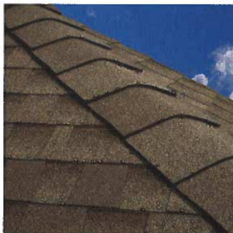
After A distinct finishing look that also protects against leaks and shingle blow-offs
